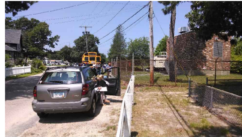
Fencing (3' board fence, 3' chain link fence, 6' security fence at pump station beyond)
