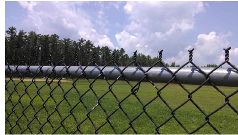
fence detail at top rail (note exposed barbs)
