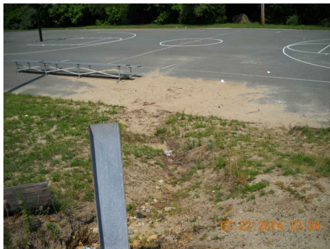
Erosion (at southwest corner of courts)
