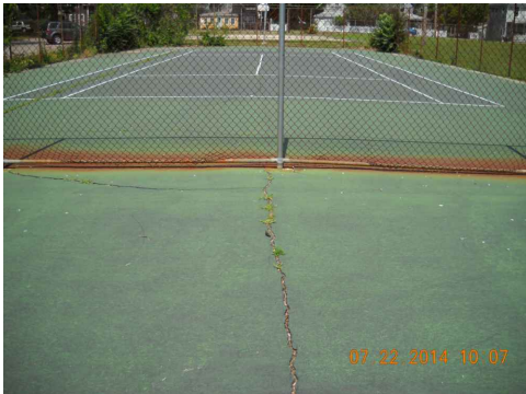
Court Surface (cracks and rust stains visible)
