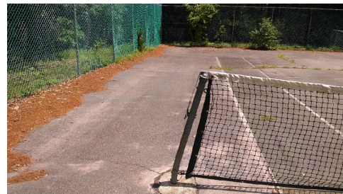
Tennis Net (damaged net post, surface cracking visible)
