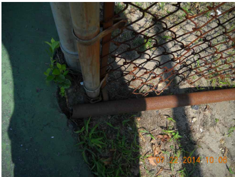
Gate hinge (damaged)
