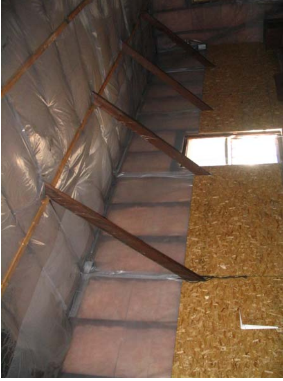
#30) 2x diagonal uplift tie to secure truss to wall. (Packaging)
