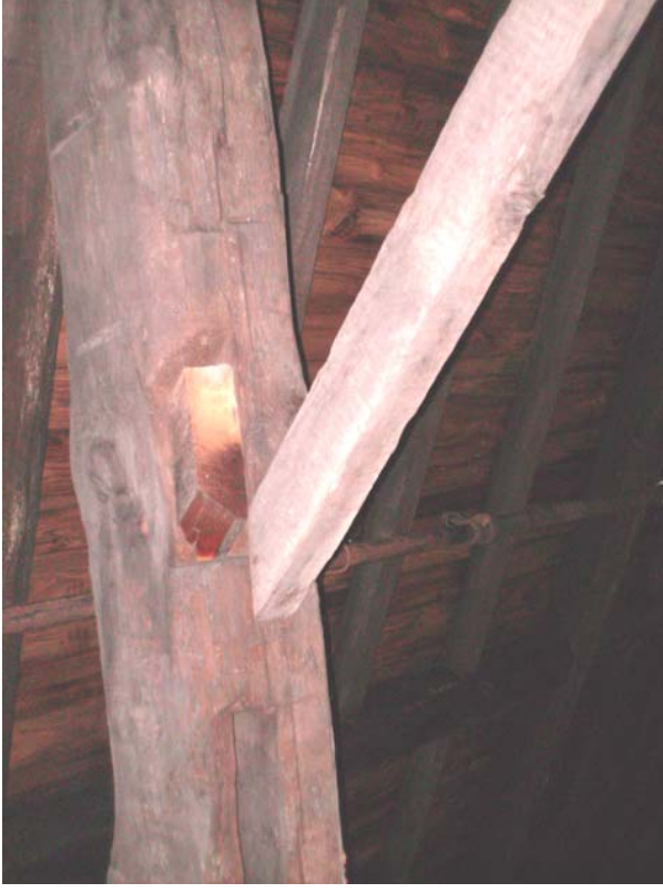
#42) Truss diagonal bracing cut-out and replaced, new bracing is smaller and toe nailed to truss. (Freight "A")
