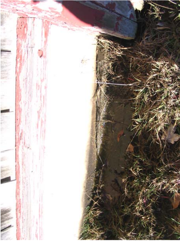
#29) Standing water located next to CMU foundation wall. A water management system should be implemented at this site. (Packaging)
