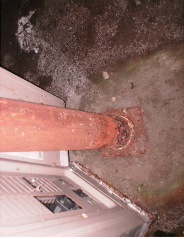
#10) Steel lolly column not secured to the foundation and has significant surface rust. The column should be replaced and mechanically fastened to a proper foundation. (Office "A")
