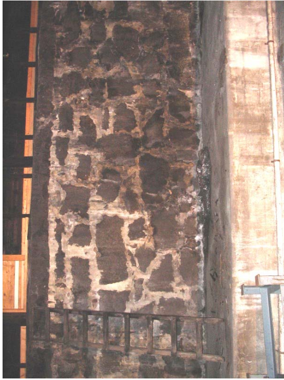
#80) Stone rubble foundation wall with concrete slab inset, and wood frame wall on top. (Factory "C")
