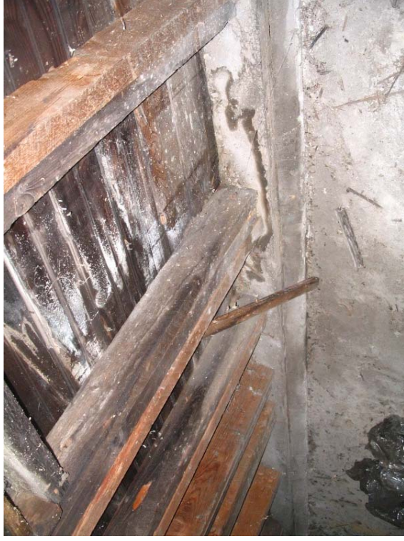
#81) Water staining and minor deterioration of sill and stud wall on low grade side. (Factory "C")
