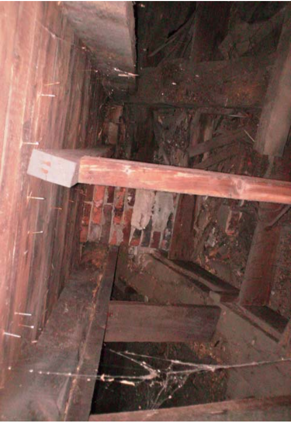
#3) An additional 2x rafter placed next to the chimney and supported with a post bearing on the ceiling joist (Office "A")
