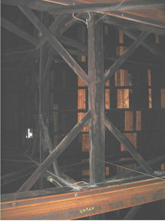
#94) Bottom chord bracing of truss, center bracing of truss (Typical) (Factory "D")
