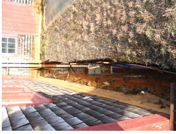
#63) Wooden foot bridge has deteriorated to the point where it should be removed or replaced. Note that one of the railings has fallen off. (Factory "ALL")
