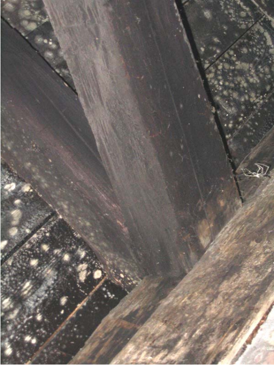
#70) Timber wall tie and roof rafter connecting to sill. (Factory "A")
