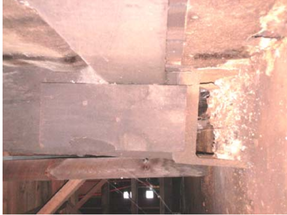
#104) Questionable support of post allows the southeast side of the building proper post base and connection shall be provided. (Factory "D")
