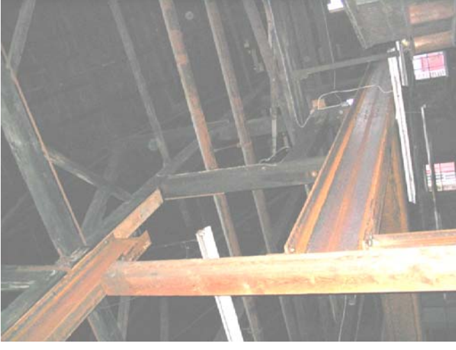
#91) Steel beams supporting the truss bottom chord and the original posts under the trusses (Factory "D")
