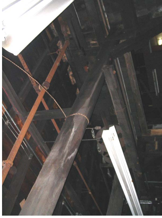
#77) Post and beam which supports the roof beam at the mid span of the rafters. (Factory "B")
