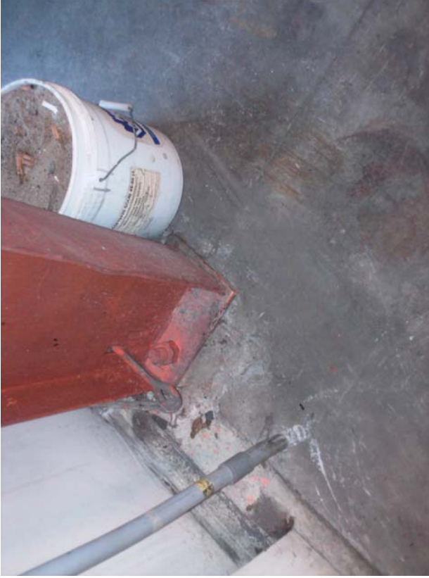
#17) Column bearing on pilaster and slab-on-grade with no leveling grout. Monitoring of pilasters should be implemented and grout placed under the columns. Also note that the cross bracing cable has been cut. (Steel Bldg.)
