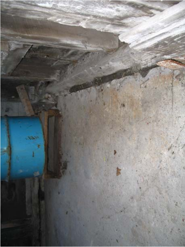
#25) Rotation of the sill due to deterioration (Pickling)
