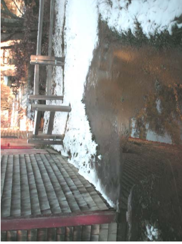
#55) Ice and water build-up against the sill. Site water management should be planned to shed water away from all buildings. (Freight "A")
