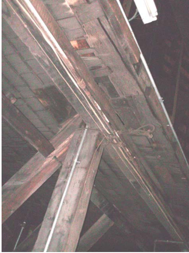
#47) The Timber frame roof support bearing on the bottom chord of the gable end truss of the original building. (Freight "B")
