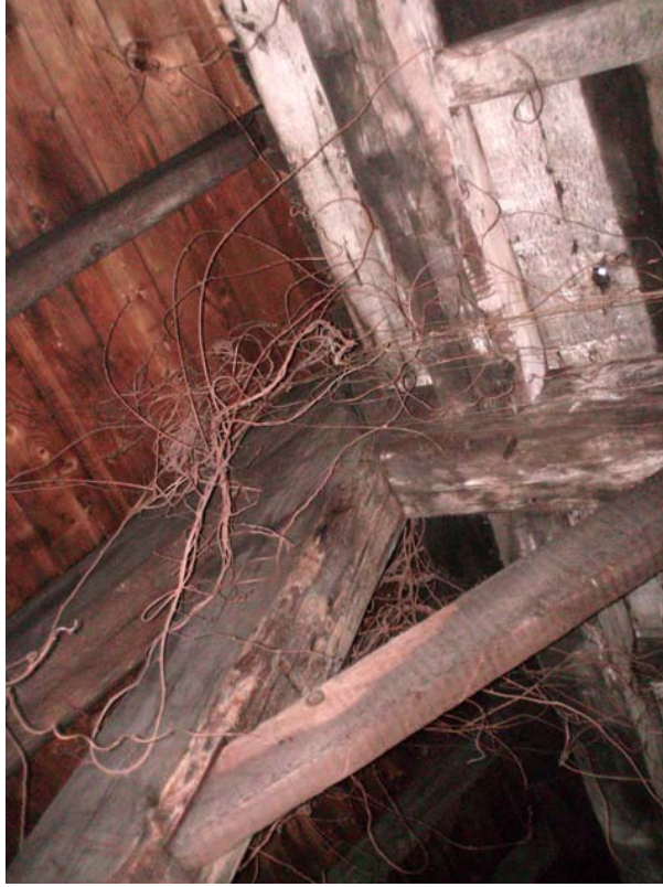
#41) Post under truss has been replaced. (Note the shim between the post and truss.) This post should be replaced with a properly sized full height post. (Freight "A")
