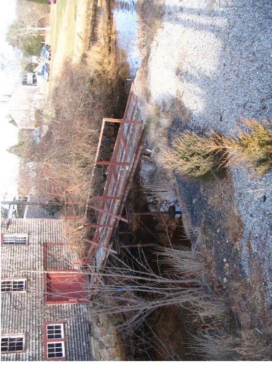
#63) Wooden foot bridge has deteriorated to the point where it should be removed or replaced. Note that one of the railings has fallen off. (Factory "ALL")
