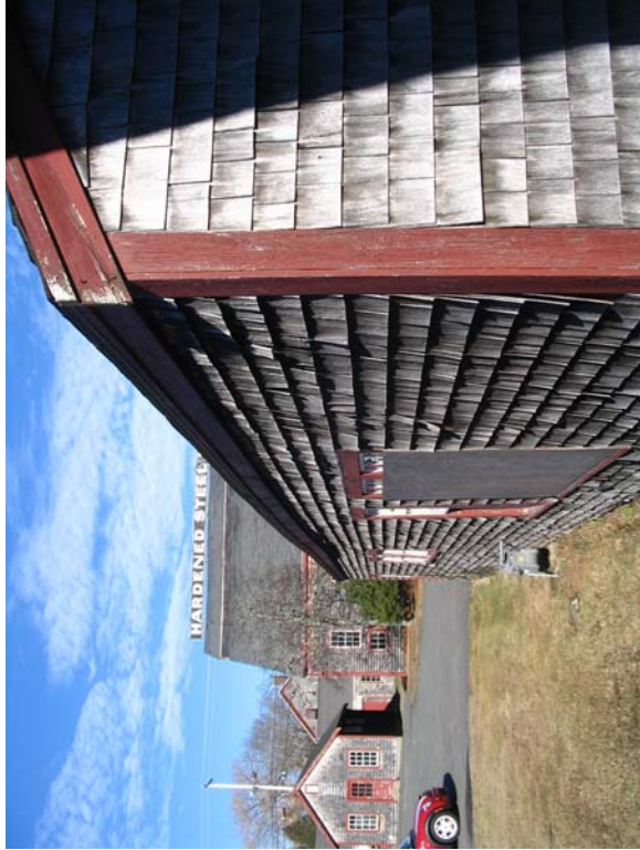
#23) Bow in wall at top plate due to the roof loading and inadequate roof tie system. (Pickling)
