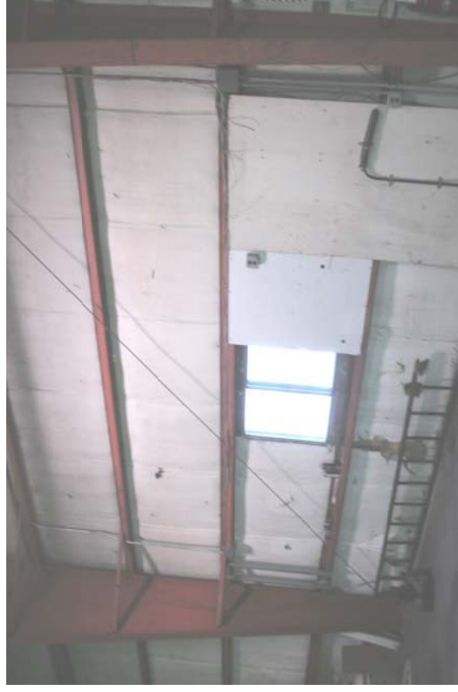
#20) Cross bracing in one direction is missing and should be replaced immediately . (Steel Bldg.)
