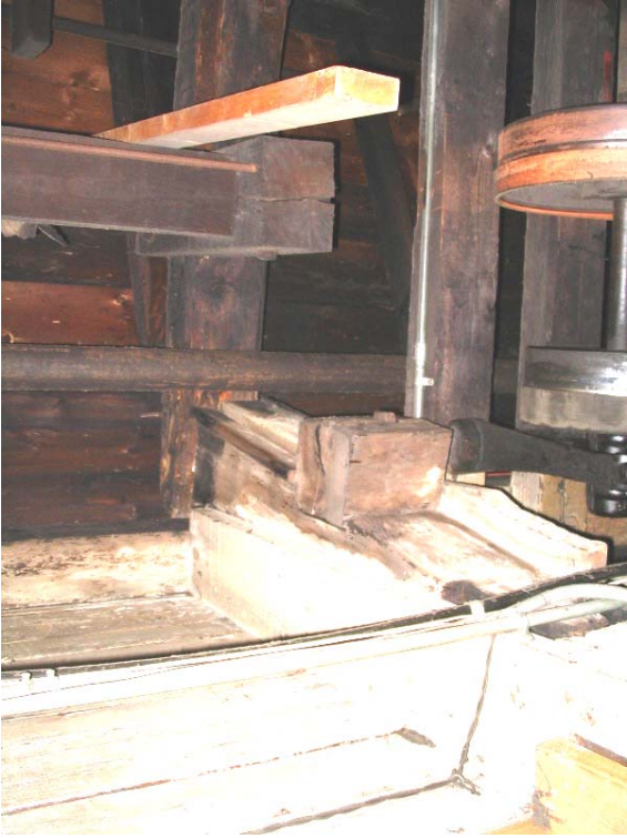
#74) Post support under wood truss, typical throughout (Factory "B")
