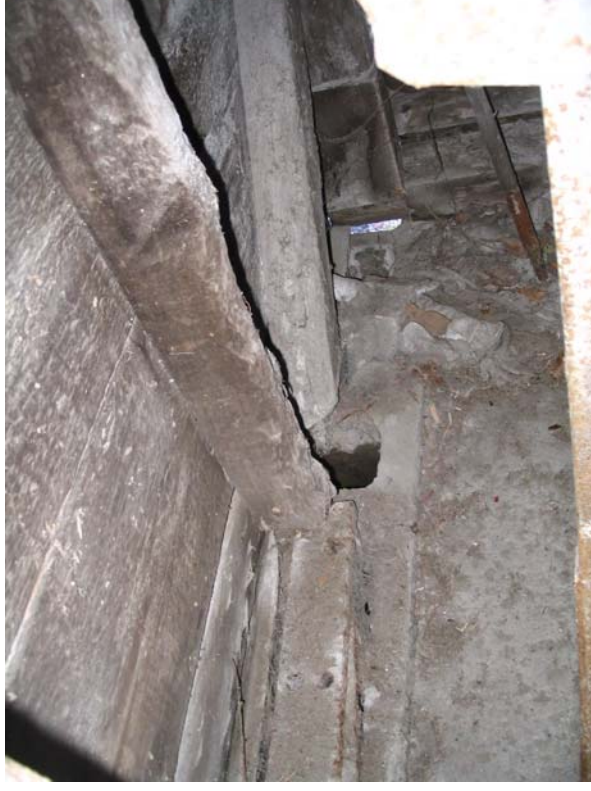
#24) Considerable deterioration of the sill. The sill should be replaced if the building is to be saved. (Pickling)
