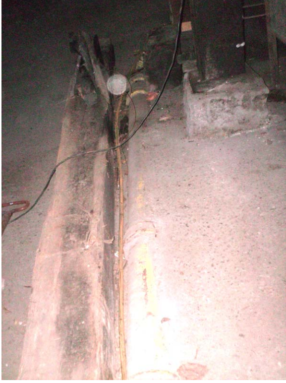
#97 Main exit pipe for culvert. Note that pipe is sloped and disappears under the slab. (Factory D")
