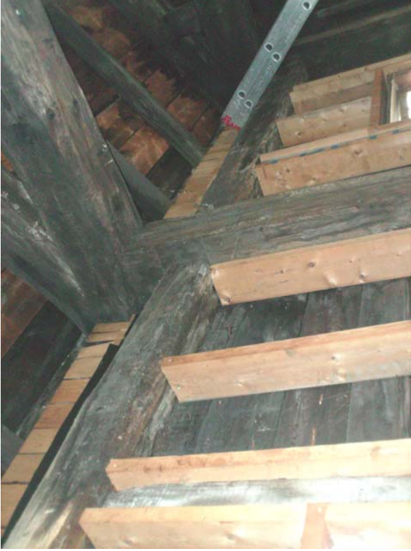
#45) Top wall plate below truss, note the 2x6 stud infill wall between the posts. (Freight "A")
