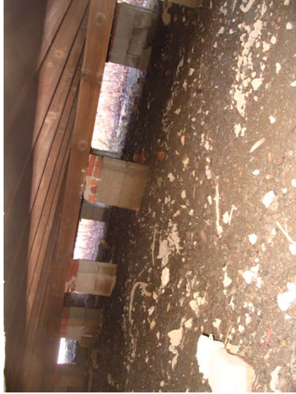
#35) Clay brick infilled between CMU and foundation. (Note: no connection of shed to pier.) (Shed)
