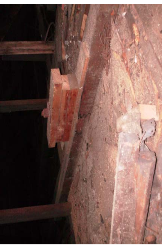
#2) Typical post support for the roof hip beam (Note the debris in the attic, which should be removed.) (Office "A")
