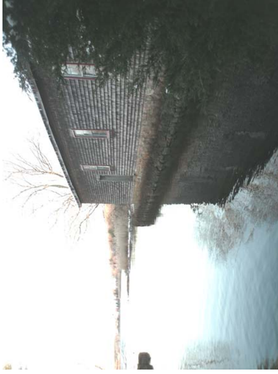
#51) The chimney for the wood burning stove needs to be repointed at the upper third. The bottom appears to be in good condition. (Freight "B")
