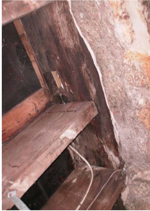
#11) Floor joist mortise and tenon into sill. Properly sized joist hangers to secure joists to sill should be used. (Office "A")
