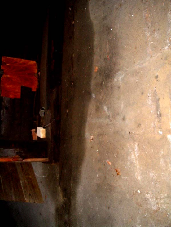
#75) Deterioration of sill between additions in area "B." This sill should be replaced with a new pressure treated sill fastened to the foundation. (Factory "B")
