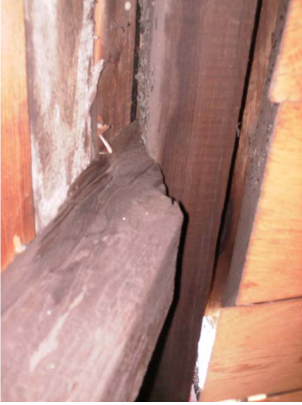
#46) The rafters bear on a 3"x5" beam spanning between trusses and provide limited bearing area for the rafters. (Freight "A")
