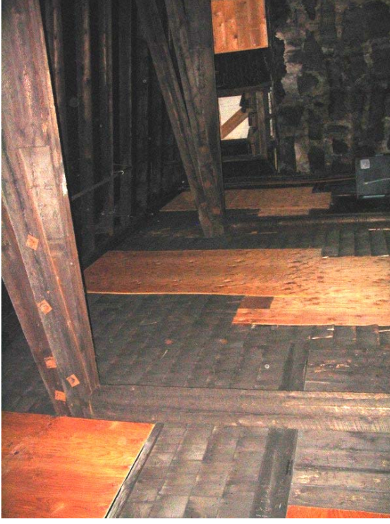
#79) Support of semi-truss on post at the original exterior wall. (Factory "C")
