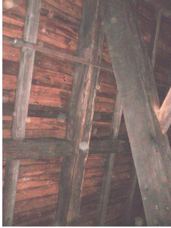
#40) Typical rafter and purlin Rafter system rafters are mortis and tenon together (Freight "A")
