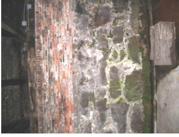
#69) Foundation Wall at high grade, 5'-7" stone rubble, 5" cement, 2'-1" clay masonry. (Factory "A")
