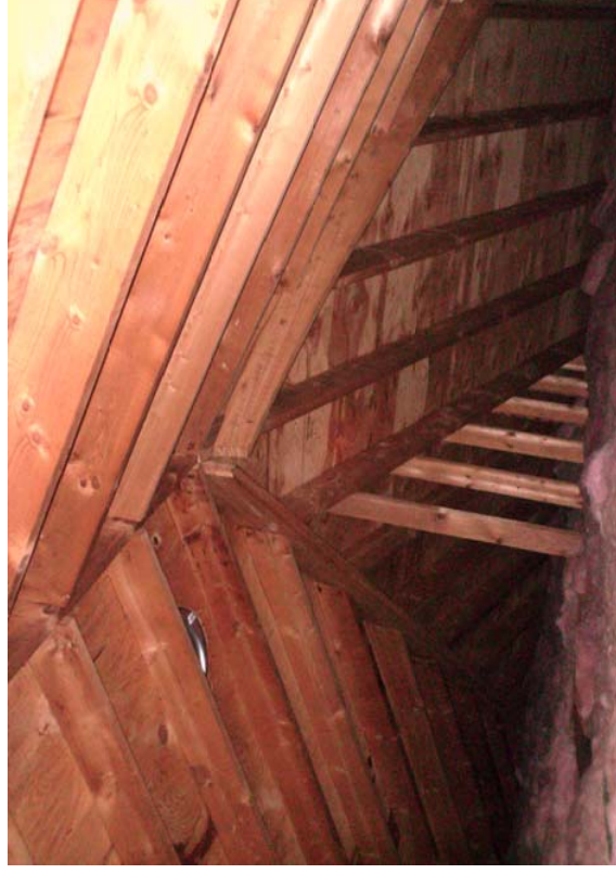
#12) Hip roof framing, using a hip board design and plywood roof sheathing. (Office "B")
