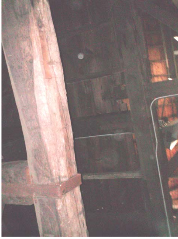
#44) Metal connector used to connect the king post to the bottom chord. (Freight "A")
