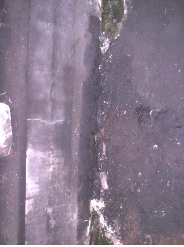
#103) Minor cracking noted in the concrete foundation wall along the low grade side of the factory (Factory "D")
