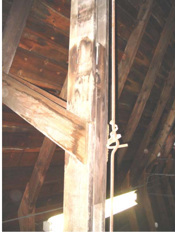
#27) Connection of steel tie elements (Note if tension seizes the ties would sag.) (Pickling)
