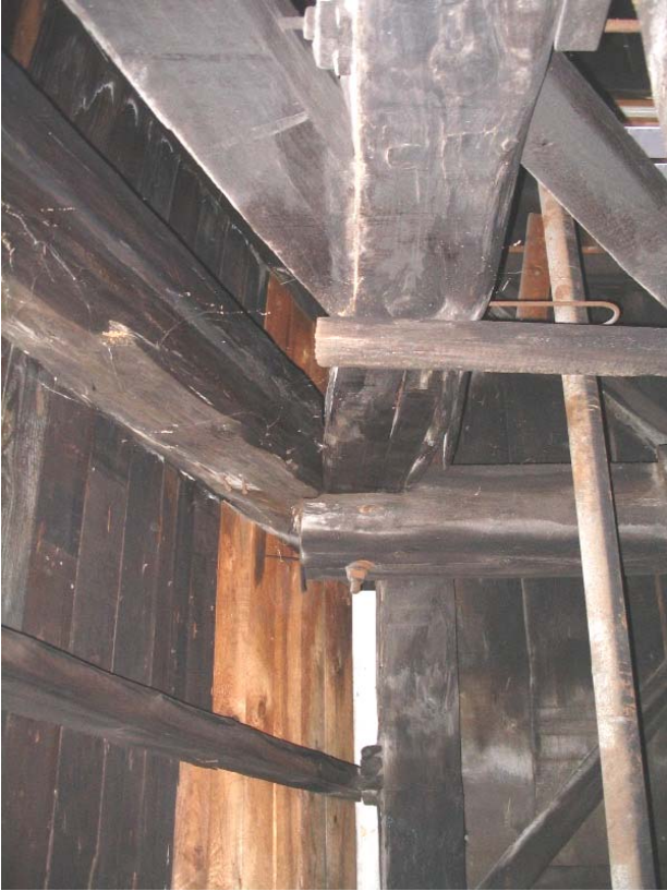
#86) Truss connection to end post. Note the shear failure of the truss at the support. (Factory "D")
