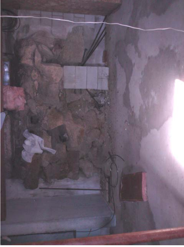
#14) Stone foundation from the original building protruding into the new building foundation. (Office "B")
