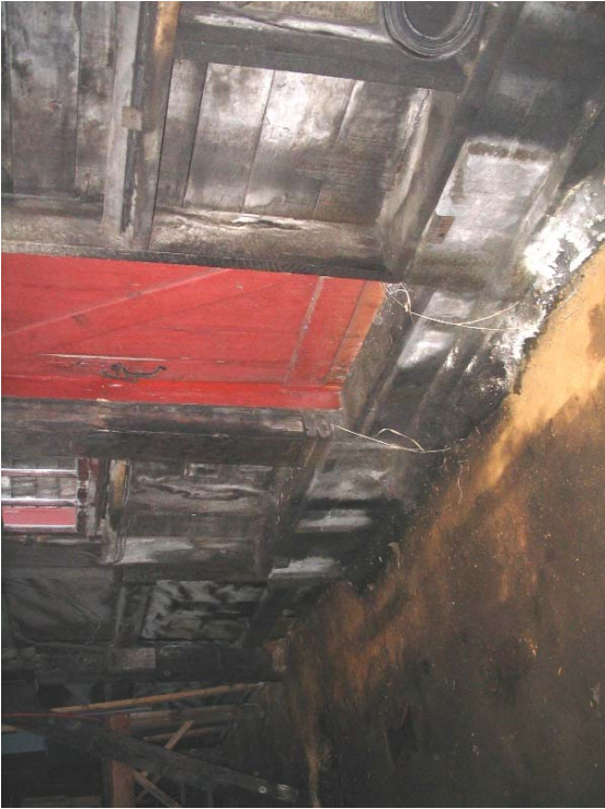
#90) 2x6 stud in fill wall with no connection of the sill to the concrete foundation wall. (Factory "D")
