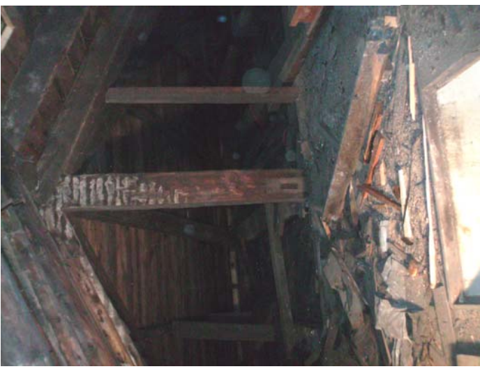
#2) Typical post support for the roof hip beam (Note the debris in the attic, which should be removed.) (Office "A")
