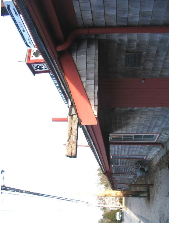
#59) Timber beam supporting roof; Note that the front wall leans in at the end. (Factory "D")
