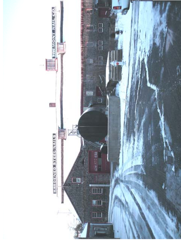
#56) Overview of the rear of the factory building. Note that the lines on the roof are the truss location. (Factory "ALL")
