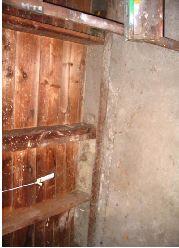
#31) Stud attached to sill w/steel angle. Sill appears to be in good condition w/little deterioration. (Packaging)
