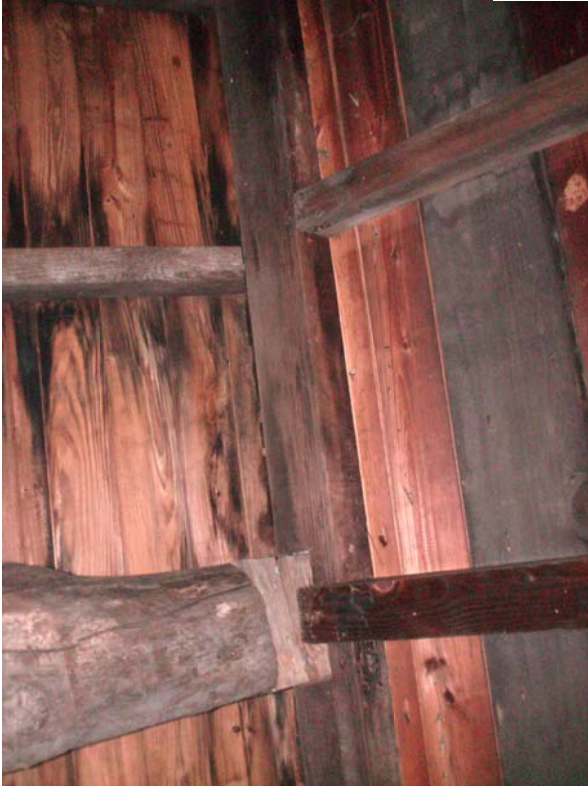
#41) Post under truss has been replaced. (Note the shim between the post and truss.) This post should be replaced with a properly sized full height post. (Freight "A")
