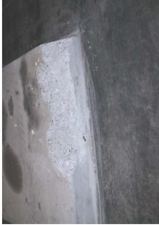
#17) Column bearing on pilaster and slab-on-grade with no leveling grout. Monitoring of pilasters should be implemented and grout placed under the columns. Also note that the cross bracing cable has been cut. (Steel Bldg.)
