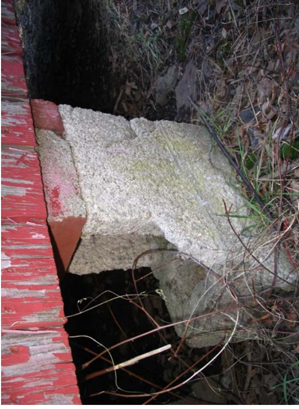
#34) Broken CMU support, Note that the CMU is not reinforced or grouted. The foundation should be replaced with steel reinforced sonotubes and "Bigfoot" footings. (Shed)
