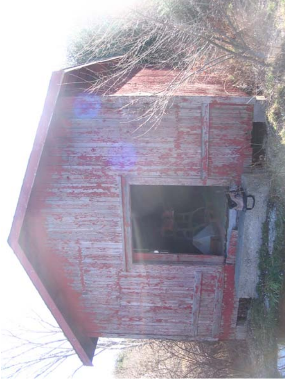
#33) Front view of shed, note that the siding is in poor condition and the exposed ends of the floor boards are deteriorated. (Shed)
