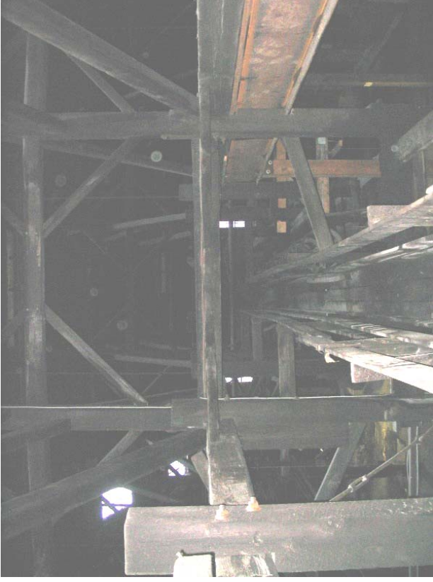
#87) Lateral cross bracing of the truss (typical) (Factory "D")
