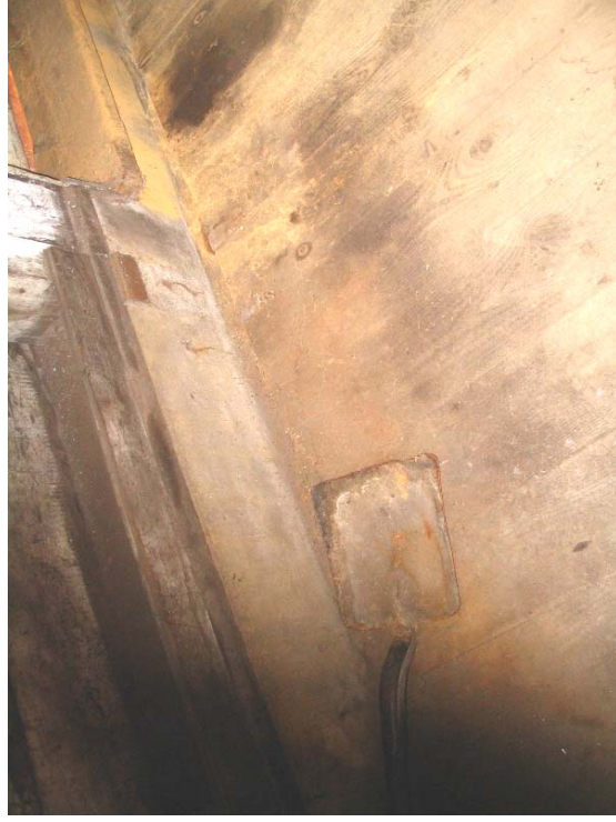
#73) 2x sill bearing atop concrete foundation wall with no fastening to the foundation observed. (Factory "B")
