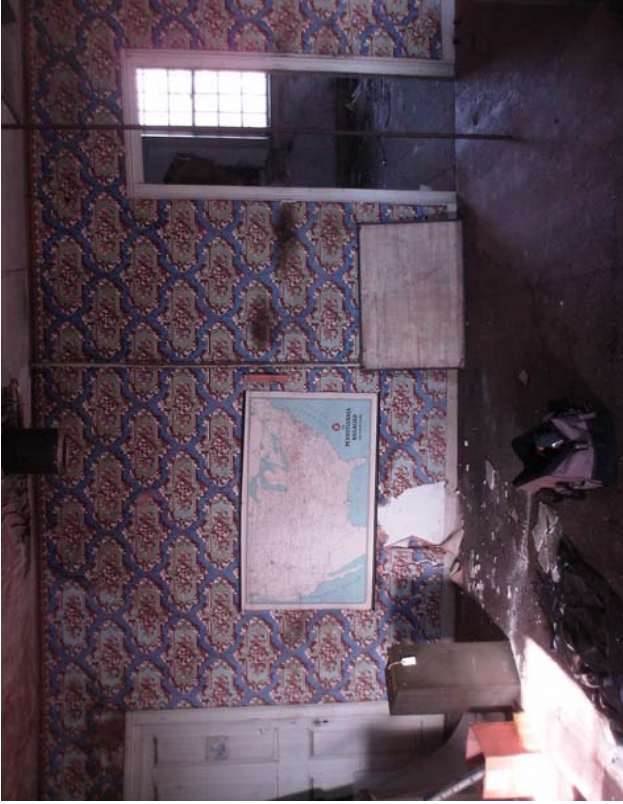
#5) Note the significant deflection of the second floor walls, with the low point at the intersection of all 3 partition walls. (Office "A")
