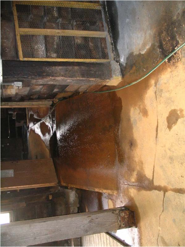
#66) Concrete cast-in-place ramp connects the main Factory "D" to the Forge "A." Note that the ramp is covered with water. (Factory "A")
