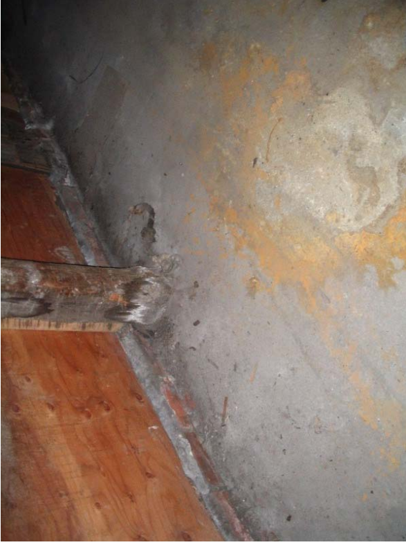
#83) Deteriorated post base with no connection to foundation. (Factory "C")
