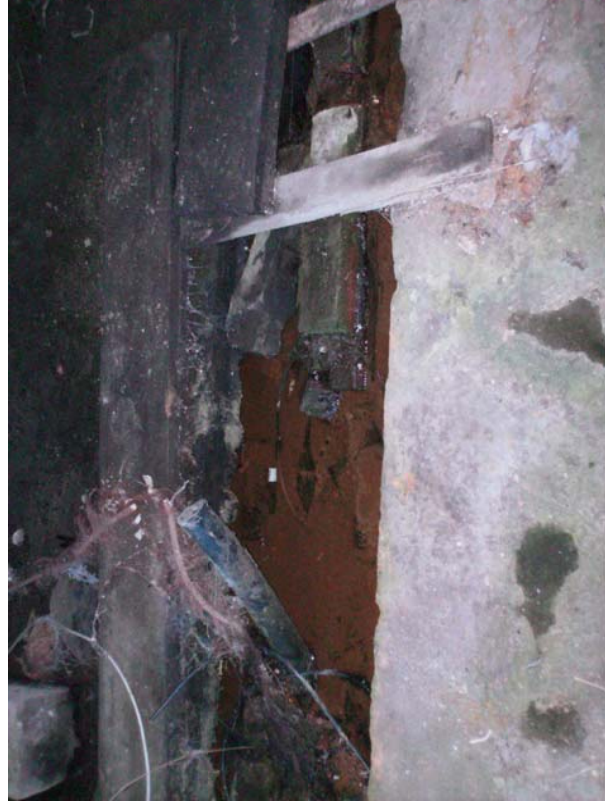
#7) The water in the ditch was flowing to the point that it was undermining the adjacent slab. (Office "A")
