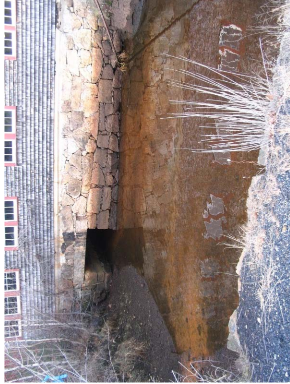
#64) Culvert exit from under the building. (Refer to "Inspections of underwater structures" Report dated March 2008 by Inner Tech Marine Services, LLC for culvert condition.) (Factory "D")
