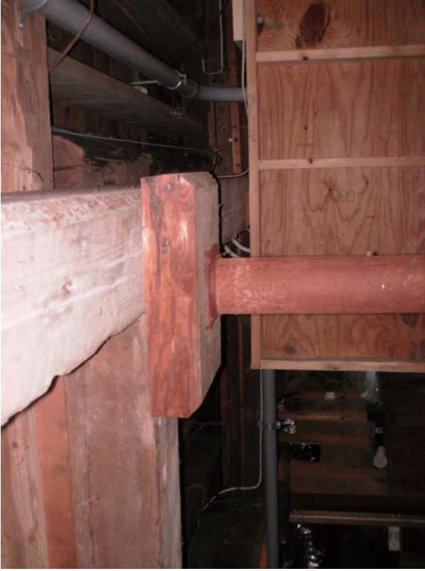
#9) Wood column "Capital" view atop steel lolly column. Note that the wood column cap is not mechanically fastened to the beams. (Office "A")
