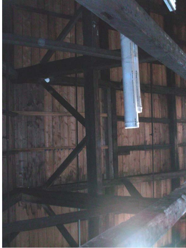
#39) Lateral bracing of the truss king post (Freight "A")
