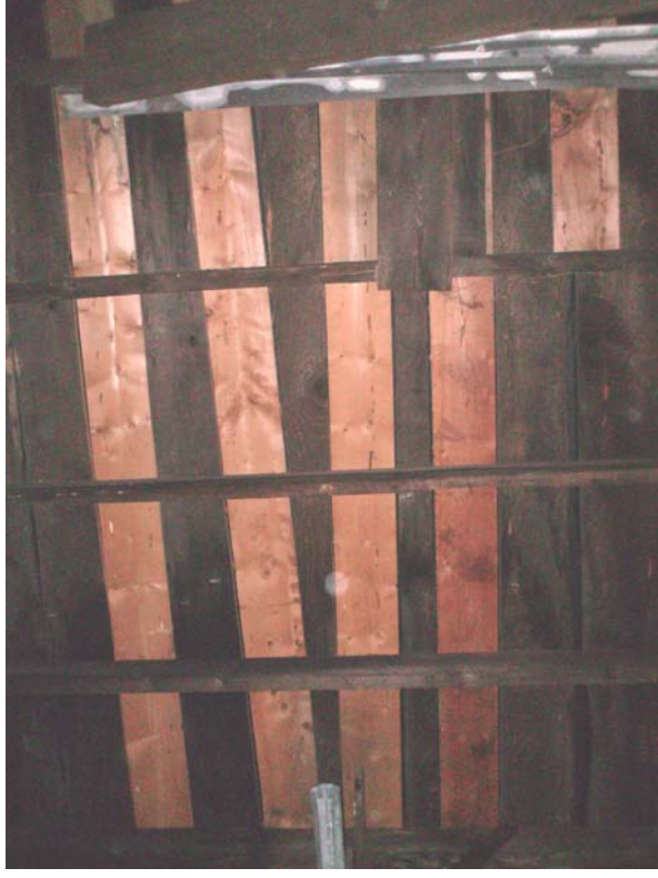
#46) The rafters bear on a 3"x5" beam spanning between trusses and provide limited bearing area for the rafters. (Freight "A")
