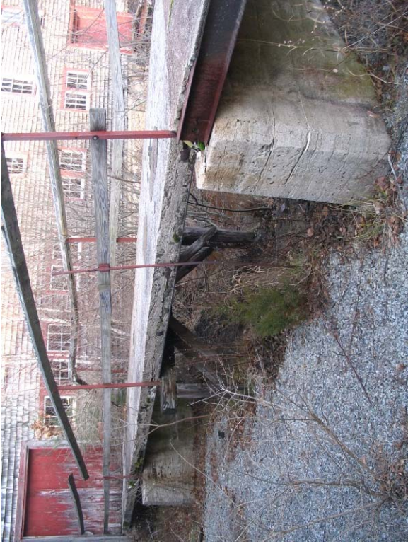
#62) Concrete bridge and platform, the bridge is in poor shape and should be removed or replaced (Factory "ALL")
