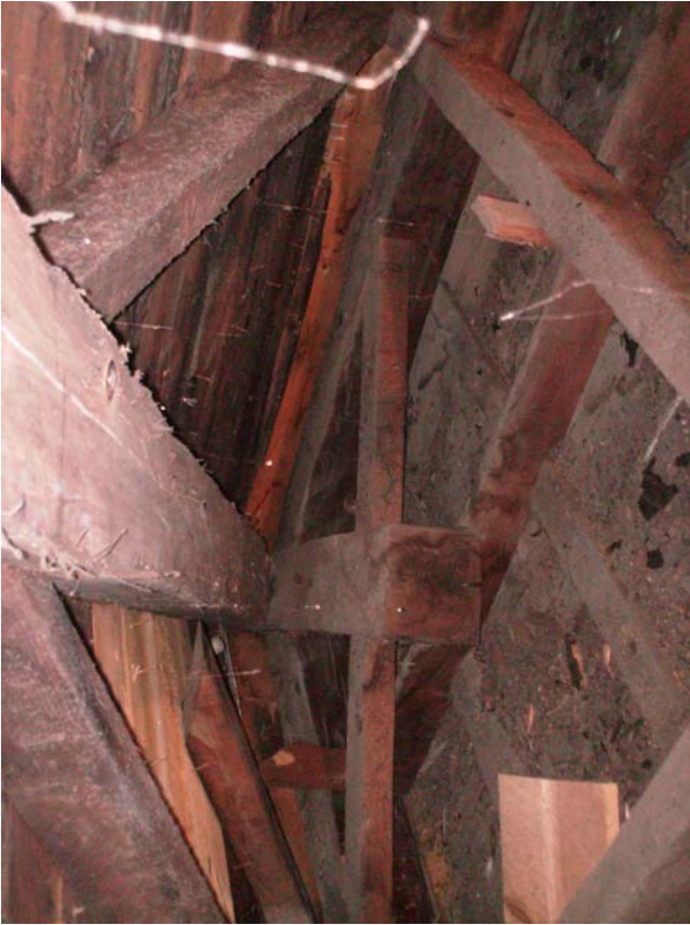
#1) Hip beam bearing on exterior wall (Note: Not all rafters attached to hip beam, proper connections should be provided.) (Office "A")
