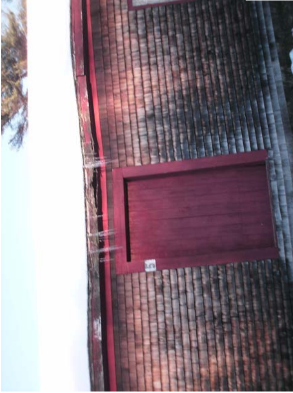
#54) Dip in roof at truck door #5, likely due to the deflection of the roof rafters and purlins (Freight "A")
