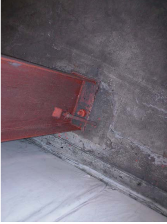
#18) Connection of cross bracing cable to column (Steel Bldg.)
