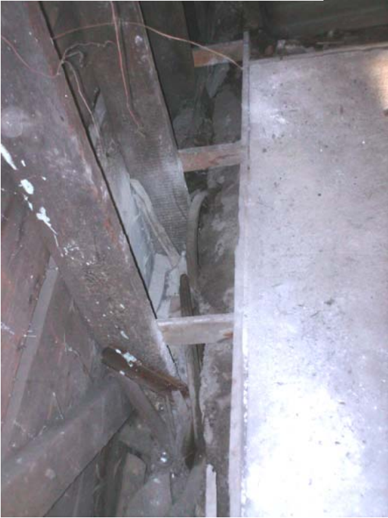
#50) View of the forming used to pour the raised slab. (Freight "B")
