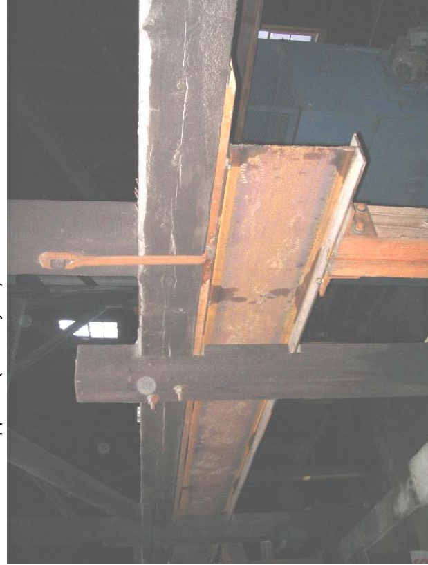
#88) Steel beam supporting the main trusses. Note that the steel beam is supported on 8x8 wood posts. (Factory "D")
