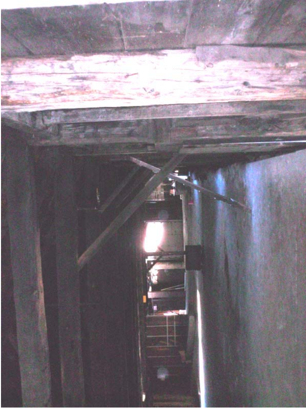
#37) Diagonal uplift ties at most trusses, Note that at some trusses these have been removed. (Freight "A")
