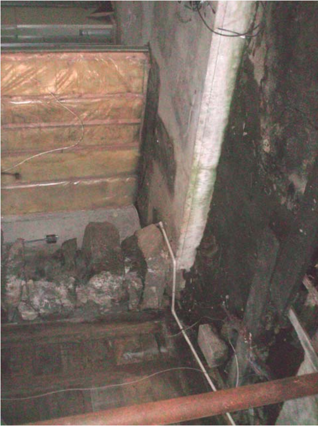
#13) Step in slab at transition between the new and original portion of the building. (Note the new portion has the higher slab elevation.) (Office "B")
