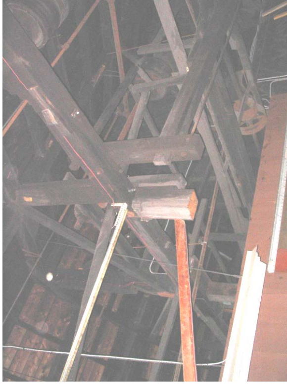
#85) Post cut under main truss; this was observed at various locations throughout the factory (Factory "D")
