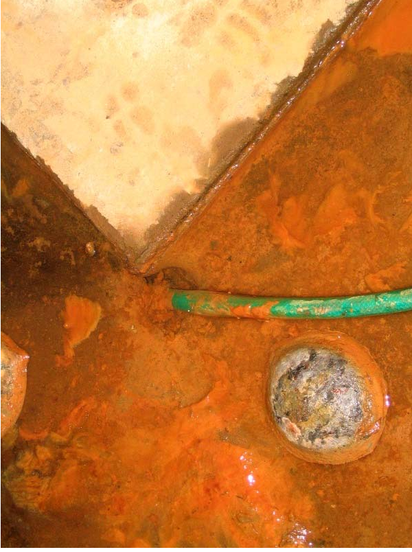
#67) Hole in concrete slab on grade filled with water. Note that the hose extends 4"-5" into the hole, due to undermining of the slab. (Factory "A")
