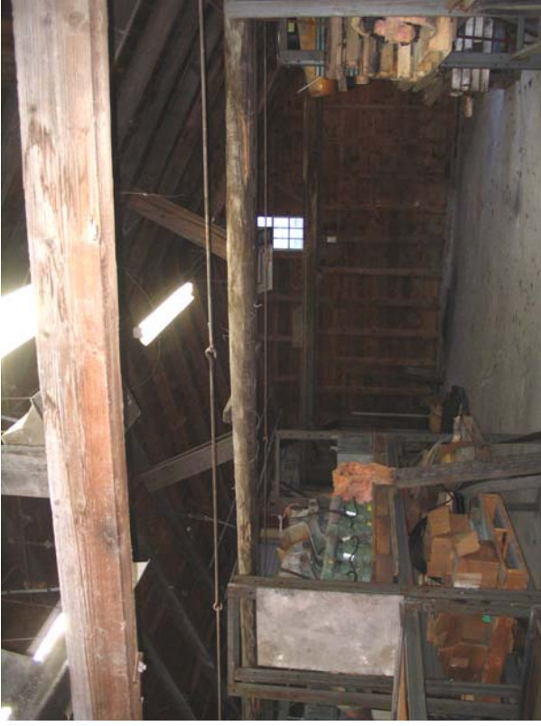
#26) Timber cross members at top of wall were attempted to be turned into tusses. Also, steel ties used to try and prevent the wall from spreading. (Pickling)
