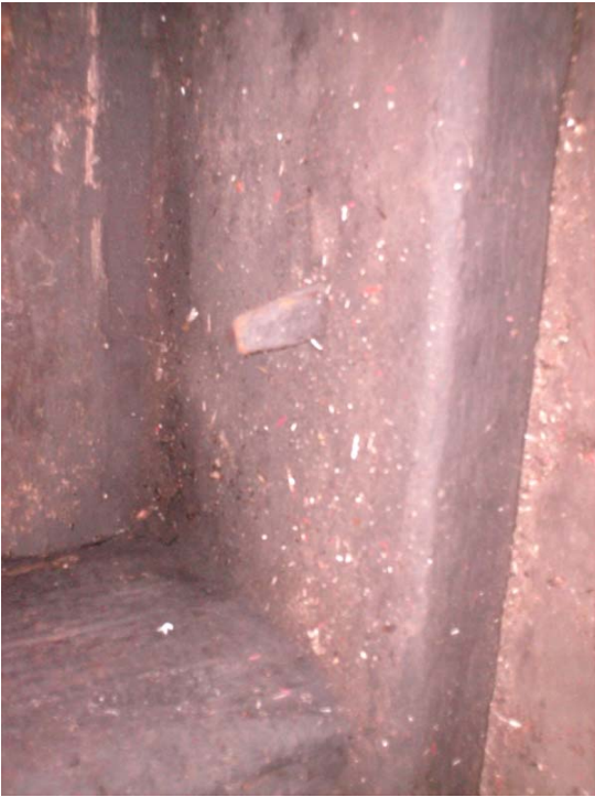
#106) Connection of sill to rubble foundation via steel wedge. (Factory "D")
