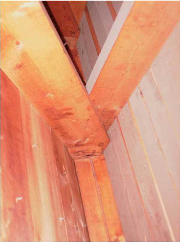
#21) Roof rafter to exterior wall connections, no tie downs were observed. (Restroom)
