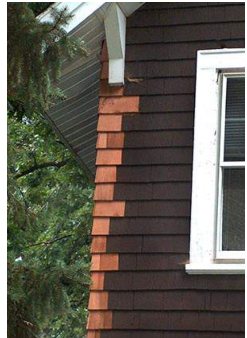
Figure 7. One of the advantages of wood shingles as a wall covering is that individual shingles that are damaged can easily be replaced. On this highly exposed corner, worn shingles have been selectively replaced to help safeguard against water damage. The new shingles will be stained to match the existing shingles.
