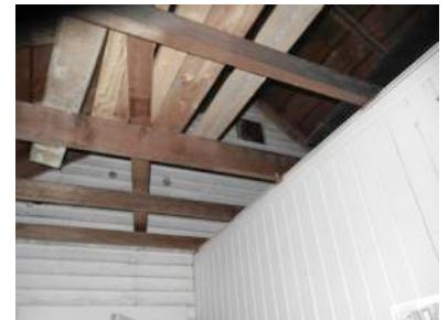
DS-8 Roof framing at storage addition
