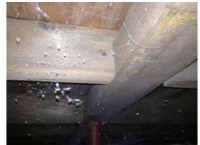
UC-17 Joists notched into beam
