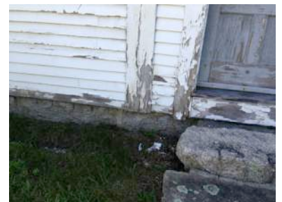
DS-4 Missing masonry joint at storage addition
