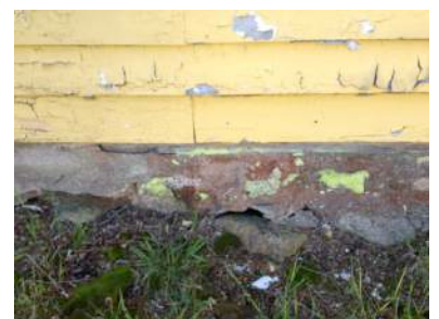
KH-5 Fieldstone foundation needs selective repointing
