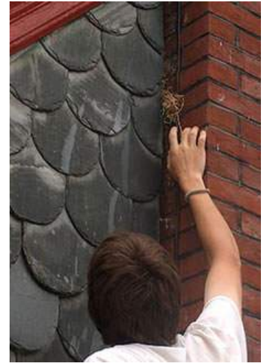
Figure 14. When inspecting connections between projections and the main building, look for areas where birds, bees and pests may enter or nest. Birds have been nesting in this porch roof and the area is being cleaned of their debris. Where an opening exists, it may be necessary to cover it with a trim piece, screening, or sealant. Photo: Bryan Blundell
