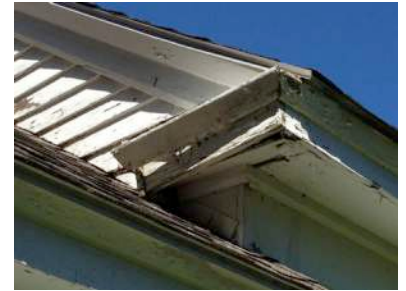
DS-6 Damaged & missing trim at eave
