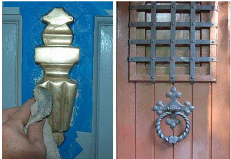
Figure 1. Maintenance involves selecting the proper treatment and protecting adjacent surfaces. Using painter's tape to mask around a brass doorknocker protects the painted door surface from damage when polishing with chemical compounds. On the other hand, hardware with a patinated finish was not intended to be polished and should simply be cleaned with a damp cloth.
