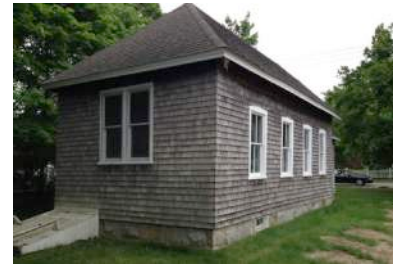
UC-1 Hip roof at east end of Chapel
