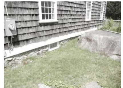
FT-3 East wall bulge behind granite boulder
