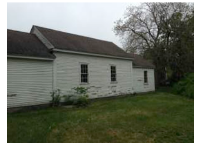
DS-7 Existing asphalt shingle roof
