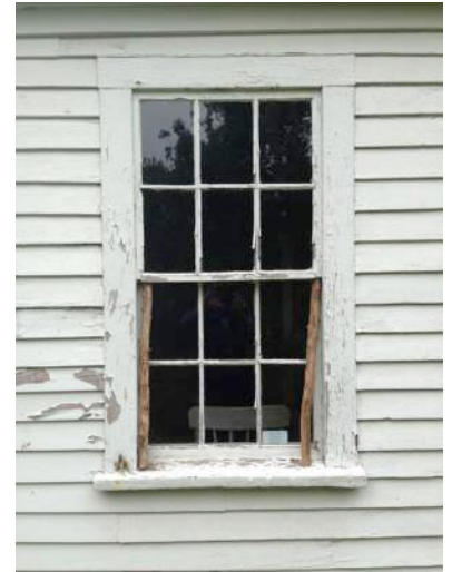
DS-10 Existing 6/6 wood double-hung window
