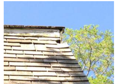
KH-13 – Missing & worn out roof shingles
