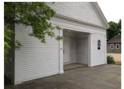
MH-4 Bluestone paving at main entrance
