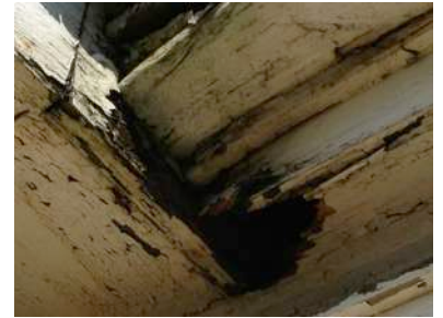
KH-16 Rodent & water damage
