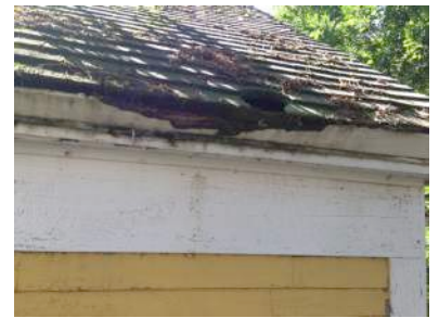
KH-12 Rodent damage at rotten trim
