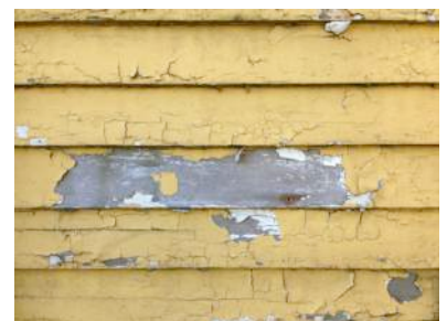
KH-9 Failed exterior paint – typical
