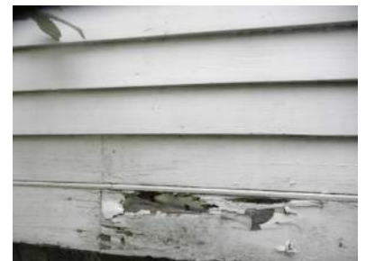
MH-19 Insect damage
