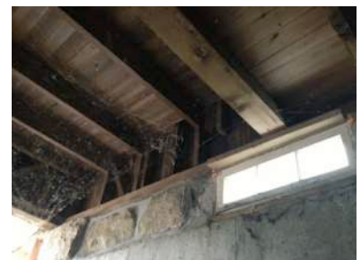
UC-20 Existing foundation & floor framing
