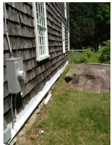
FT-7 Bulging east wall
