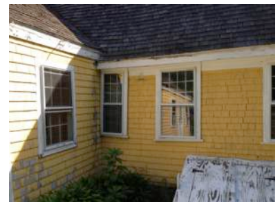
KH-15 Missing downspouts
