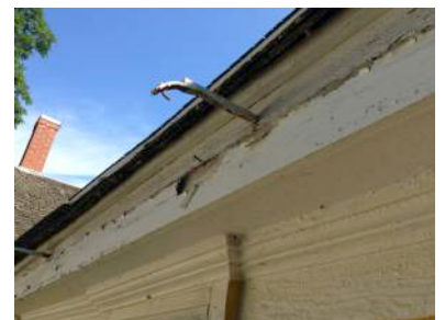
KH-14 Existing gutter hangers
