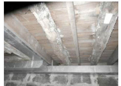
KH-18 Existing framing with reinforcements
