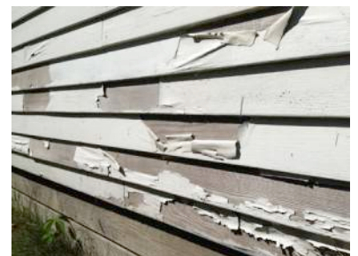
DS-5 Failing paint at east side
