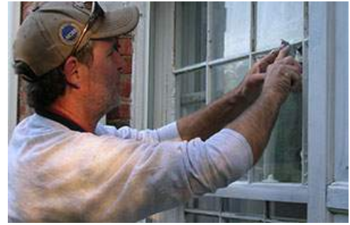
Figure 11. Glazing putty should be maintained in sound condition to prevent unwanted air infiltration and water damage. New glazing putty should be pulled tight to the glass and edge of the wood, creating a clean bevel that matches the historic glazing
