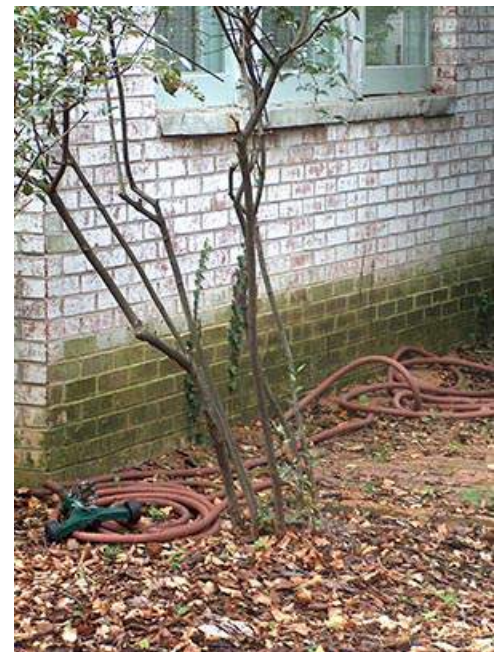
Figure 16. This chronically wet area has a mildew bloom brought on by heat generated from the air-conditioning condenser unit. The dampness could be caused by a clogged roof gutter, improper grading, or a leaking hose bibb.
