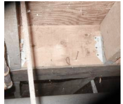
MH-17 Reinforced floor framing
