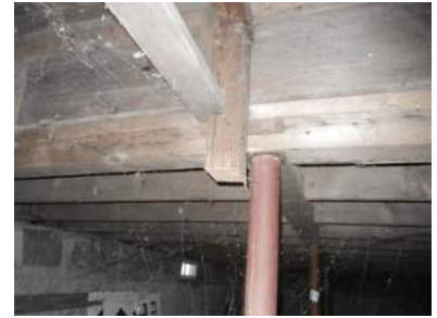
UC-16 Center beam supported by columns
