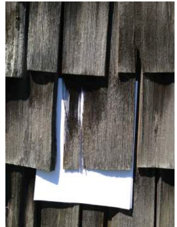
FT-6 Worn out wood shake siding
