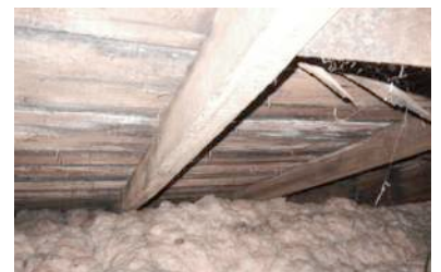
MH-9 Broken roof sheathing
