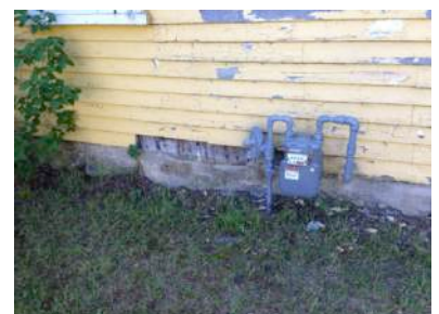
KH-10 Missing clapboard
