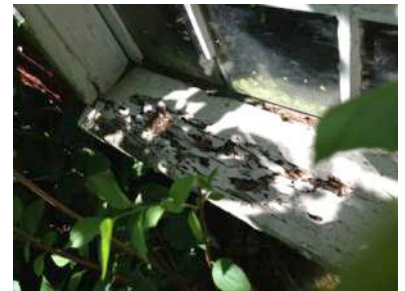
KH-21 Insect damage at basement window sill
