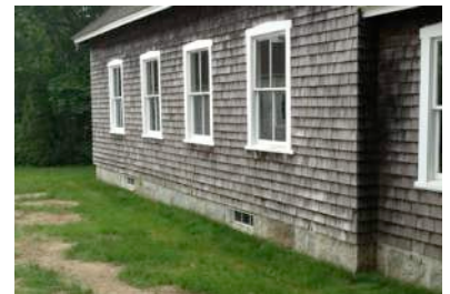
UC-7 Pitch grade away from foundation
