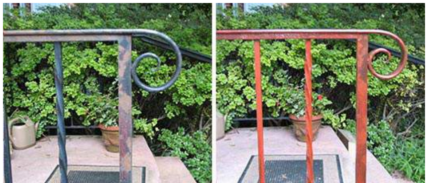
Figure 15. Metal projecting elements on a building, such as sign armatures and railings, are easily subject to rust and decay. Proper surface preparation to remove rust is essential. Special metal primers and topcoats should be use
