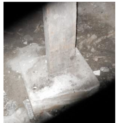
MH-16 Existing concrete footing
