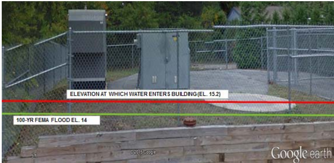
Figure 69 Hathaway Pump Station
