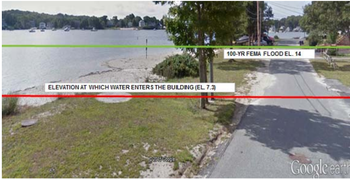
Figure 38 Riverside Pump Station
