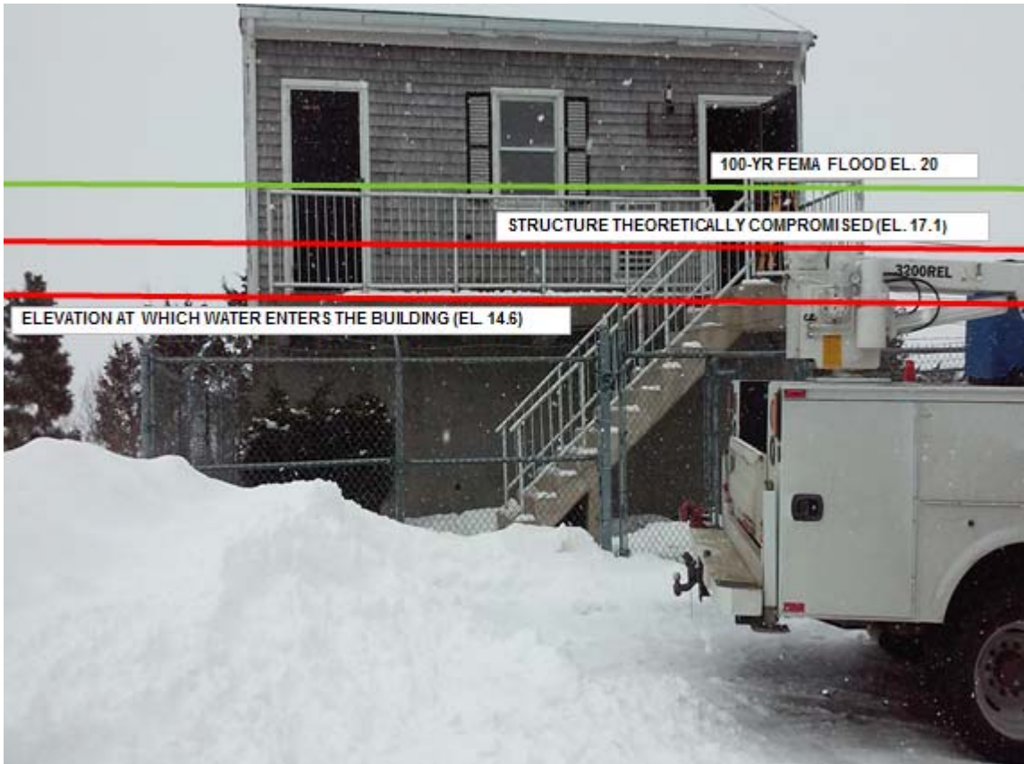
Figure 27 Ruggles Pump Station
