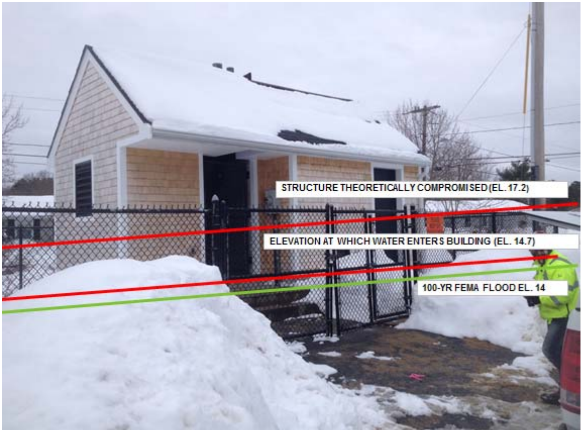
Figure 71 Terry Lane/Pine Tree Estates (Terry Lane) Pump Station
