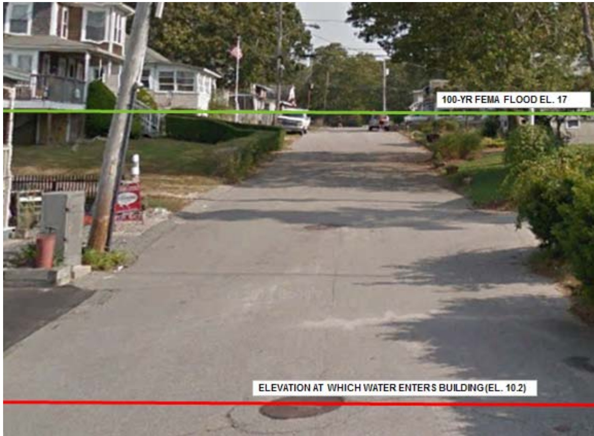
Figure 6 Bay Street Pump Station
