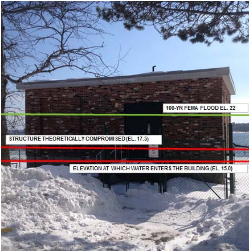
Figure 25 Onset Pier Pump Station
