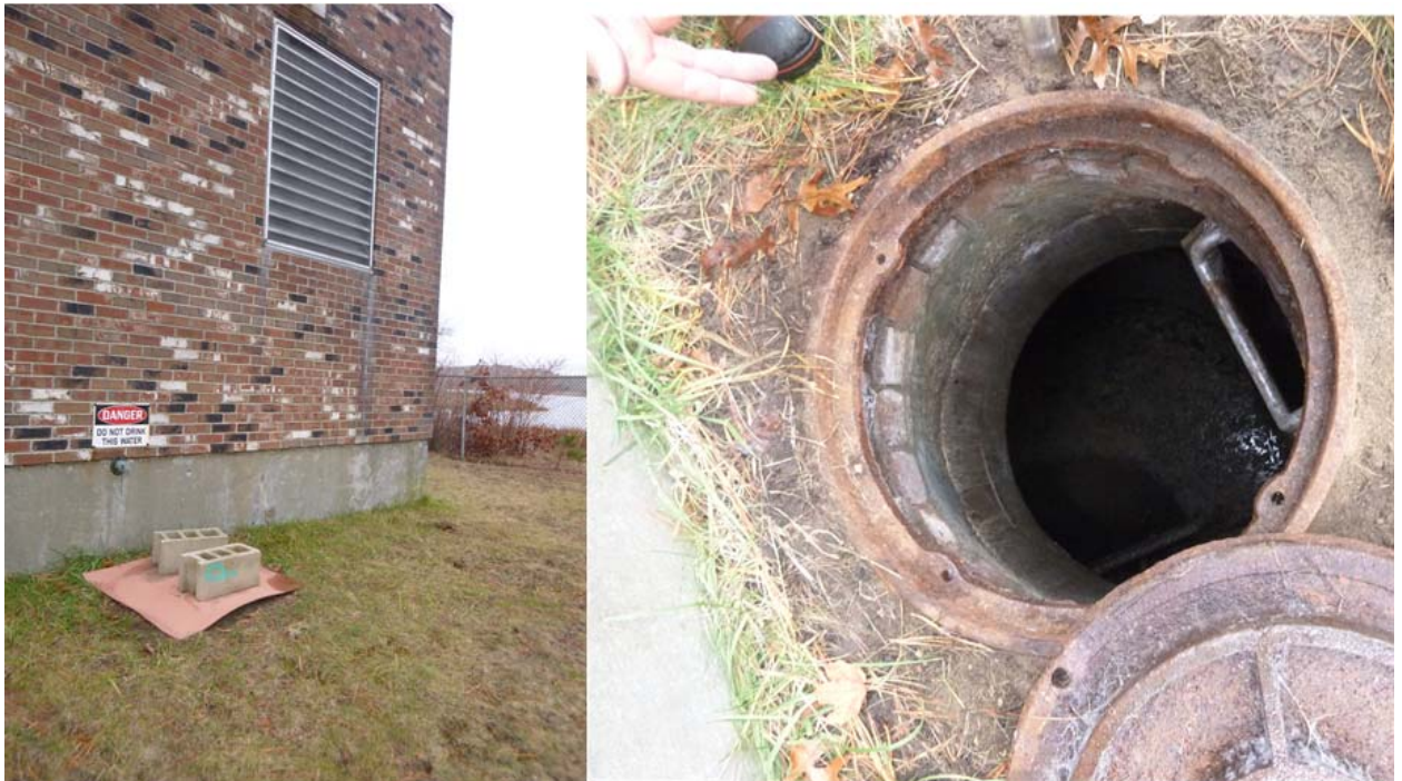
Figure 55 North Boulevard Wet Well Manhole Cover
