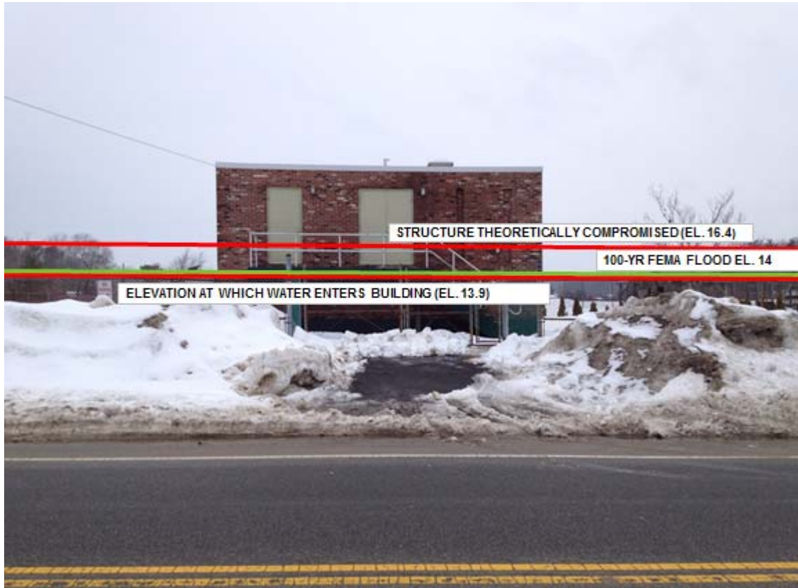
Figure 57 Hynes Field Pump Station
