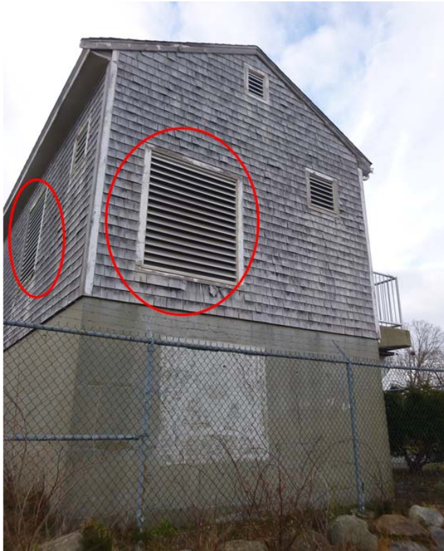
Figure 28 Ruggles Potential Water Entry Points
