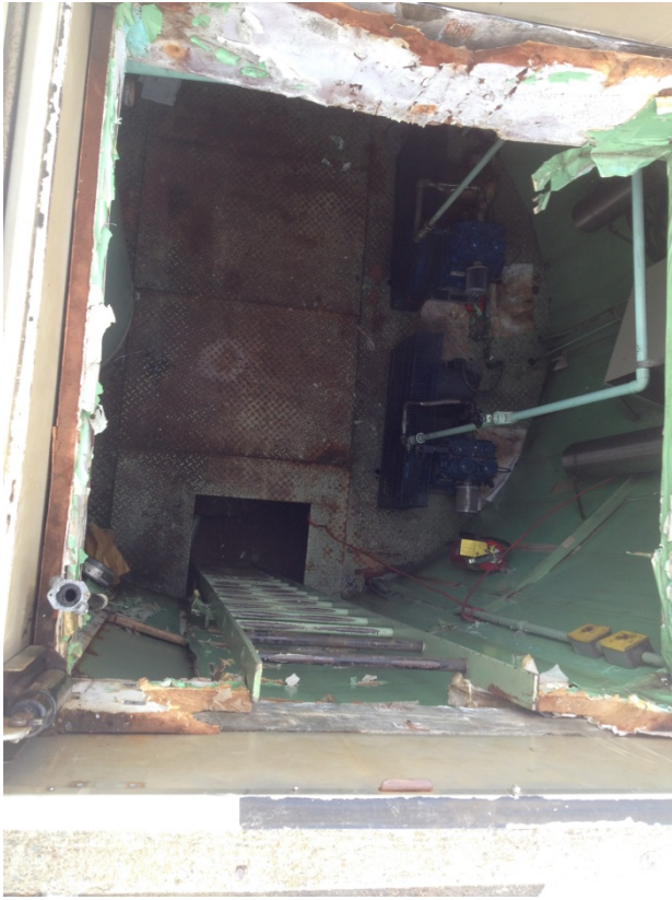
Figure 10 South Boulevard Substructure
