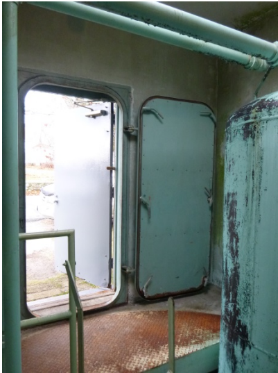
Figure 61 East Boulevard Watertight Door
