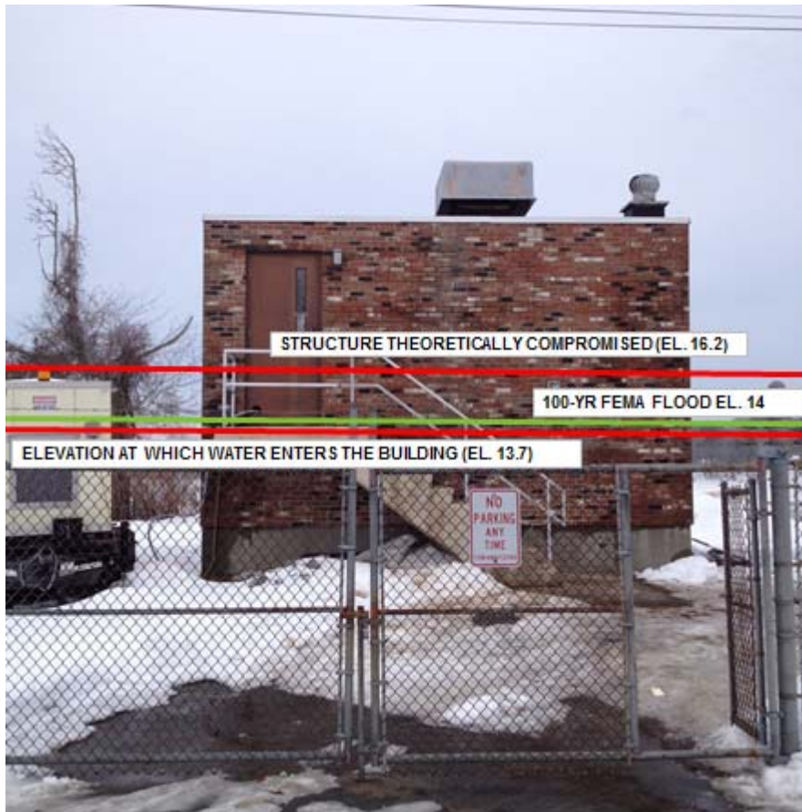
Figure 54 North Boulevard Pump Station
