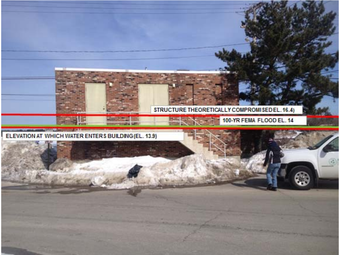
Figure 45 Narrows Pump Station
