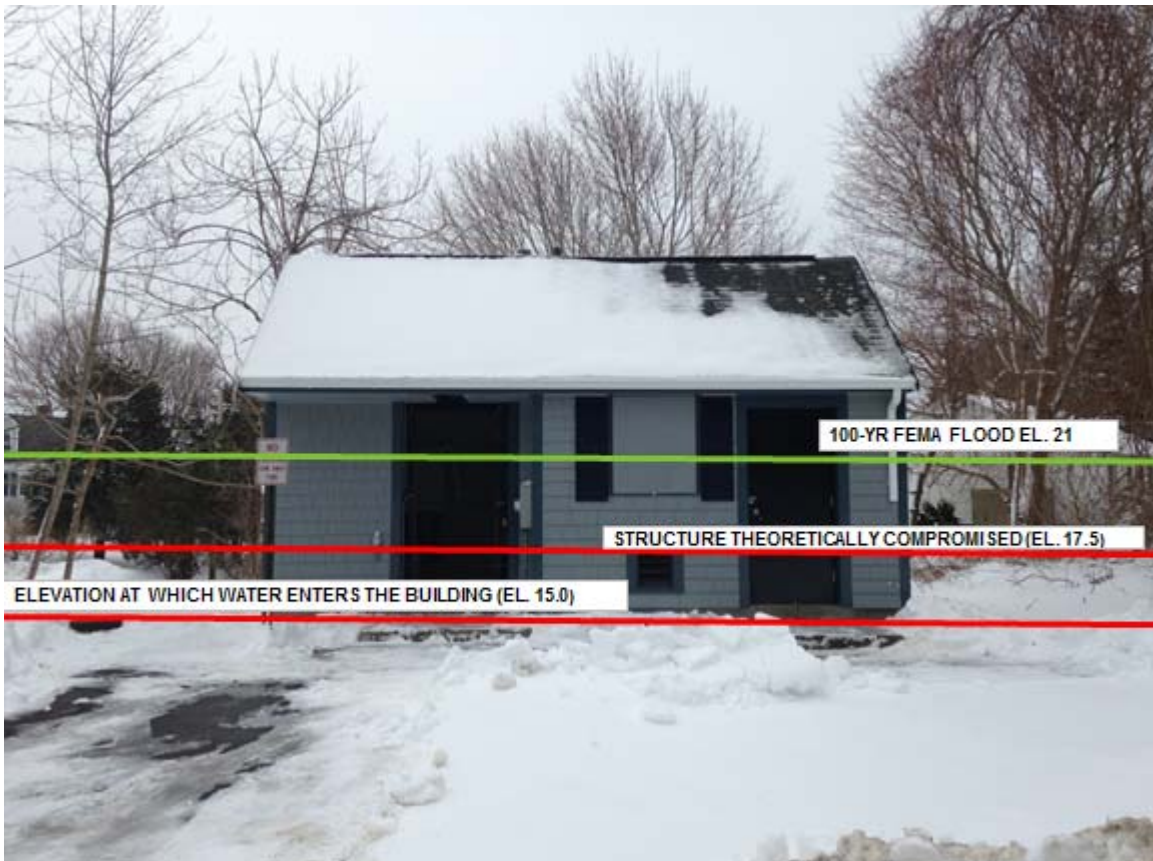
Figure 12 Hill Street Jefferson Shores Pump Station
