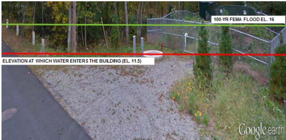
Figure 30 Cromessett Road Pump Station
