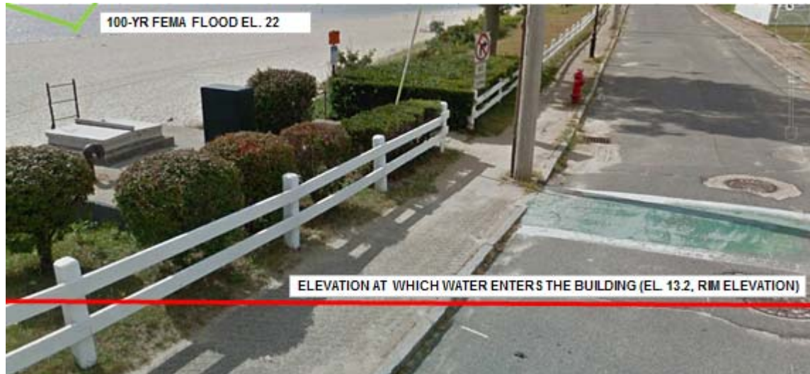
Figure 9 South Boulevard Pump Station
