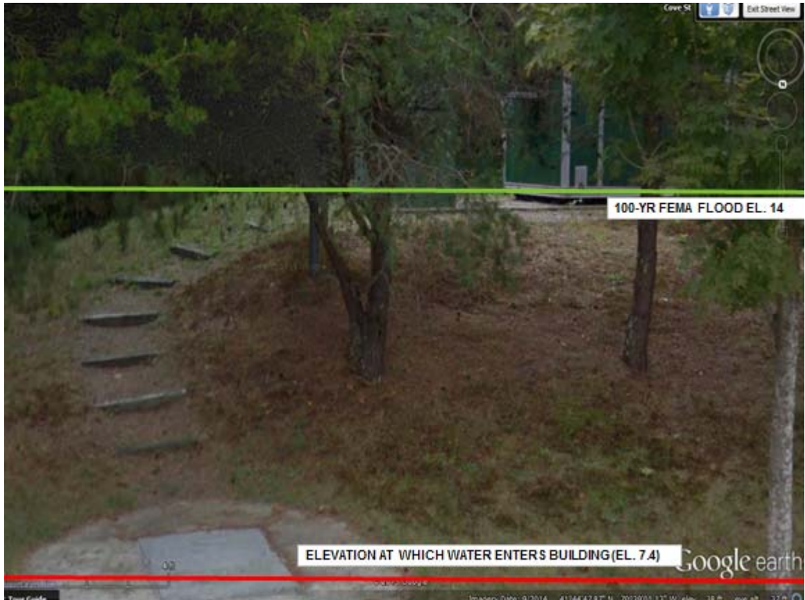
Figure 36 Onset Heights Pump Station
