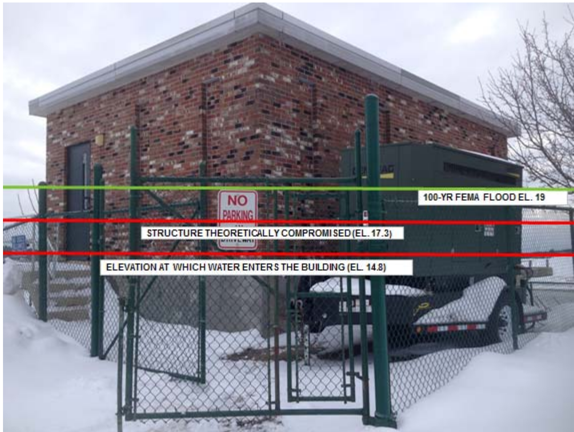
Figure 23 South Water Street Pump Station
