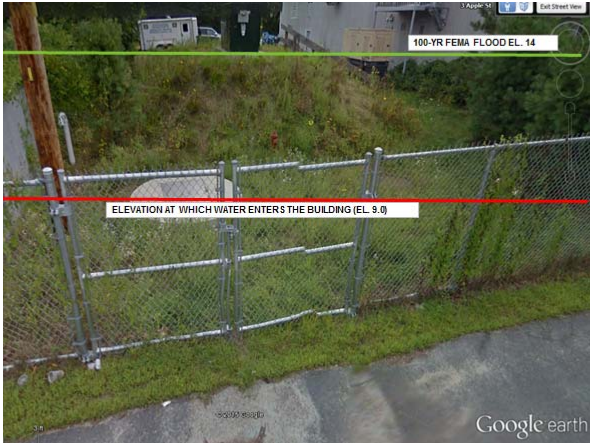
Figure 34 Apple Street Pump Station
