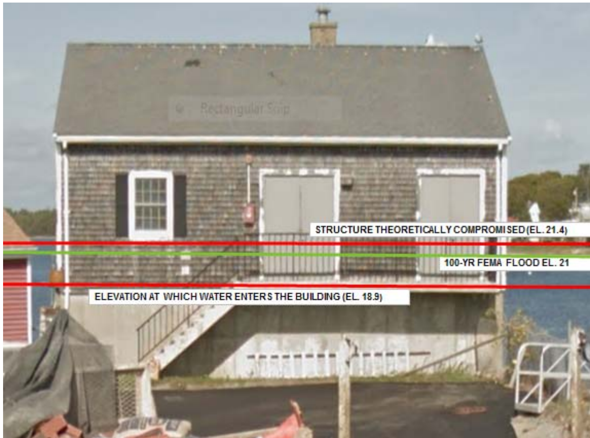
Figure 19 Cohasset Narrows Pump Station
