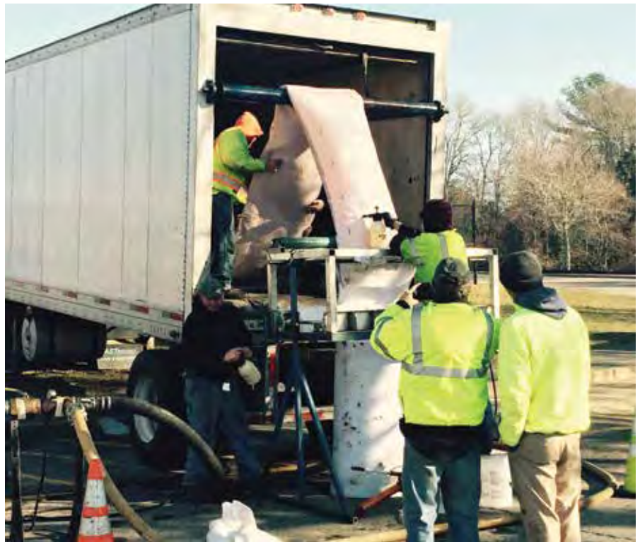
Liner Installation 21-inch RCP at Viking Drive near Wareham Middle School
