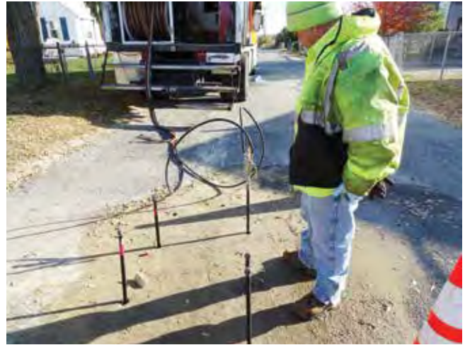
Grout was inserted on both sides of the pipe deflection
