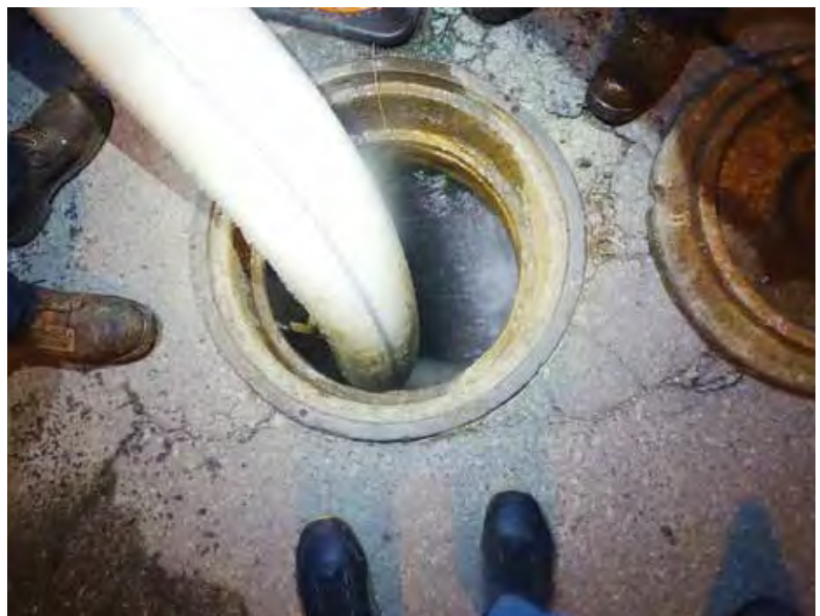
Liner inversion and curing worked very well at pipe deflection
