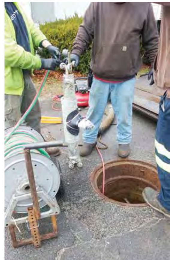
Tee Liner with inflatable packer assembled and ready for insertion
