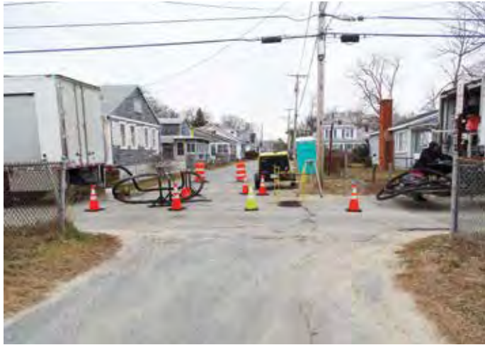
Tight working conditions, narrow streets, minimal site impact
