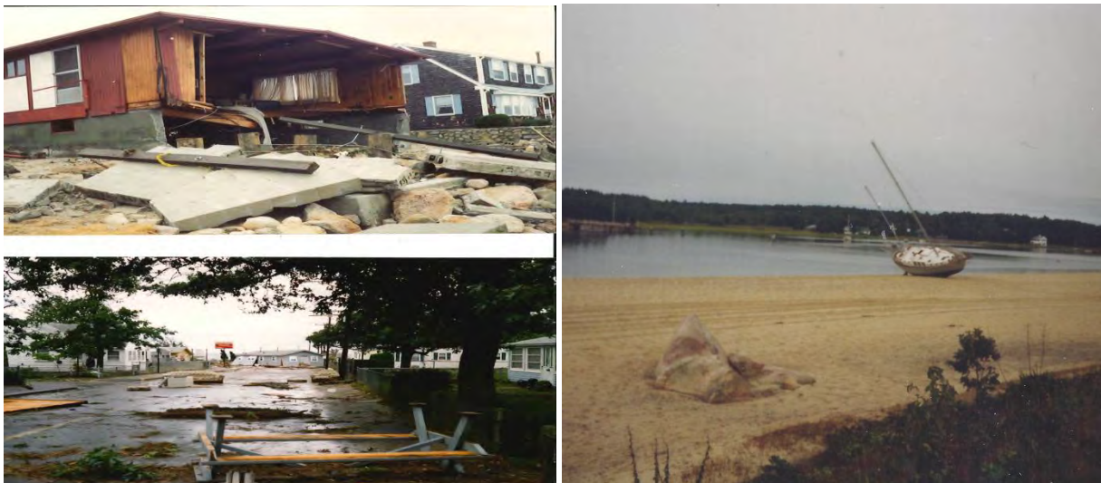
Figure 3-11. Impacts to the homes and roadways in the Swifts Beach area (left 2 photos) and to boats in Onset Harbor (right) during Hurricane Bob in 1991.
