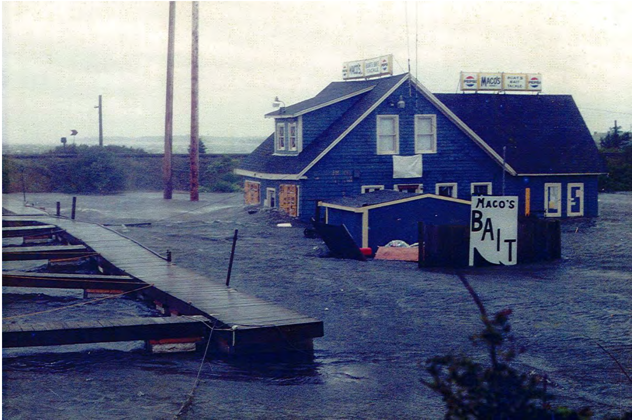
Figure 3-1. Coastal flooding impacting Maco's Bait Shop during Hurricane Bob (1991).
