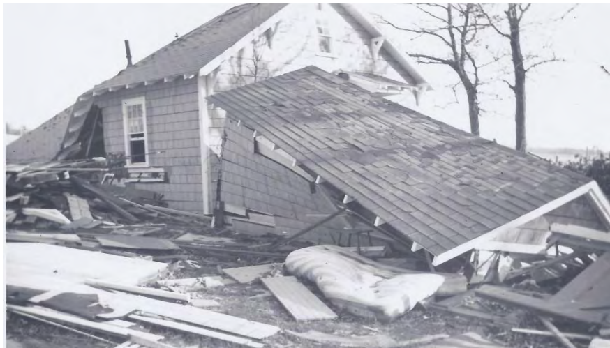
Figure 3-14. Wind-damaged home during Hurricane Edna (1954).
