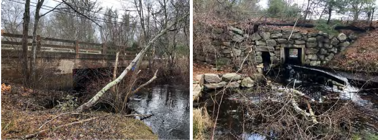
Figure 3-27. Fearing Hill Road Bridge (left) and Main Street culvert at Old Trout Farm (right).
