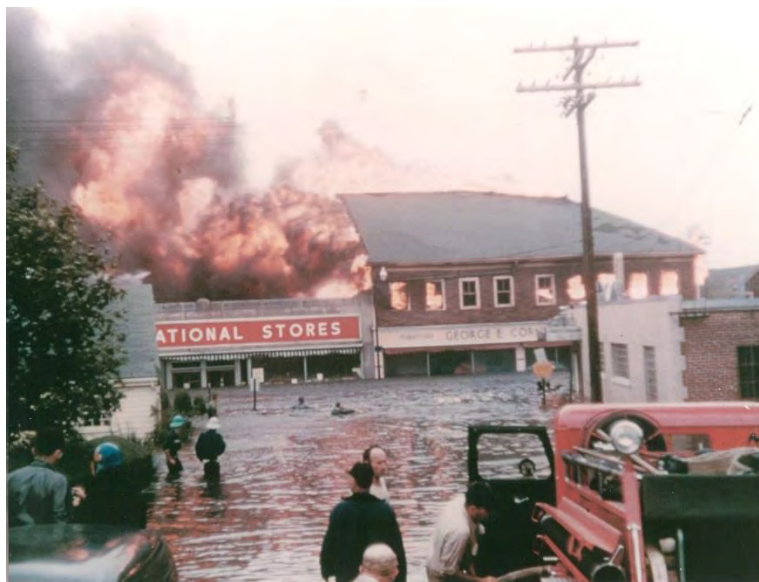
Figure 3-17. Fire impacting a department store as secondary impact from Hurricane Carol.
