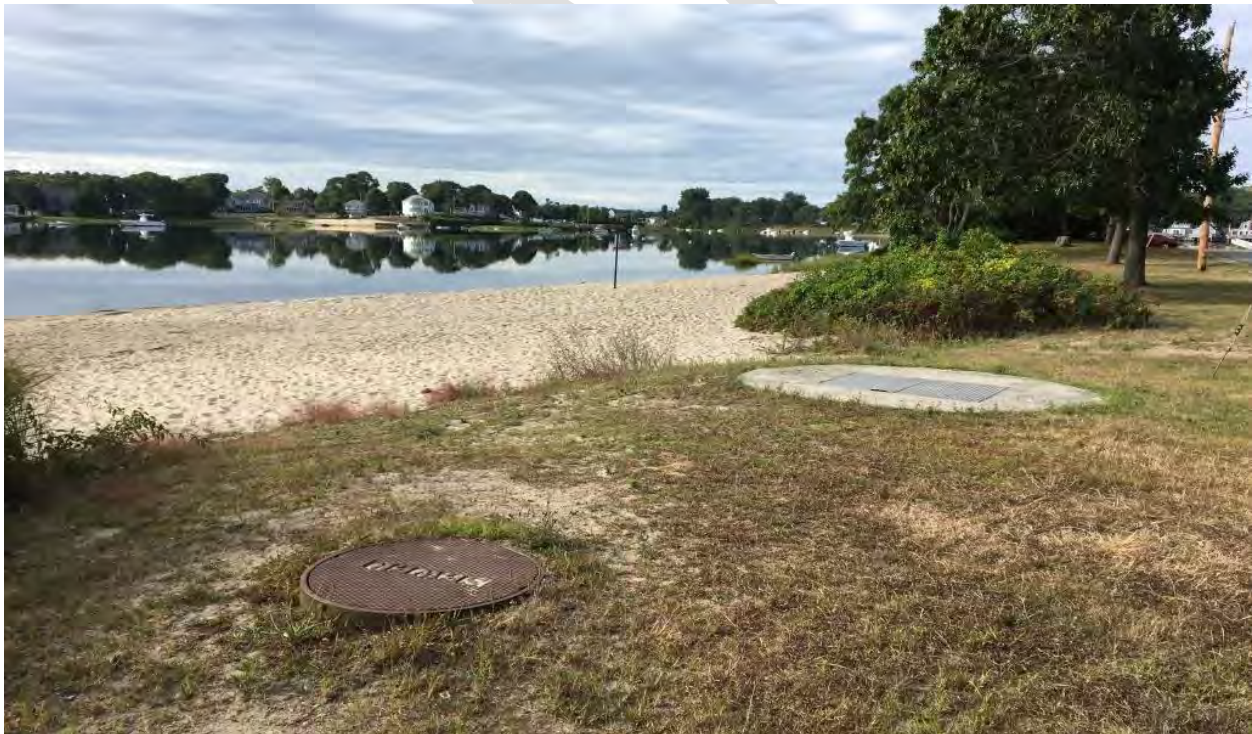
Figure 4-7. Riverside Pump Station.
