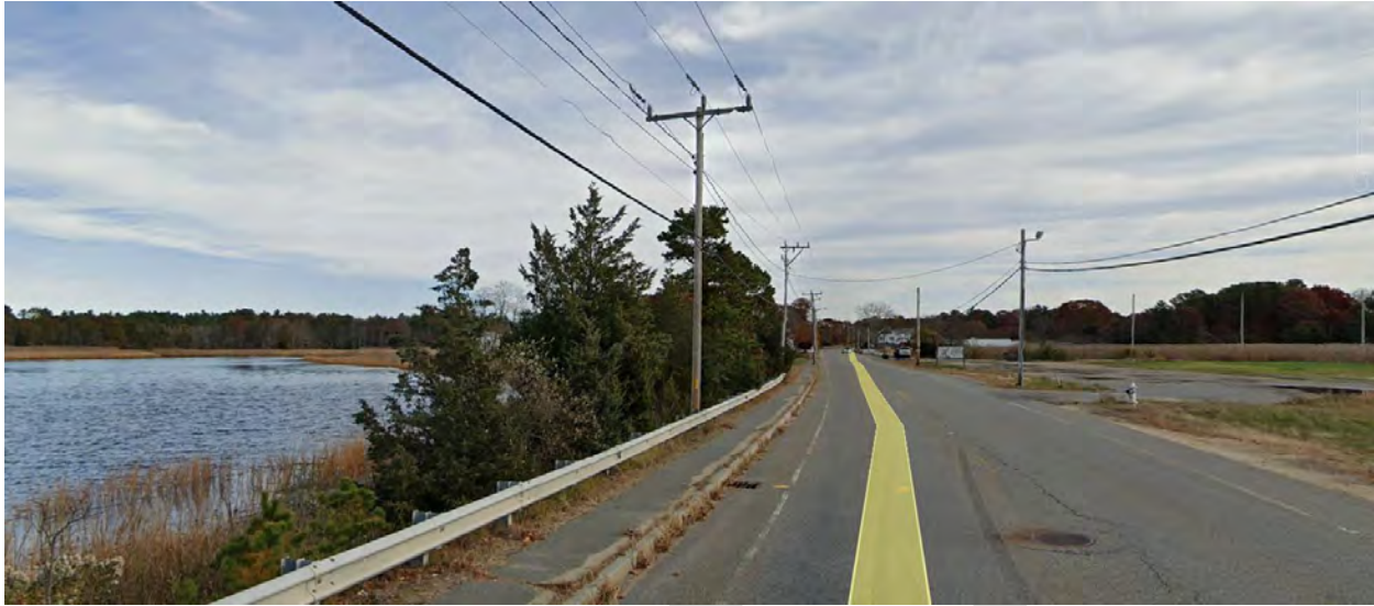
Figure 4-23. Sandwich Road, facing east, near the Golf Shots Driving Range. (Image from GoogleEarth, 2018)
