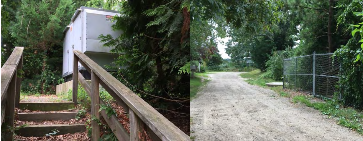
Figure 4-3. Arnold Pump Station.
