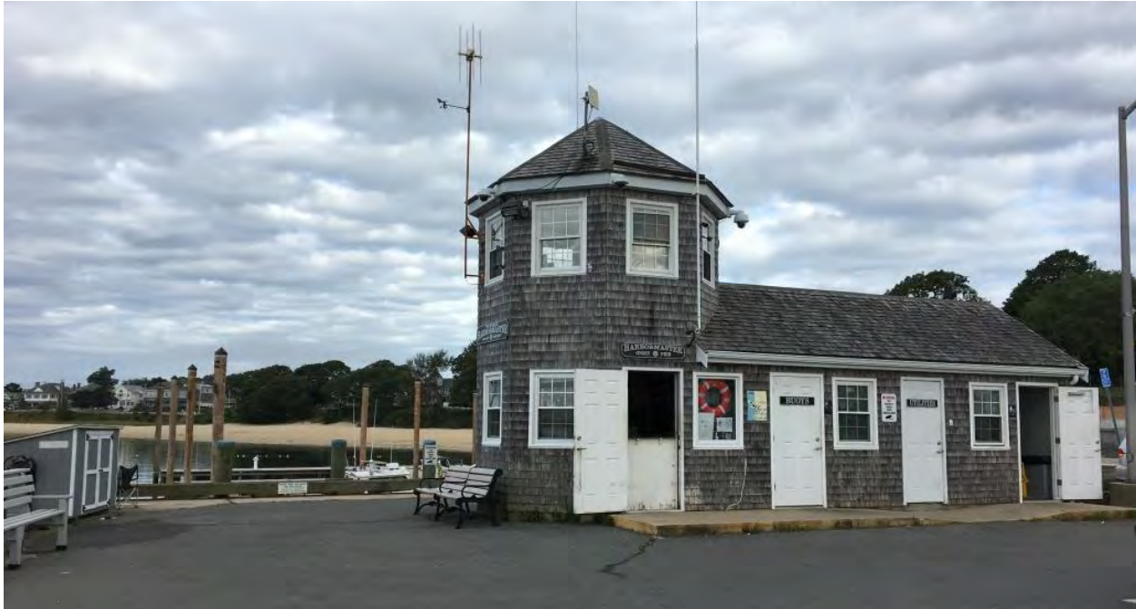
Figure 4-13. Harbormaster Building at Onset Pier.
