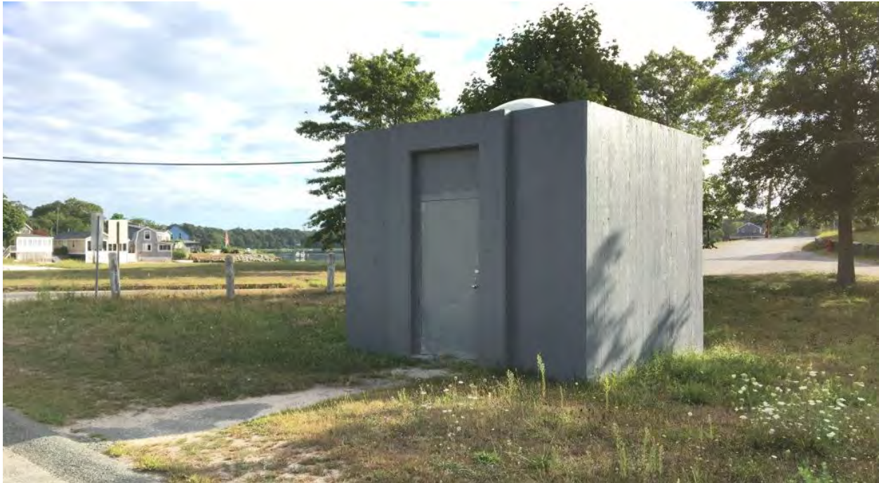
Figure 4-11. East Boulevard Ejector Pump Station.
