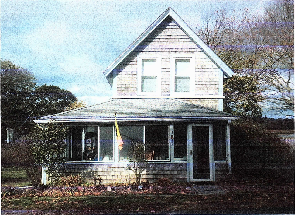
VIEW FROM WEST BLVD.
