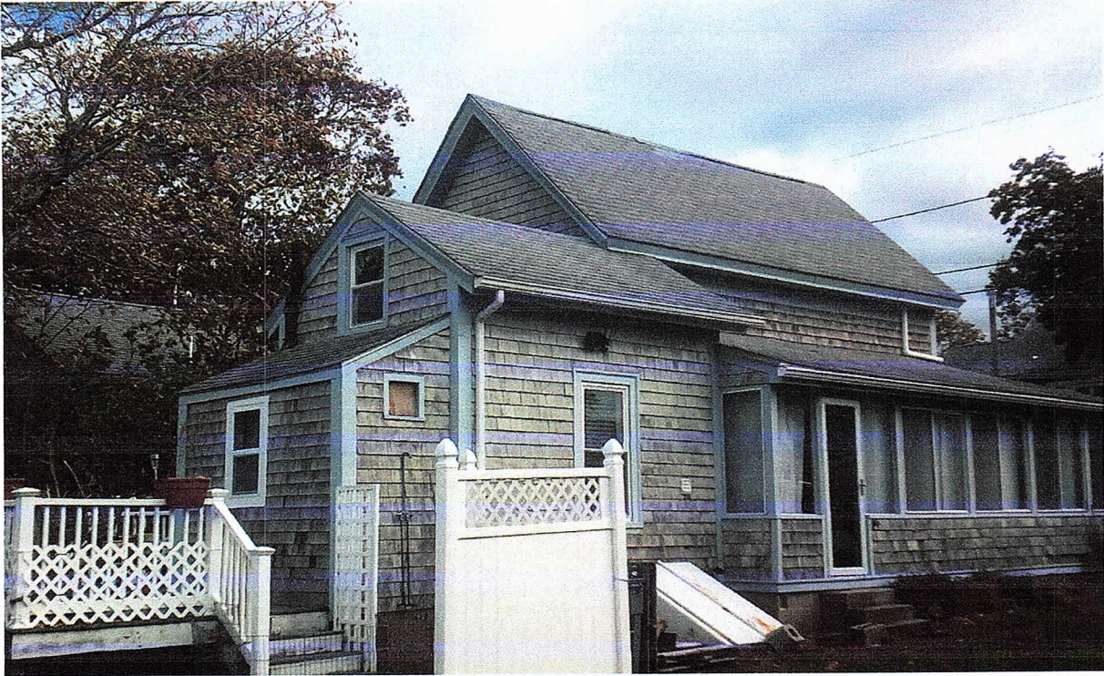
VIEW FROM SOUTHWEST (REAR)
