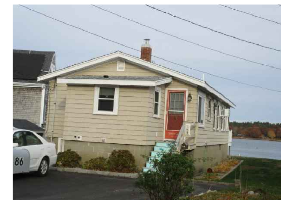
EXISTING STREET VIEW ( WEST )
