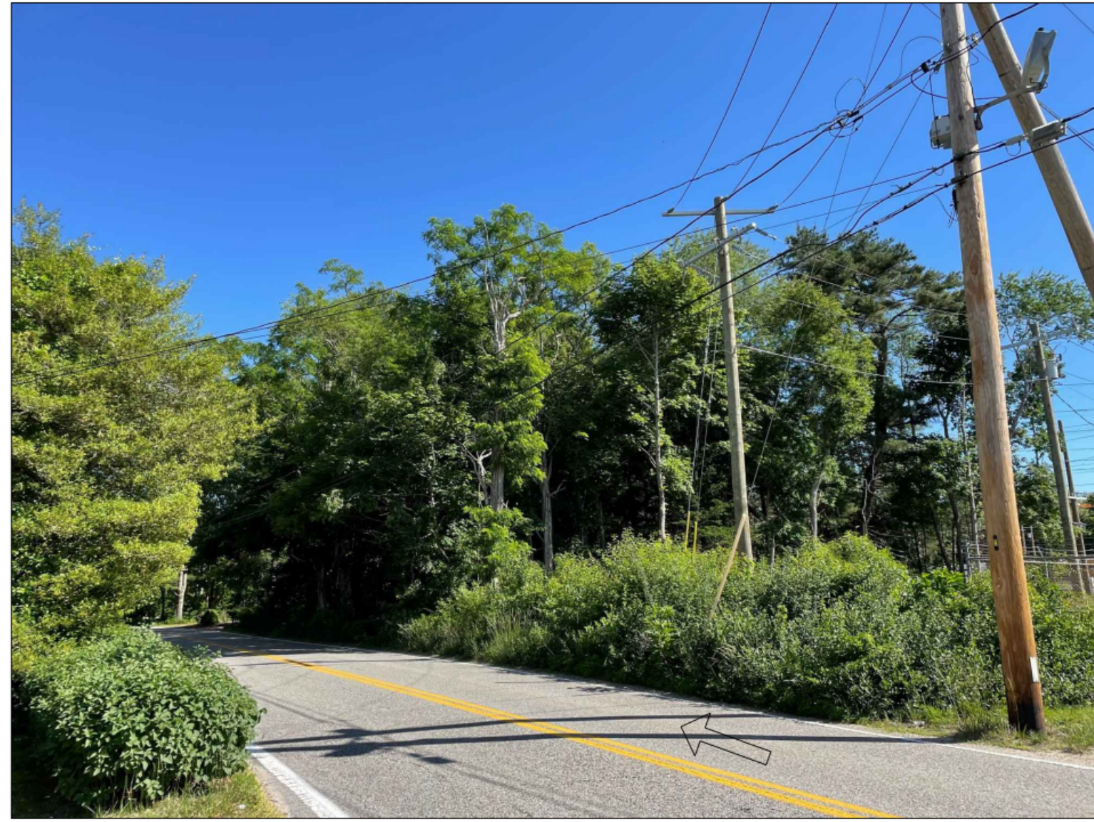
DOTY STREET LOOKING NORTH WEST
