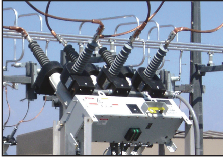
▲ 45° angle mounting for applications requiring the same load and line side connector height.
