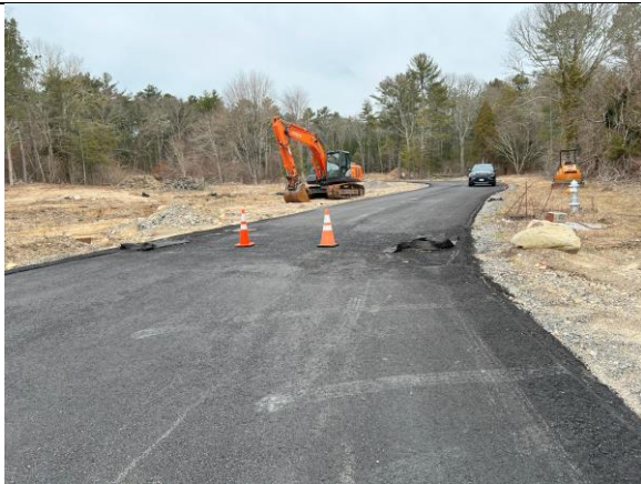
Photograph 1 – Roadway binder installation
