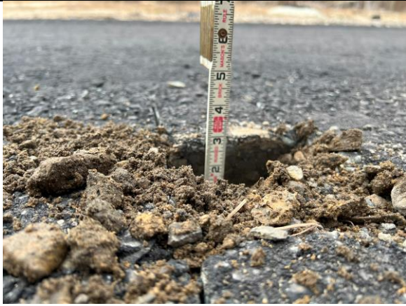
Photograph 3 – Roadway core (sta 2+50 +/-).
