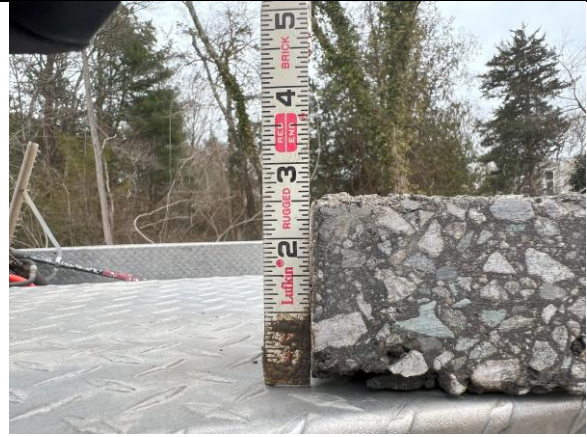
Photograph 4 – Roadway core (sta 2+50 +/-).
