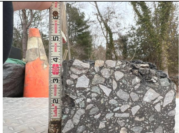
Photograph 6 – Roadway core (sta 5+00 +/-).
