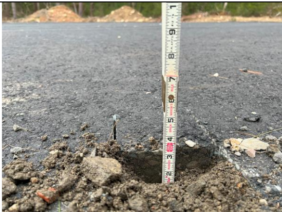
Photograph 5 – Roadway core (sta 5+00 +/-).
