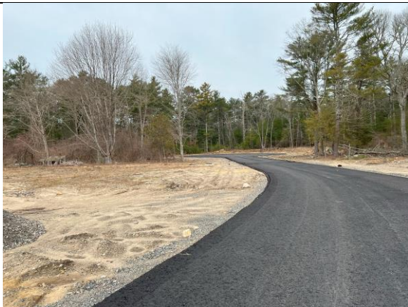
Photograph 7 – General state of Roadway, shoulders, etc.
