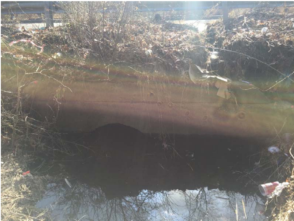
View of culvert at Sta 89+30.00 +/- (Northerly Side)
