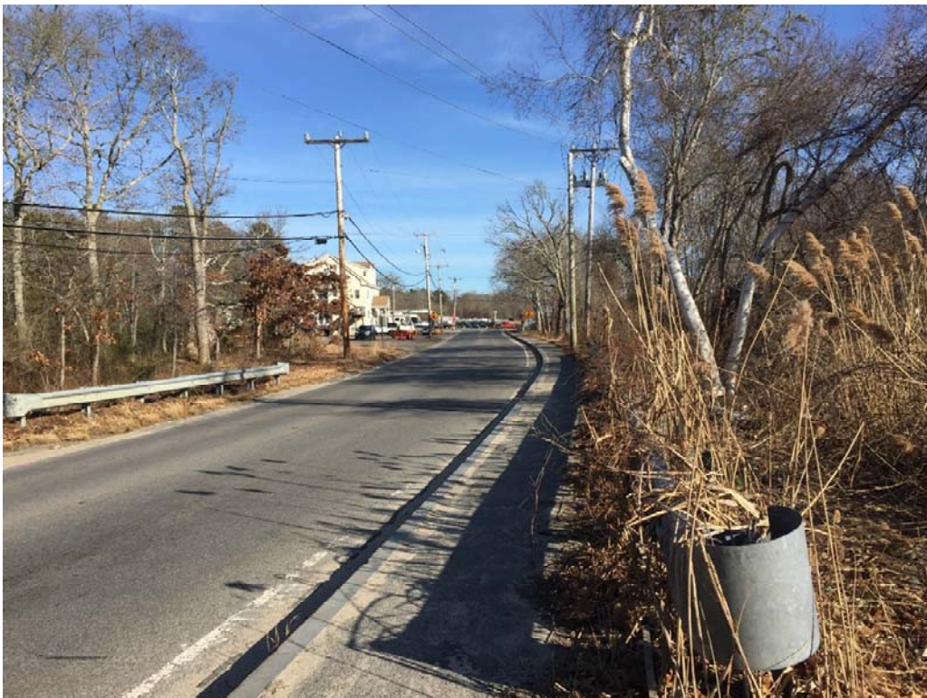
View of Minot Ave looking Eastbound at STA point 88+00 +/-
