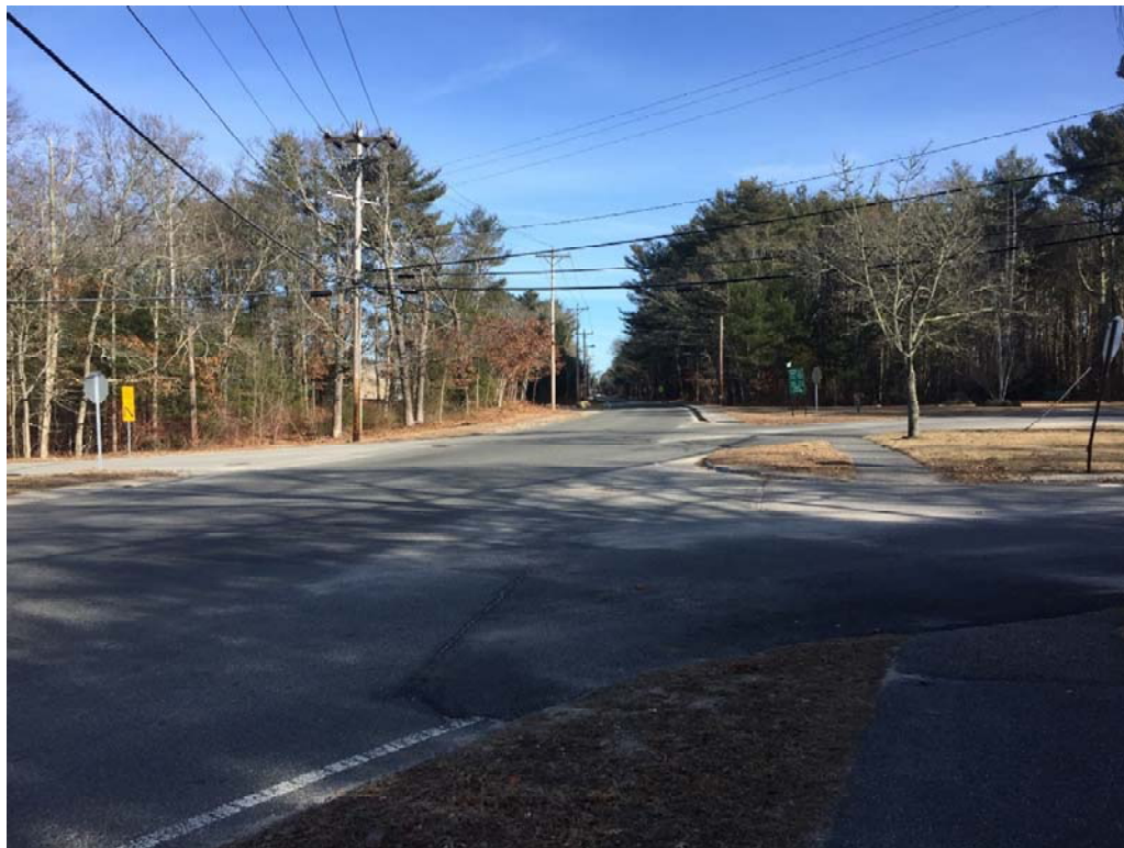
View of intersection at Narrows Rd and Indian Neck Rd looking Eastbound at STA point 20+00 +/-
