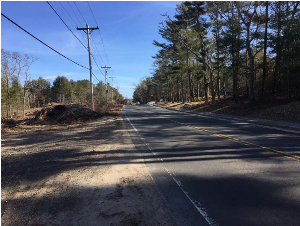
View of Minot Ave looking Eastbound at STA point 67+00 +/-
