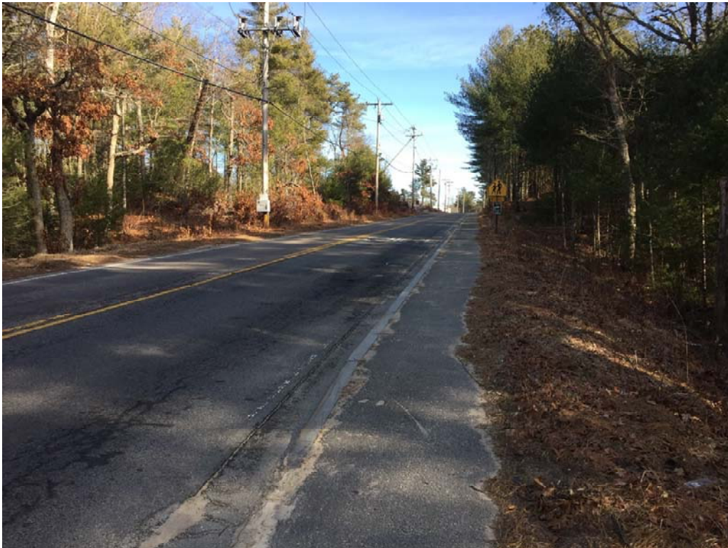
View of Minot Ave looking Eastbound at STA point 53+00 +/-
