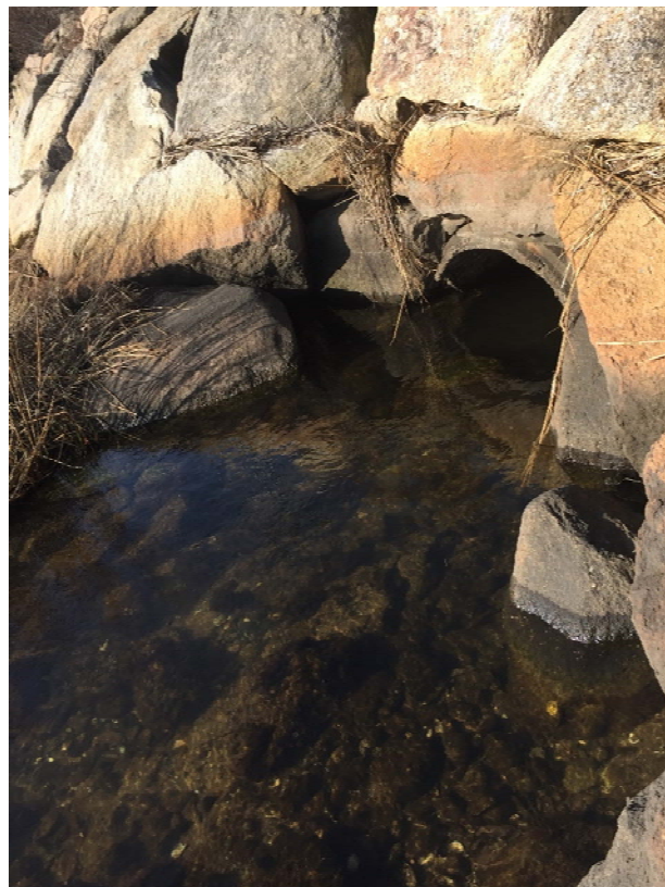
View of culvert at Sta 15+57.00 +/- (Southerly Side)
