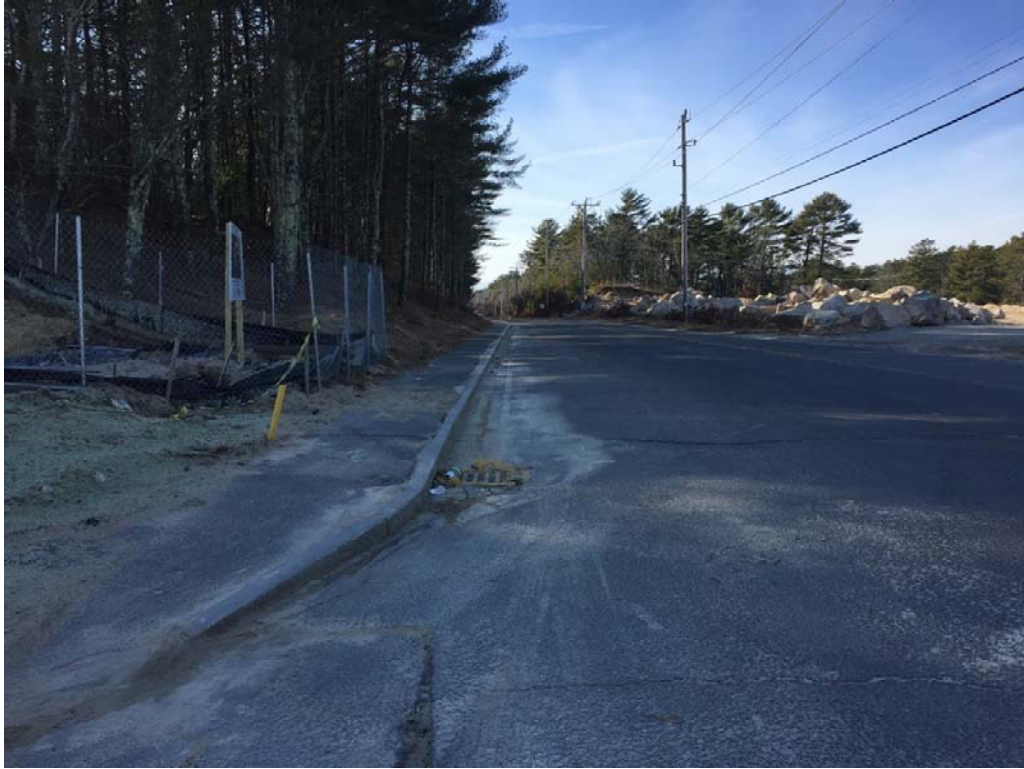
View of Minot Ave looking Westbound at STA point 61+00 +/-
