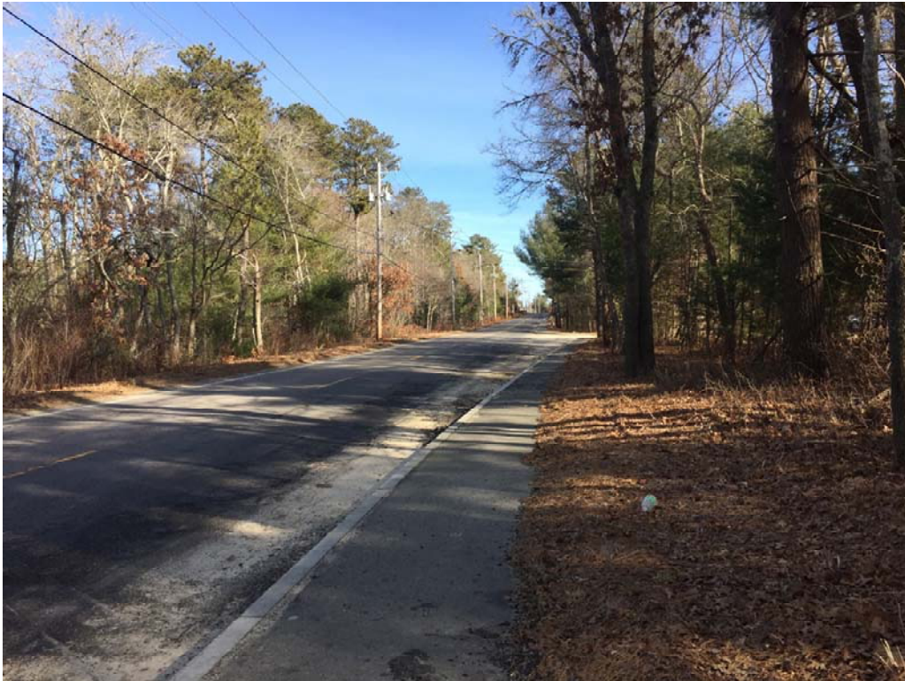
View of Minot Ave looking Eastbound at STA point 45+00 +/-
