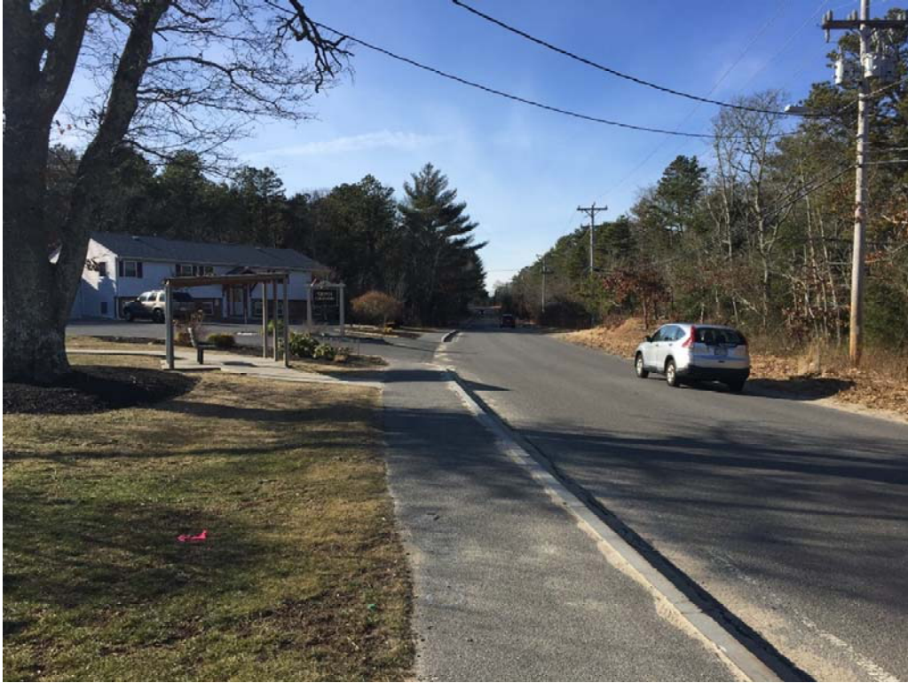
View of Minot Ave looking Westbound at STA point 88+00 +/-
