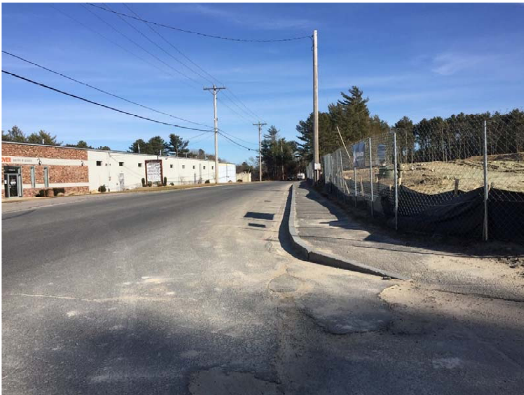
View of Minot Ave looking Eastbound at STA point 61+00 +/-
