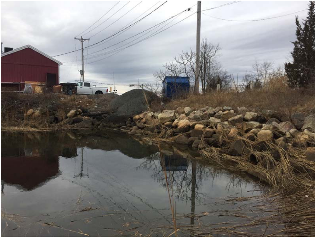
View of existing rip-rap by Sta 0+00.00 (Southerly Side)
