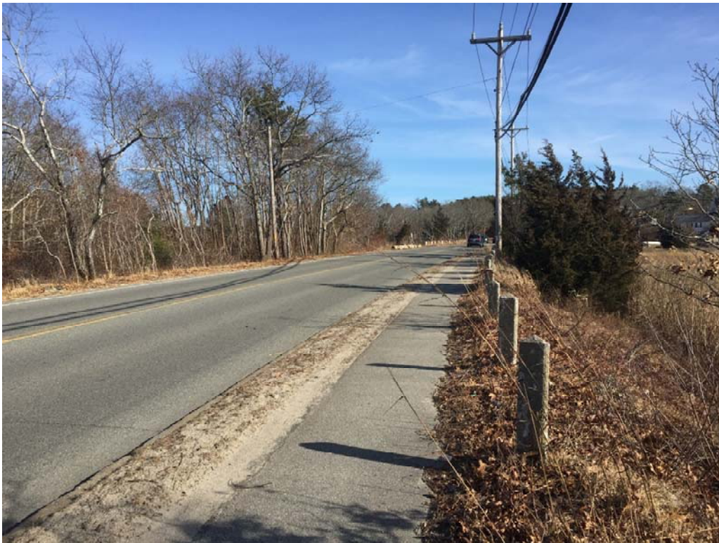
View of Narrows Rd looking Eastbound at STA point 12+00 +/-
