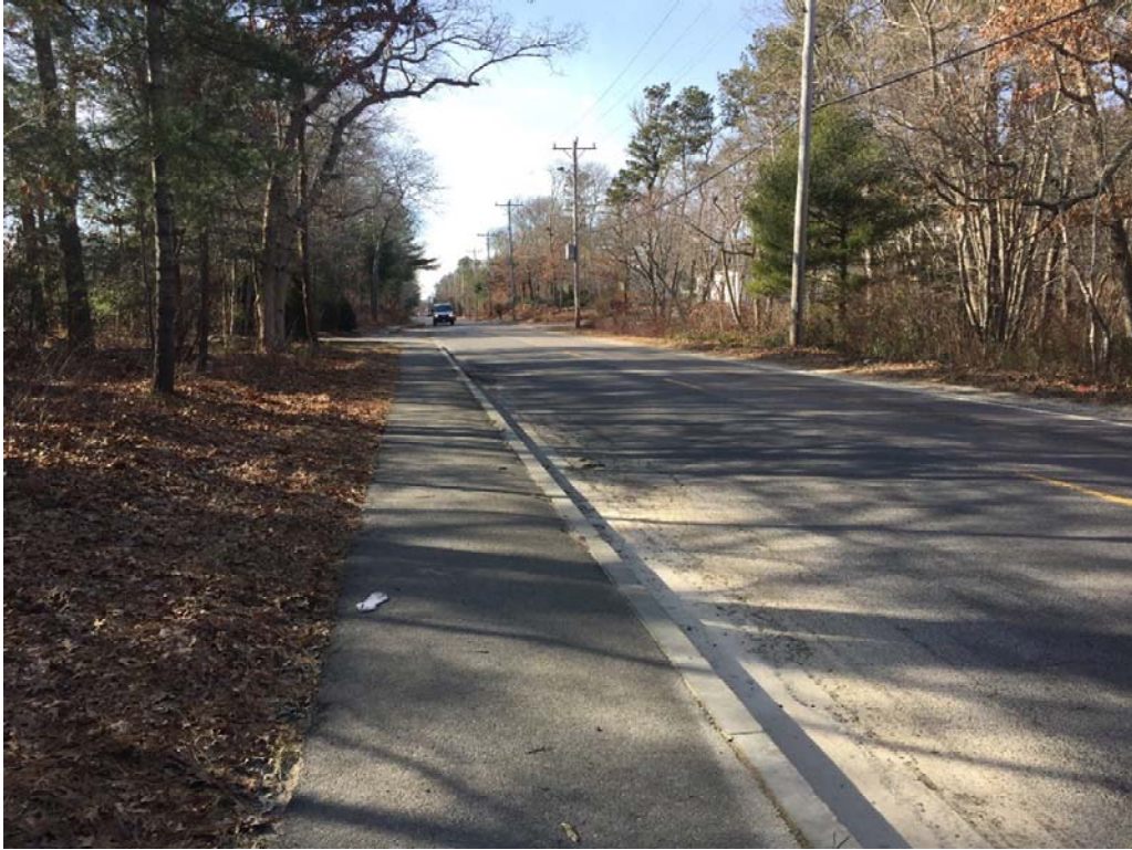
View of Minot Ave looking Westbound at STA point 45+00 +/-
