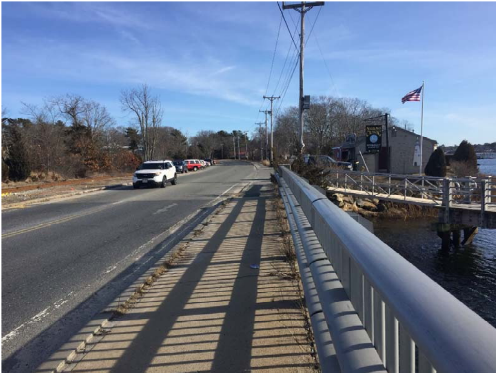
View of intersection at Narrows Rd and Sandwich Rd looking Eastbound
