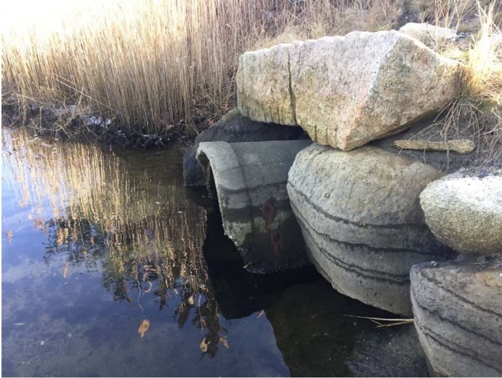
View of culvert at Sta 15+57.00 +/- (Northerly Side)
