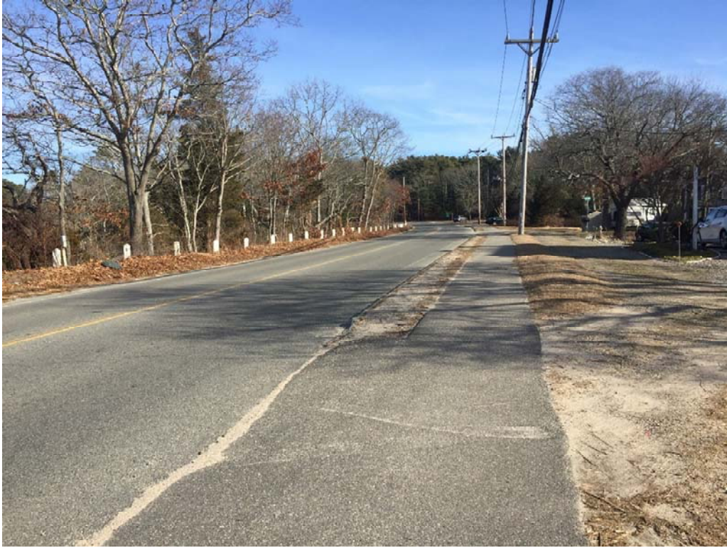
View of Narrows Rd looking Eastbound at STA point 16+00 +/-
