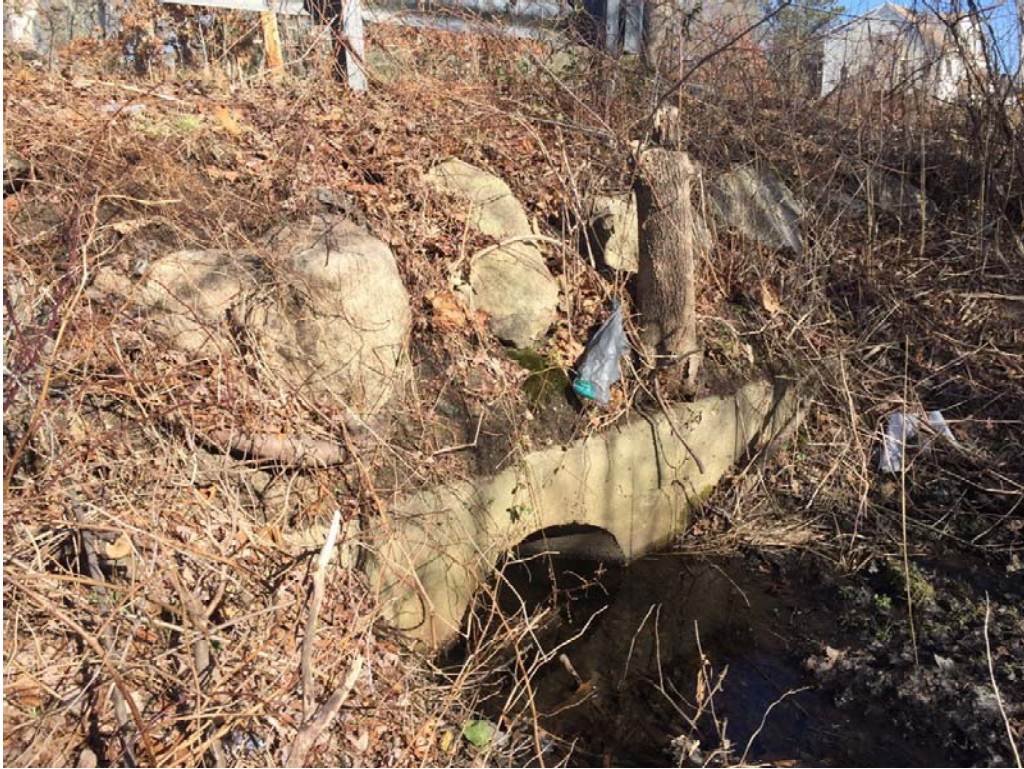
View of culvert at Sta 89+30.00 +/- (Southerly Side)
