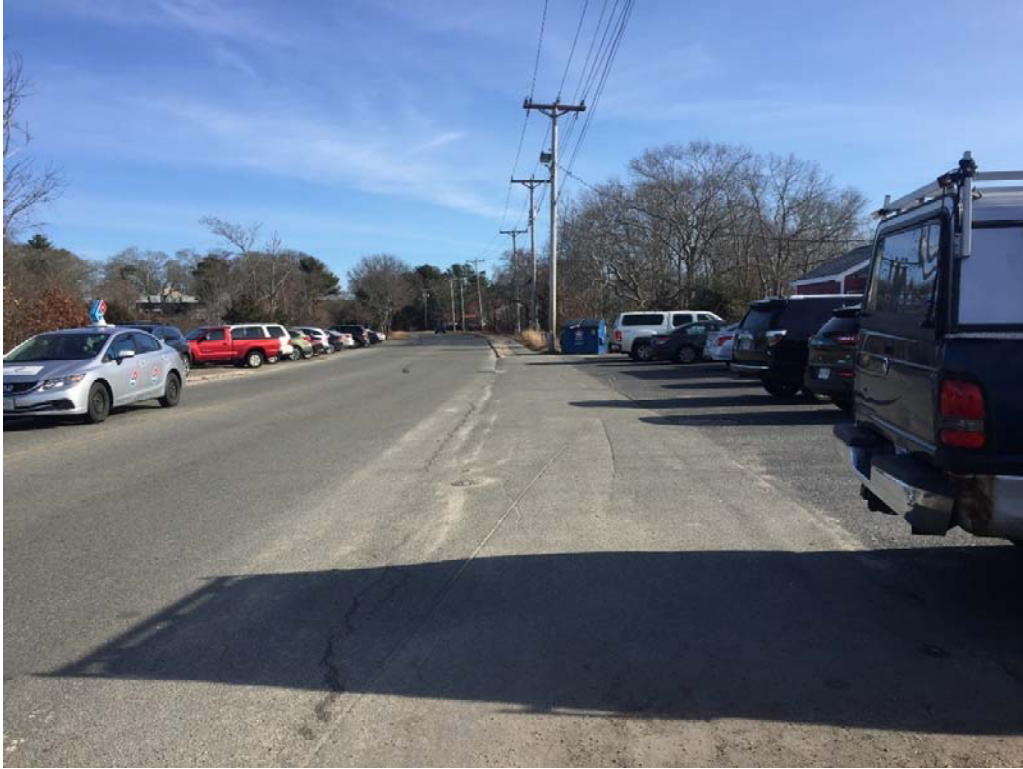
View of Narrows Rd looking Eastbound in front of Narrows Restaurant
