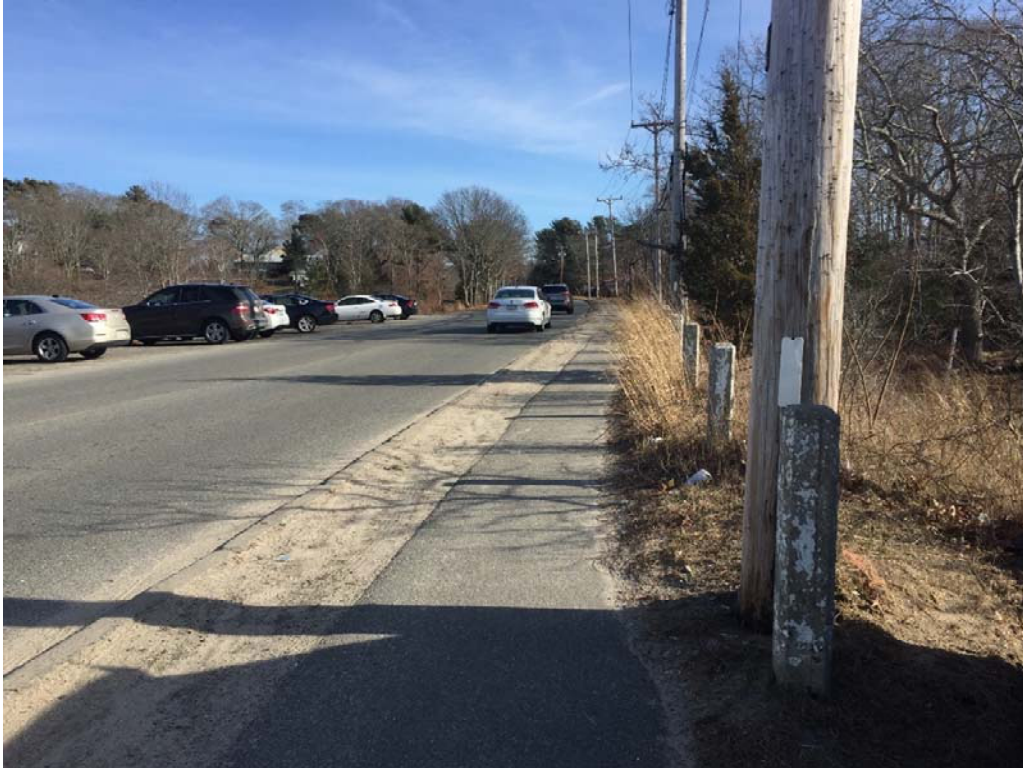
View of Narrows Rd looking Eastbound at STA point 0+00 +/-
