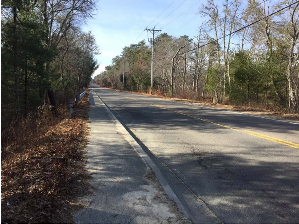
View of Minot Ave looking Westbound at STA point 53+00 +/-
