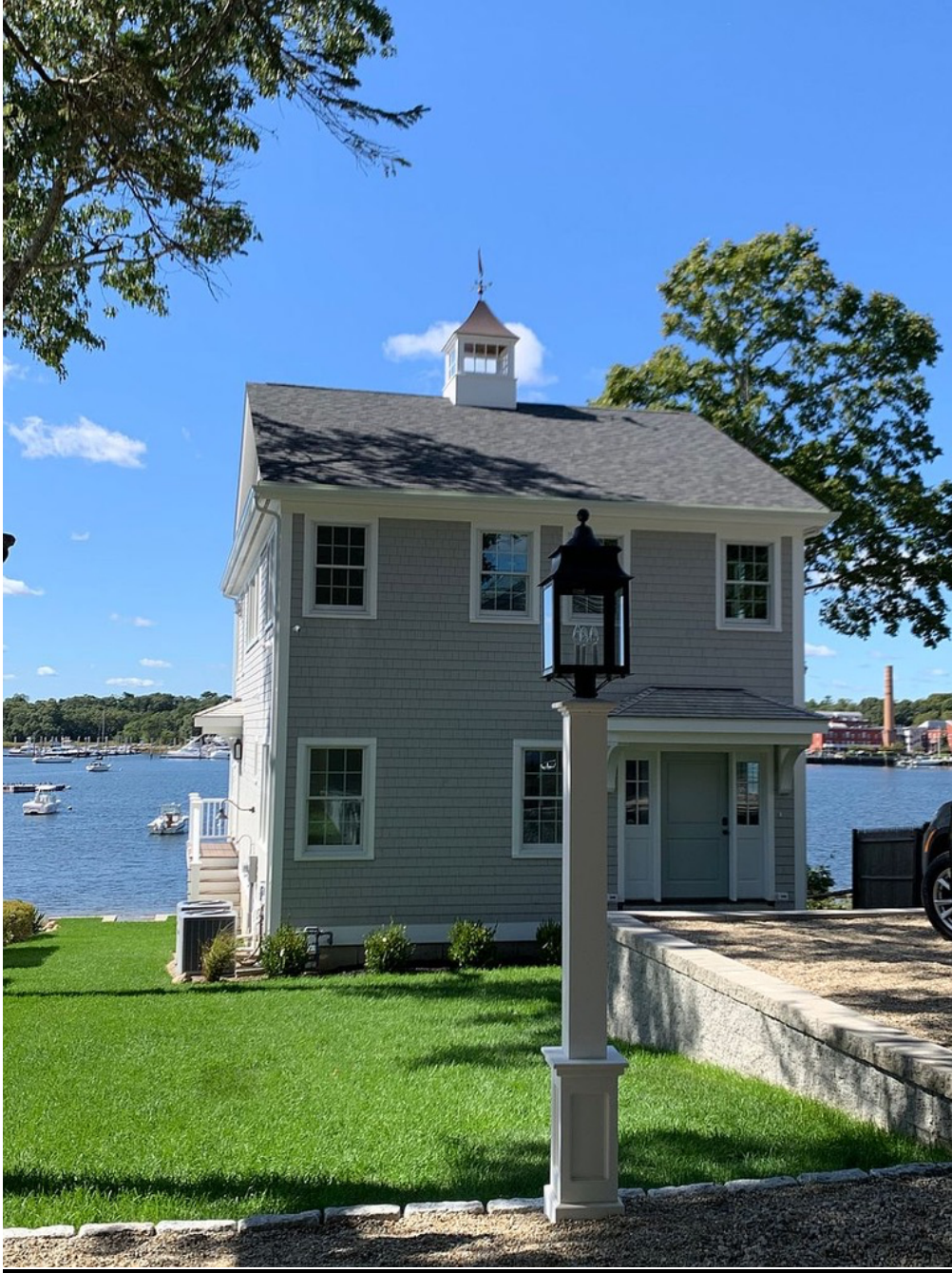
9 Oak Hill After renovation and Special Permit (front view)
