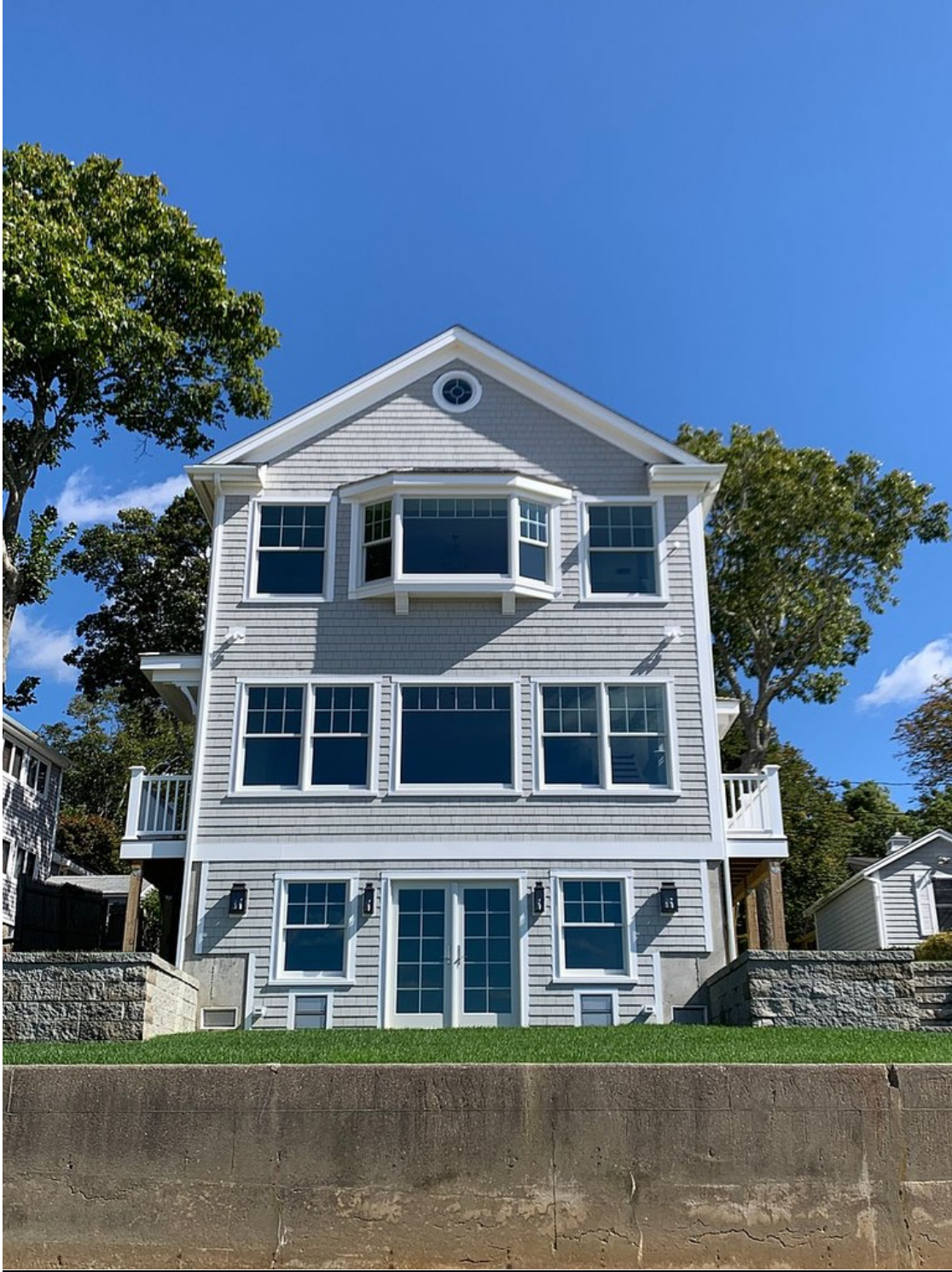
9 Oak Hill After renovation and Special Permit (back view)
