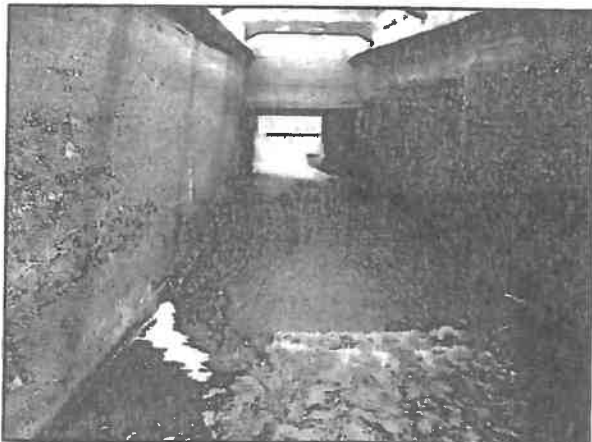
Flume before work commenced.
