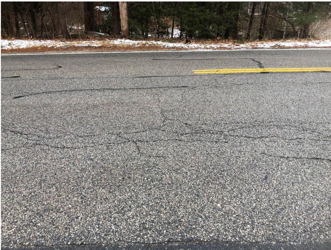
Plymouth Street Pavement View South
