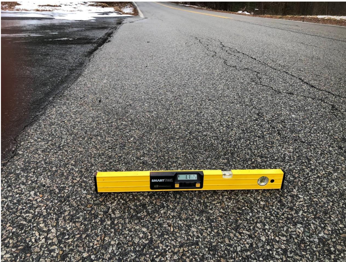
Plymouth Street Transverse Slope at Centerline View East
