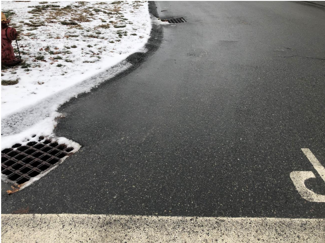
Godfrey Circle Pavement West Side View North
