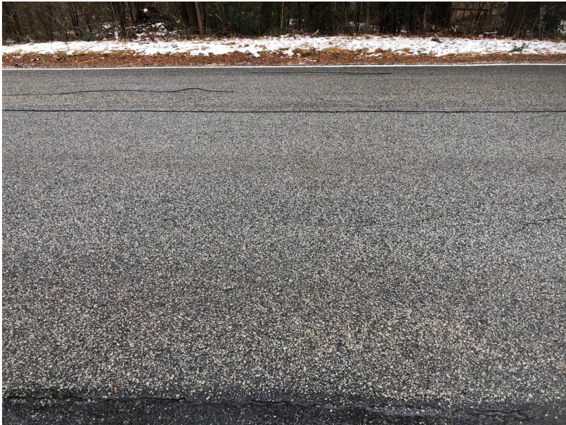
Plymouth Street Pavement View South
