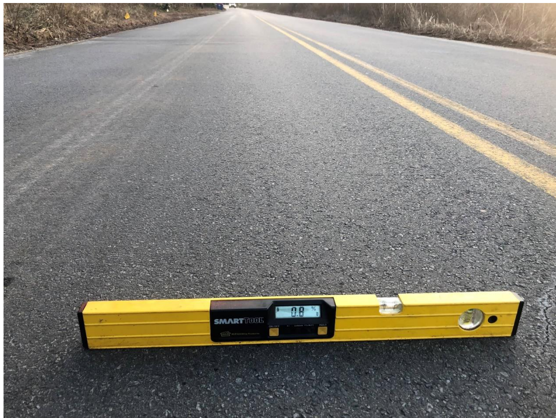
Great Neck Road Transverse Slope at Centerline View East
