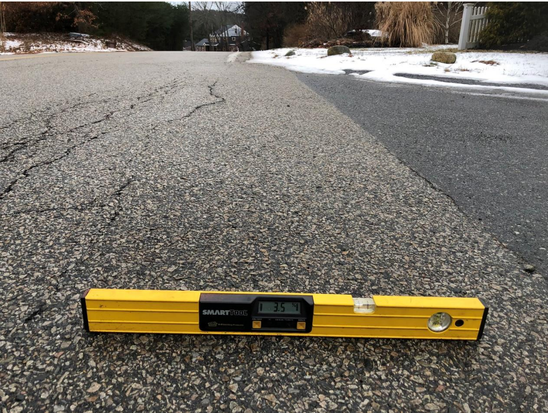
Plymouth Street Transverse Slope View West
