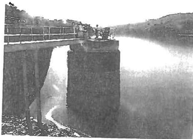
Figure 2 – Photo of Crystal Springs Adit Tower
