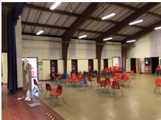
Cafetorium with curved glue-laminated timber beams.
