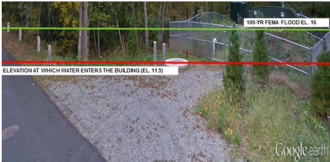
Figure 30 Cromessett Road Pump Station
