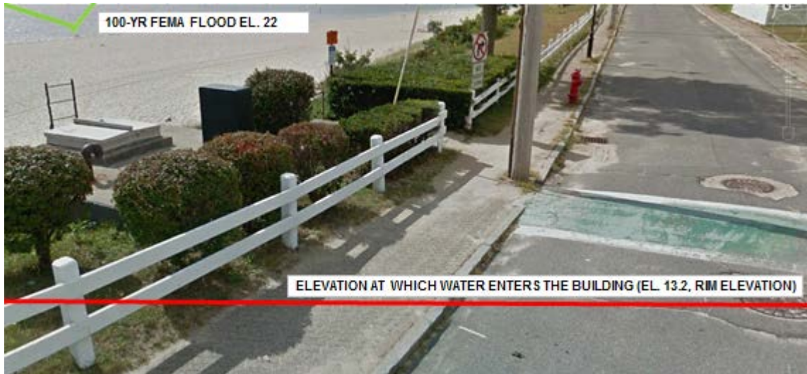
Figure 9 South Boulevard Pump Station
