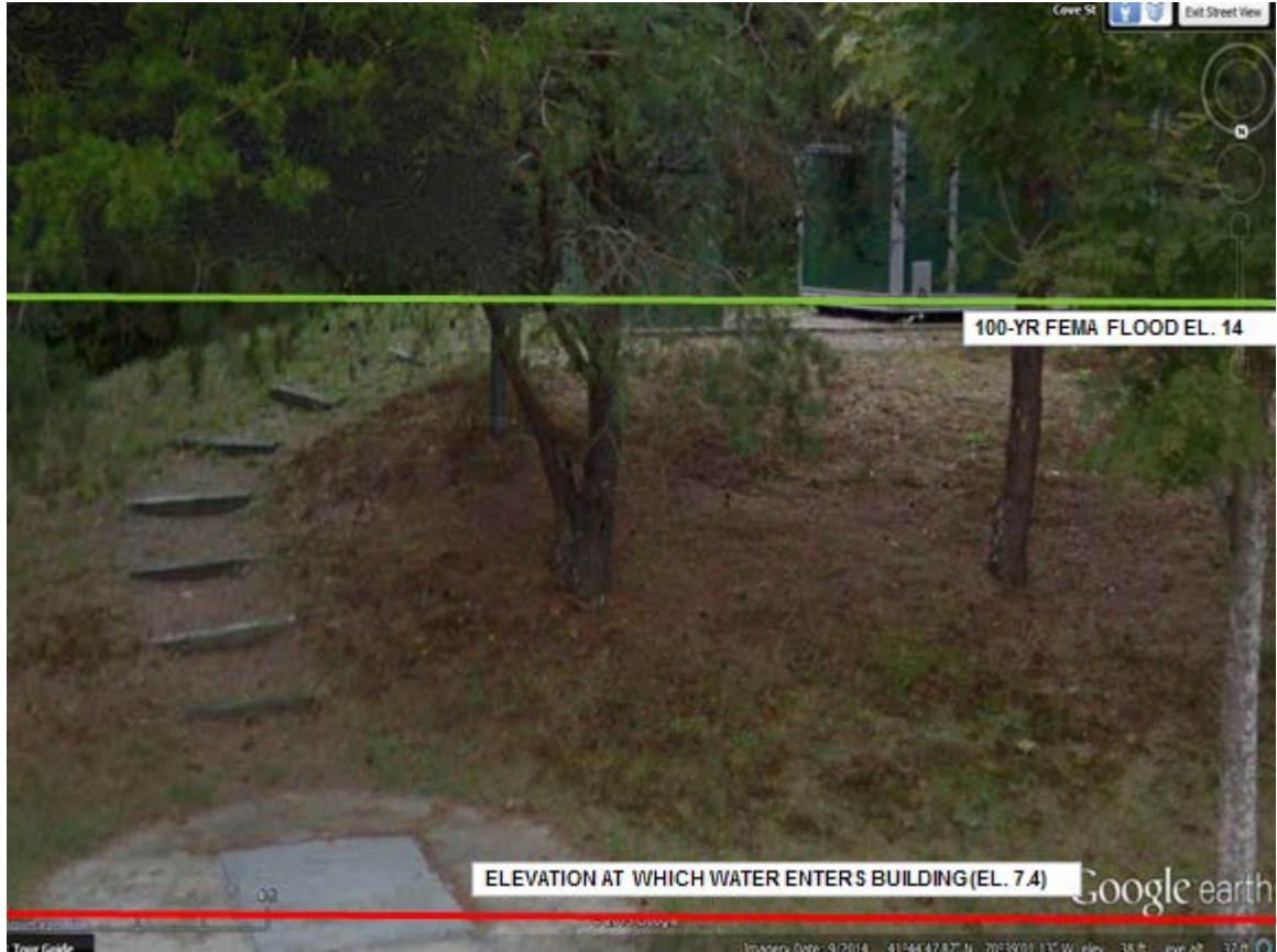
Figure 36 Onset Heights Pump Station
