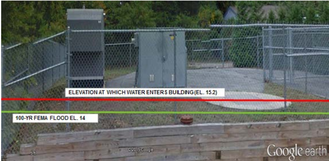
Figure 69 Hathaway Pump Station
