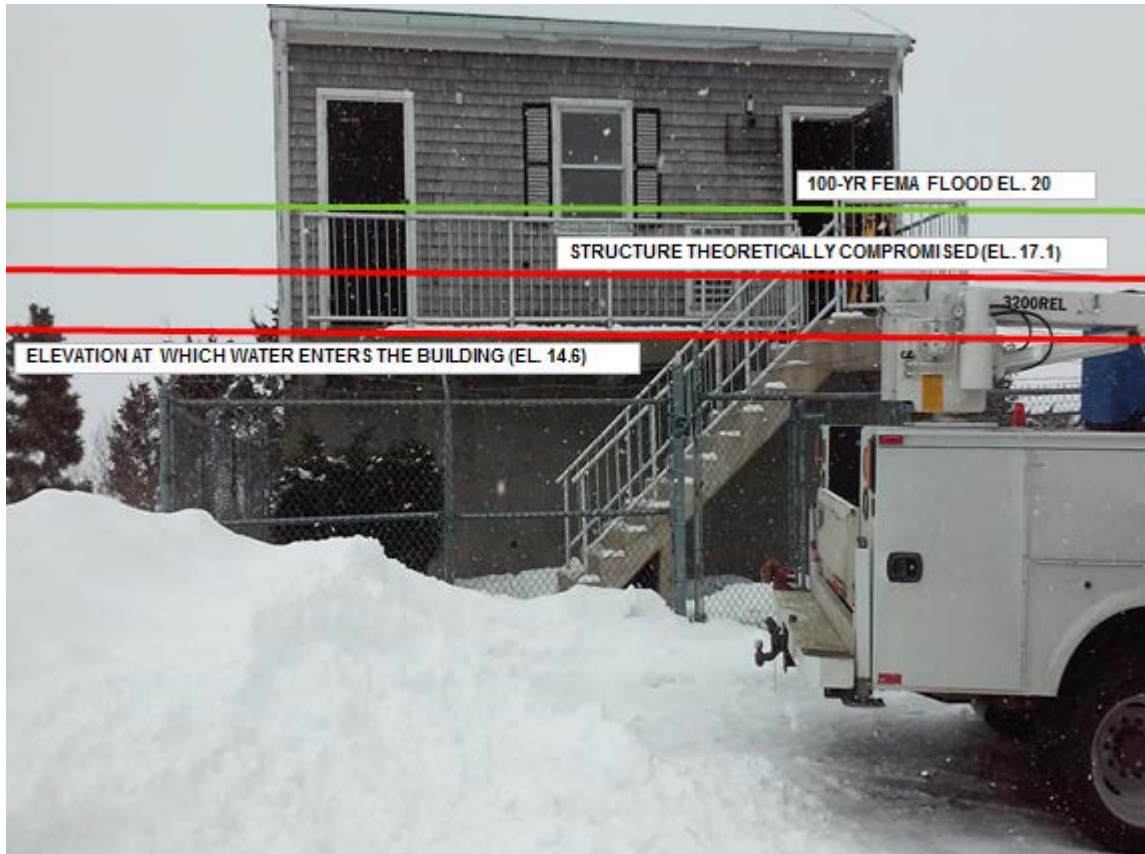
Figure 27 Ruggles Pump Station
