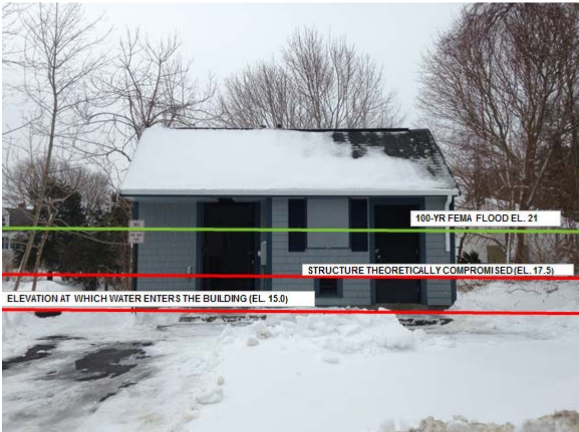
Figure 12 Hill Street Jefferson Shores Pump Station
