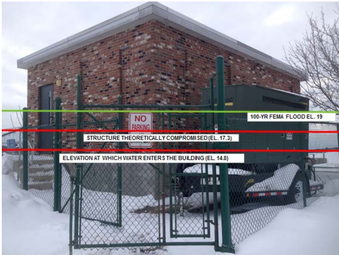
Figure 23 South Water Street Pump Station
