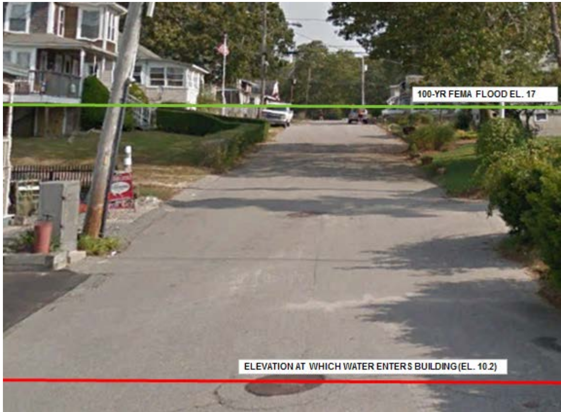
Figure 6 Bay Street Pump Station
