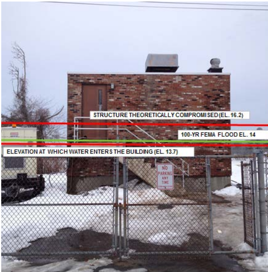
Figure 54 North Boulevard Pump Station
