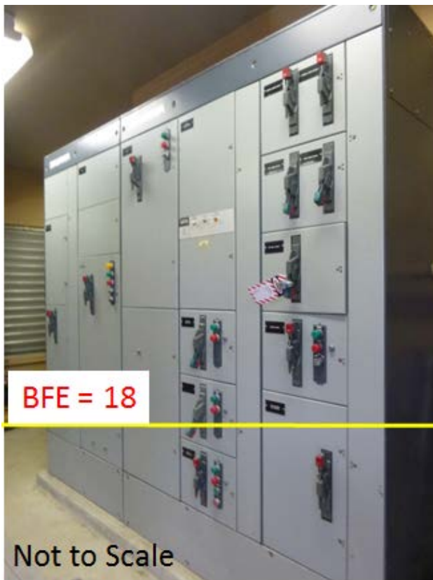
Figure 17 Smith Master Control Panel (MCC)
