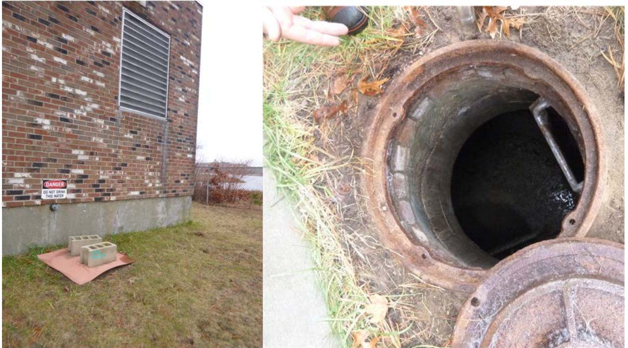
Figure 55 North Boulevard Wet Well Manhole Cover
