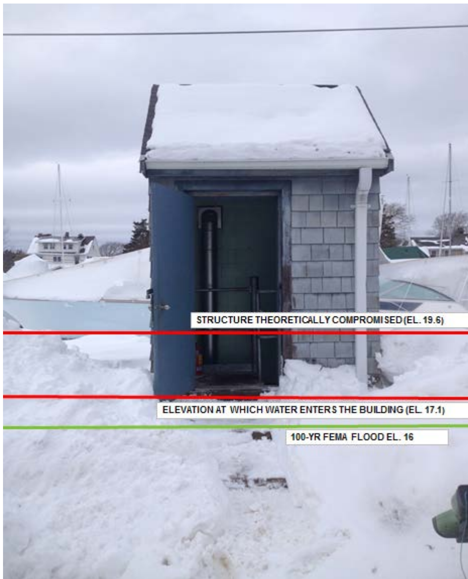
Figure 73 Green Street Pump Station
