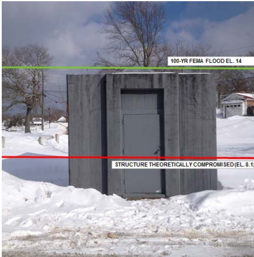
Figure 60 East Boulevard Pump Station
