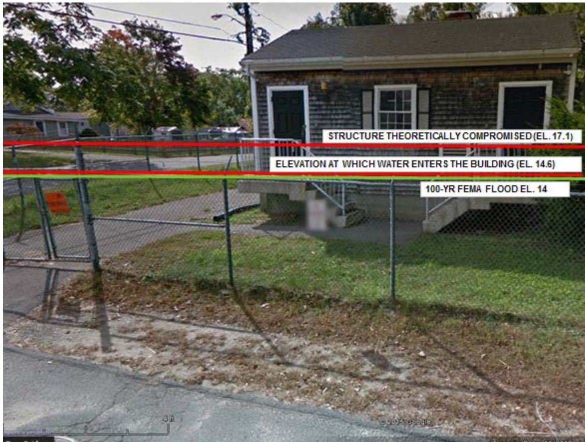
Figure 48 Pinehurst Pump Station
