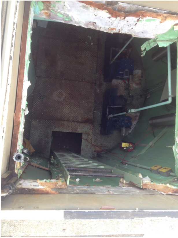
Figure 10 South Boulevard Substructure
