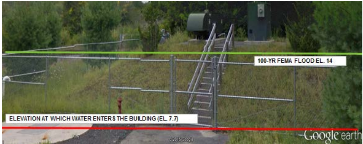
Figure 65 Indian Neck Pump Station
