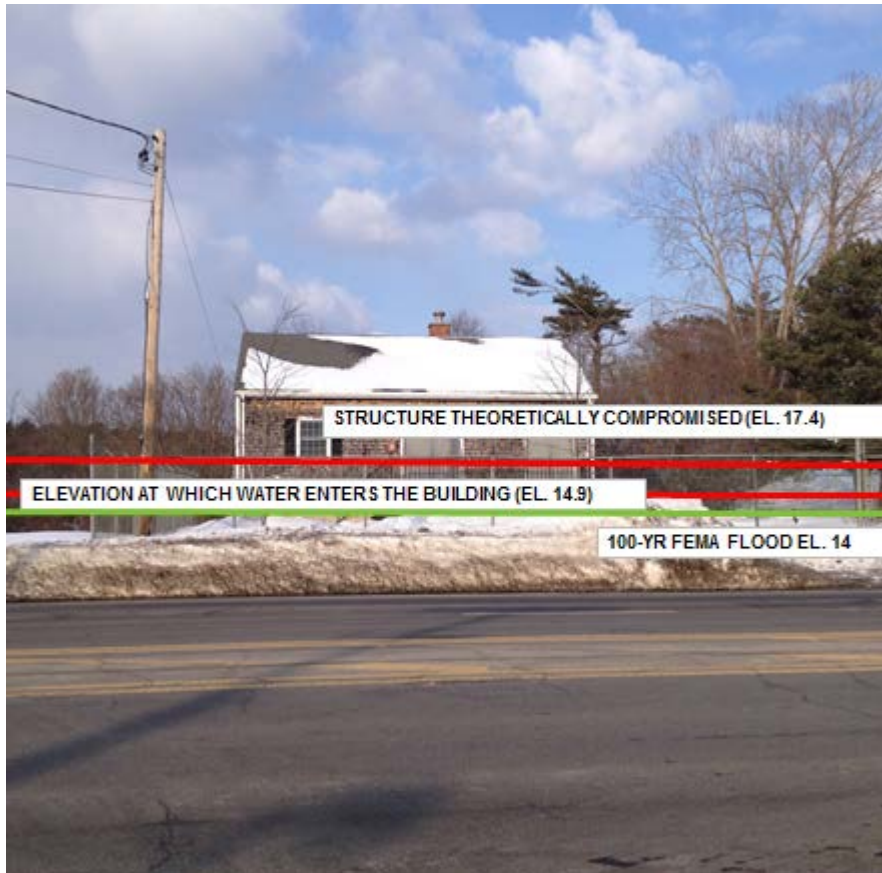
Figure 51 Dick's Pond Pump Station
