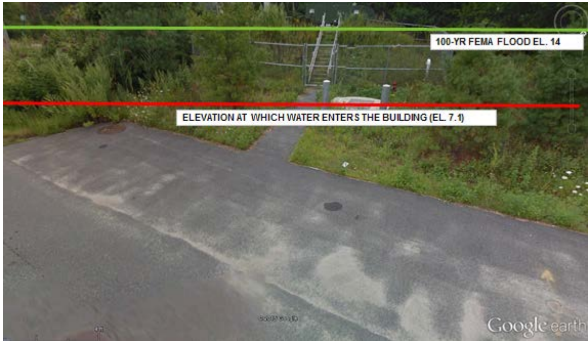
Figure 39 Avenue A Pump Station
