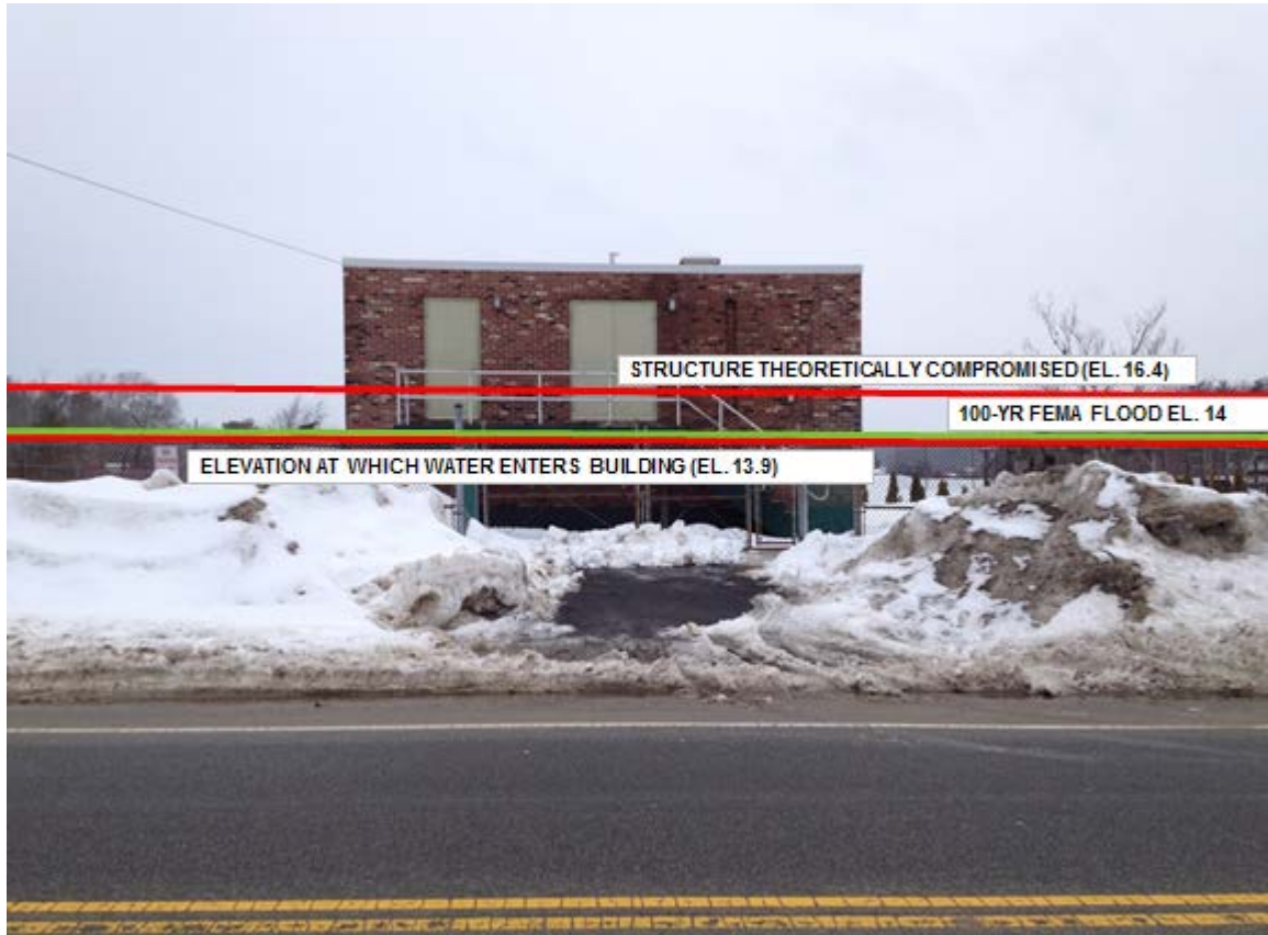
Figure 57 Hynes Field Pump Station
