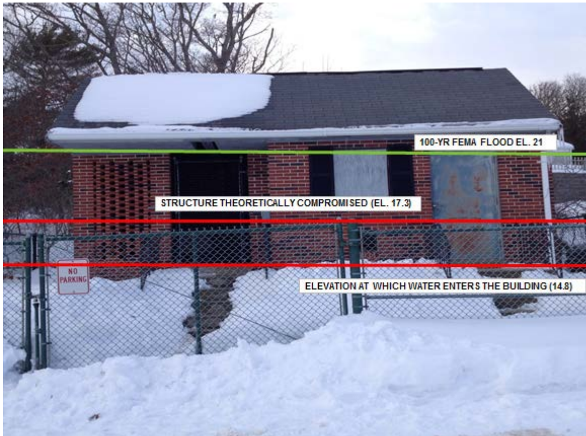
Figure 14 Saltworks Road Pump Station
