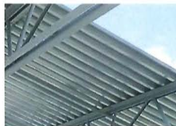
STEEL ROOF AND FLOOR DECK
