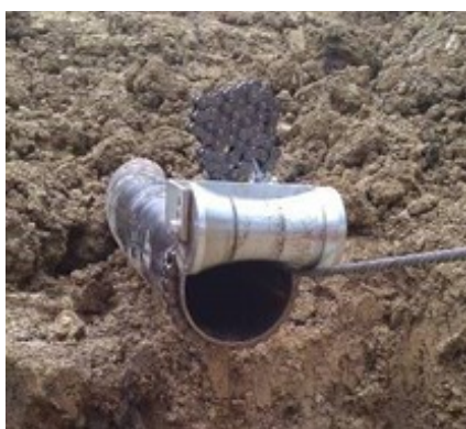
Illustration 18: Rope protection roller installed on host pipe
