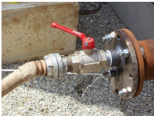
Illustration 9: Dummy flange installed to the host pipe
