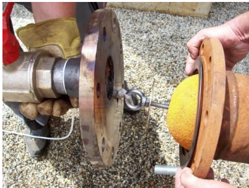
Illustration 8: Installing a pigging flange (with rope inlet, the pig in this example is made of foam)
