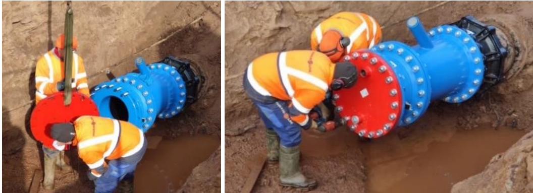
Illustration 24: Testing flange installation
