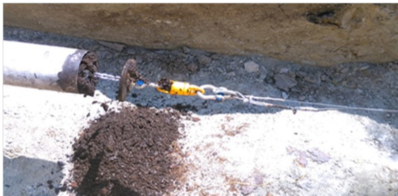
Illustration 21: Rubber discs arriving to target pit
