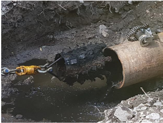
Illustration 19: Scrapers arriving to target pit
