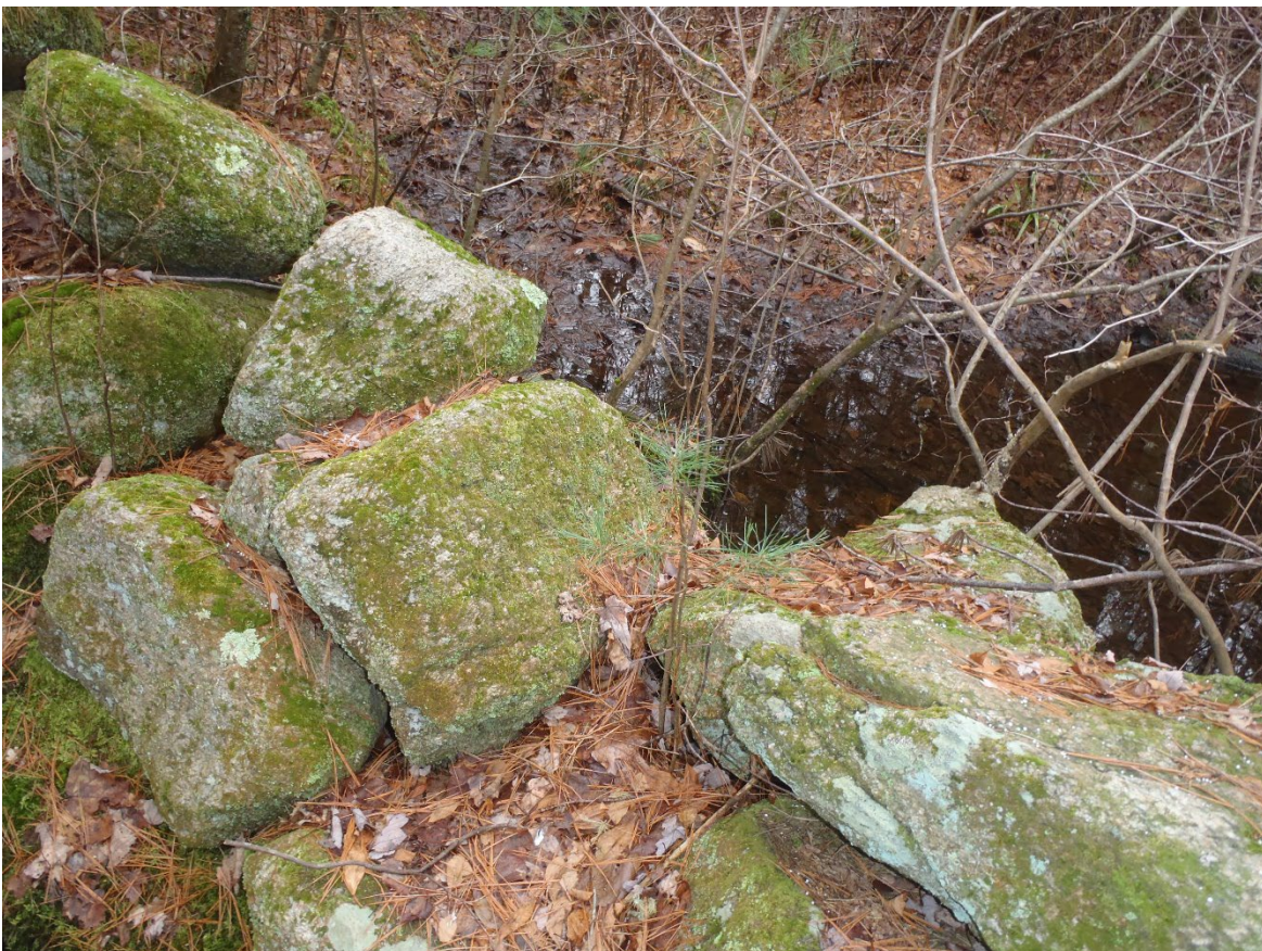
Stone wall next to standing water
