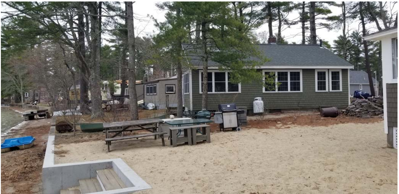
Right Side View (West Elevation)
