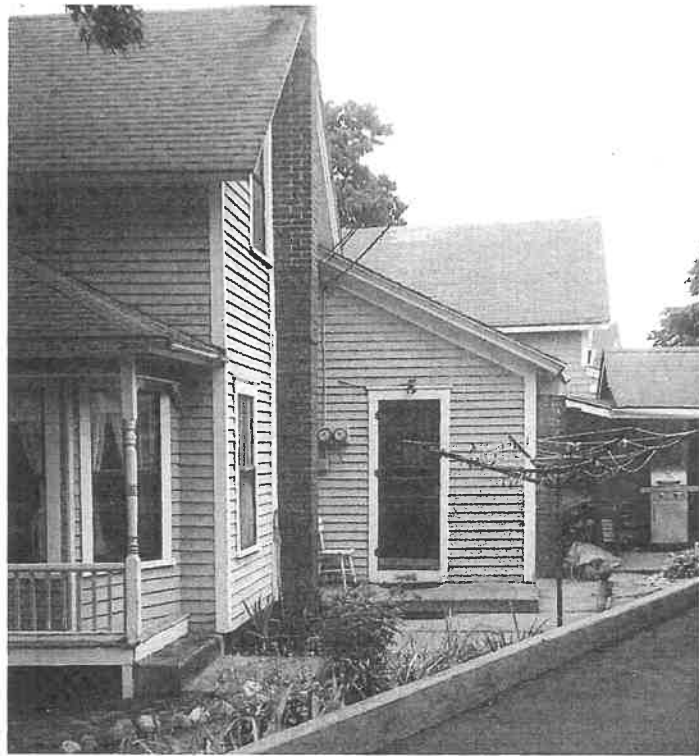
REAR VIEW @ AREA OF WORK
