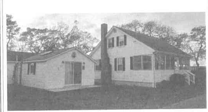
Exterior Photo of Left Side
