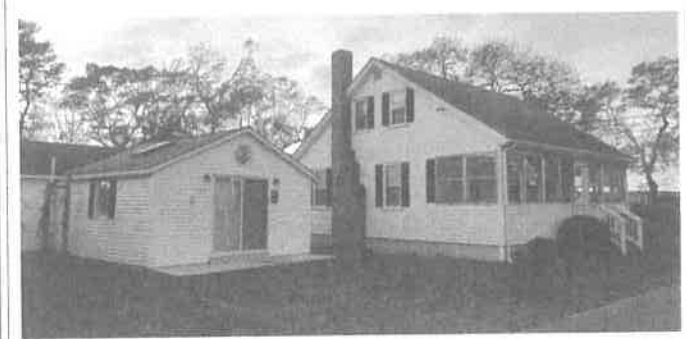
Exterior Photo of Left Side
