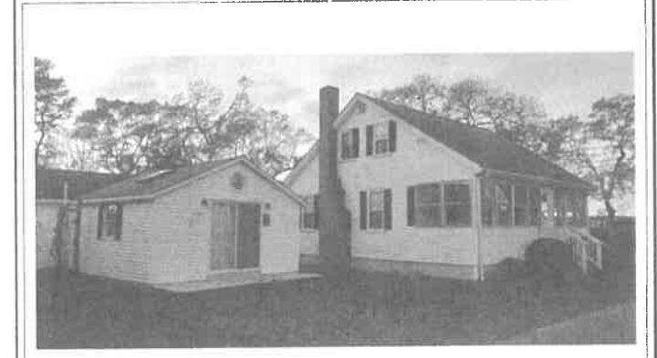
Exterior Photo of Left Side
