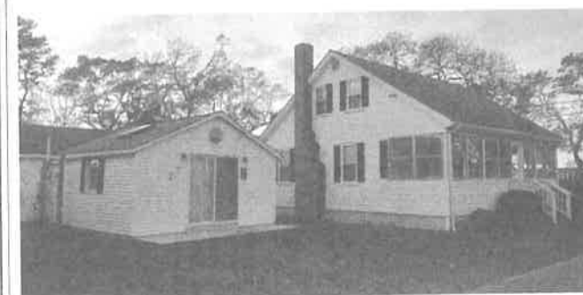
Exterior Photo of Left Side
