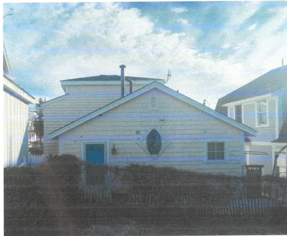
EXISTING VIEW FROM NORTH @ AREA OF ADDITION
