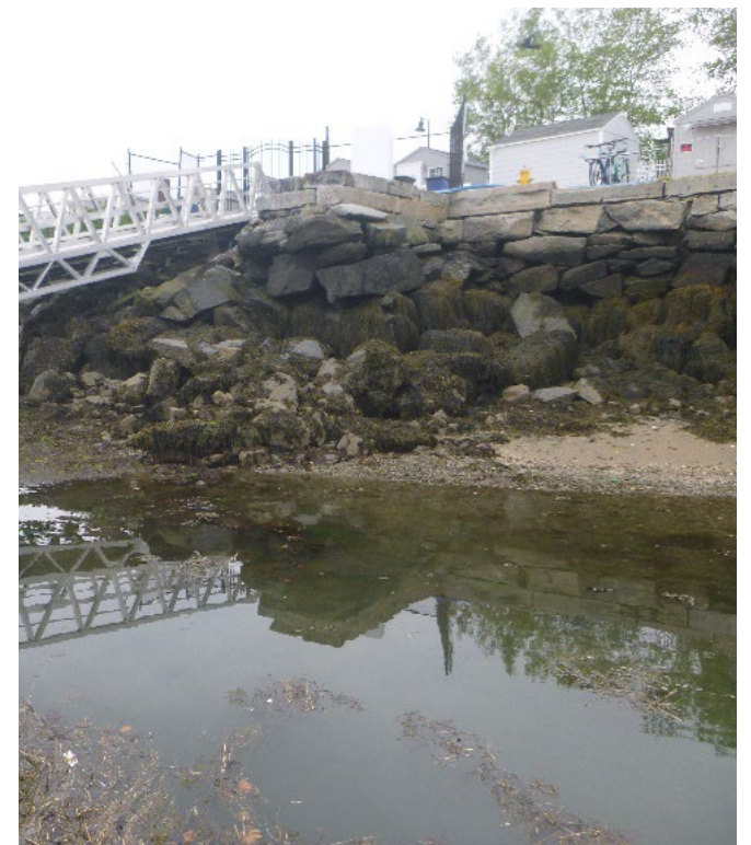
Seawall Rehabilitation, Portland, ME.
