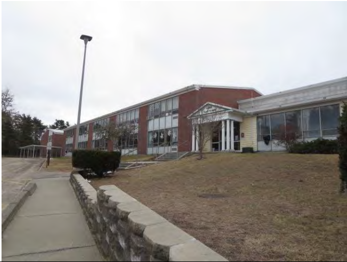
Photo #1: North side of Site building.
