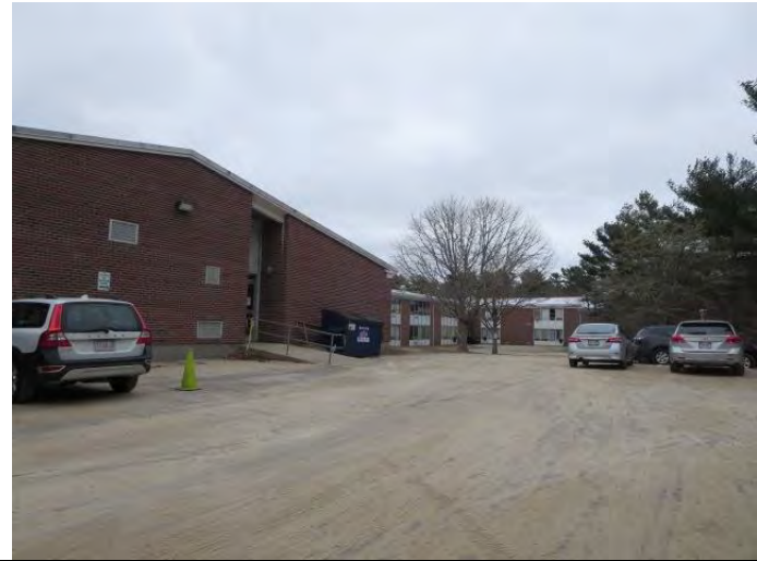
Photo #6: South side of Site building.
