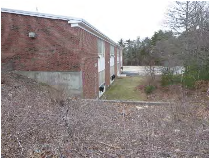
Photo #3: East side of the Site building.
