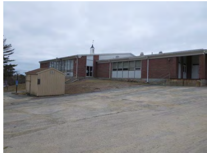
Photo #4: West side of Site building.
