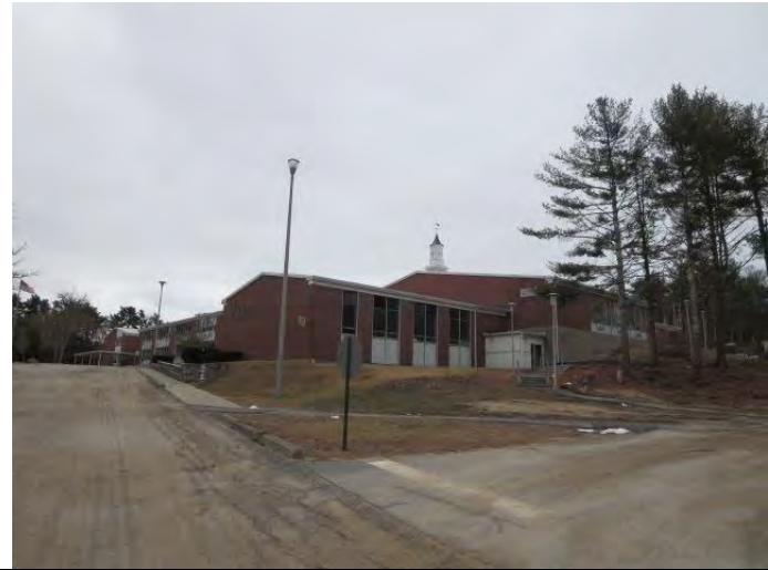
Photo #2: North and west sides of the Site building.
