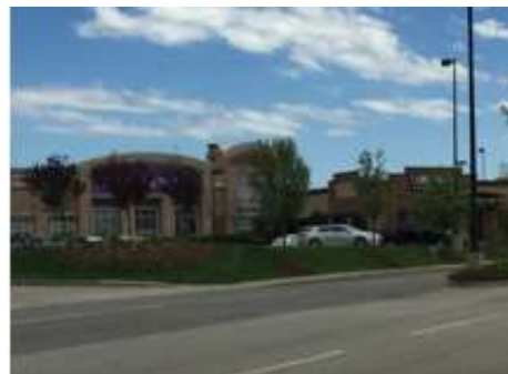
Commercial Strips and Centers
