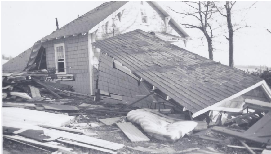
Figure 3-14. Wind-damaged home during Hurricane Edna (1954).
