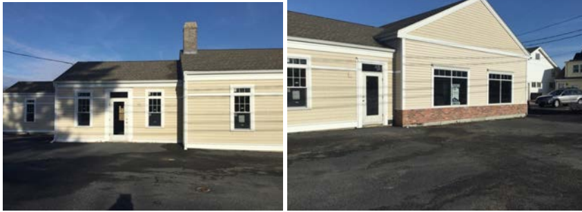
Main building - vacant
