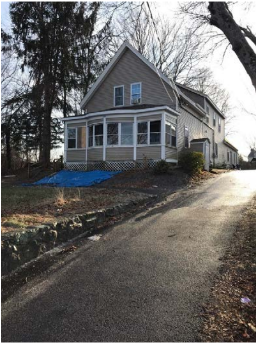
Views of building from Main Street; boarded-up windows on front porch and deteriorating siding in places. Tarp covering front garden area.
