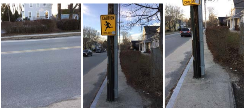
View of sidewalk encroachment.
