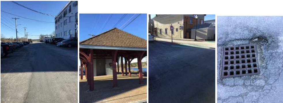
Looking northerly along right of way near train station. Drainage structures are in middle of pavement and width of roadway varies significantly along this stretch.
