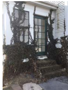
Side and rear façade details – damaged and rotting trim and gutters, vines growing on and inside building
