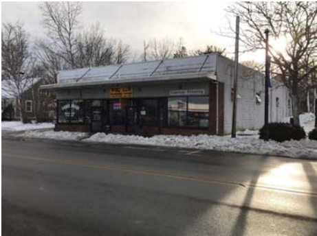
Front façade of building, top half deteriorating
