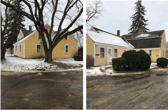
Side and rear of structure
