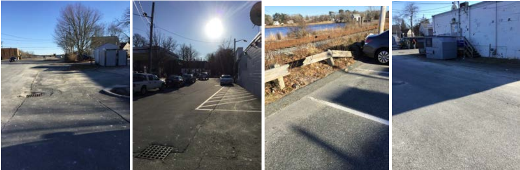
Wooden guardrail sections are broken or missing here cars can easily come in contact with them.
