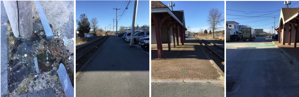
Looking northerly along right of way near train station. Drainage structures are in middle of pavement and width of roadway varies significantly along this stretch.
