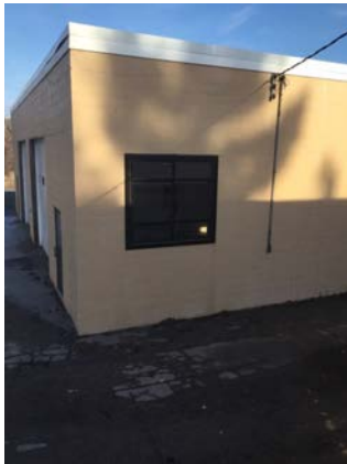
Garage attached to main building; in good condition
