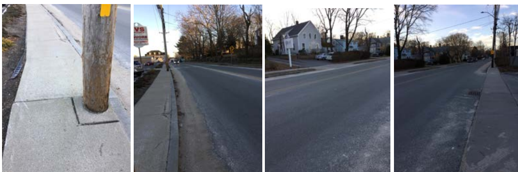
Pole locations and neighboring hedge row, render sidewalk nearly impassable.
