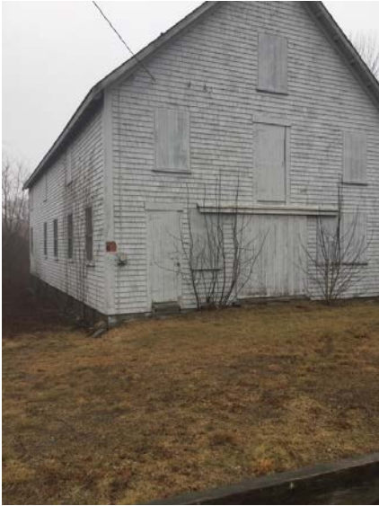
Main part of the building; boarded windows and badly deteriorating siding
