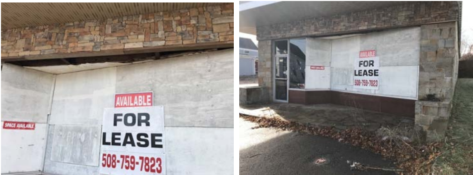
Boarded up windows on front façade with For Lease signs
