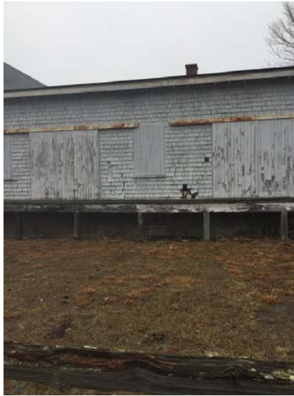
Main part of the building; boarded windows and badly deteriorating siding
