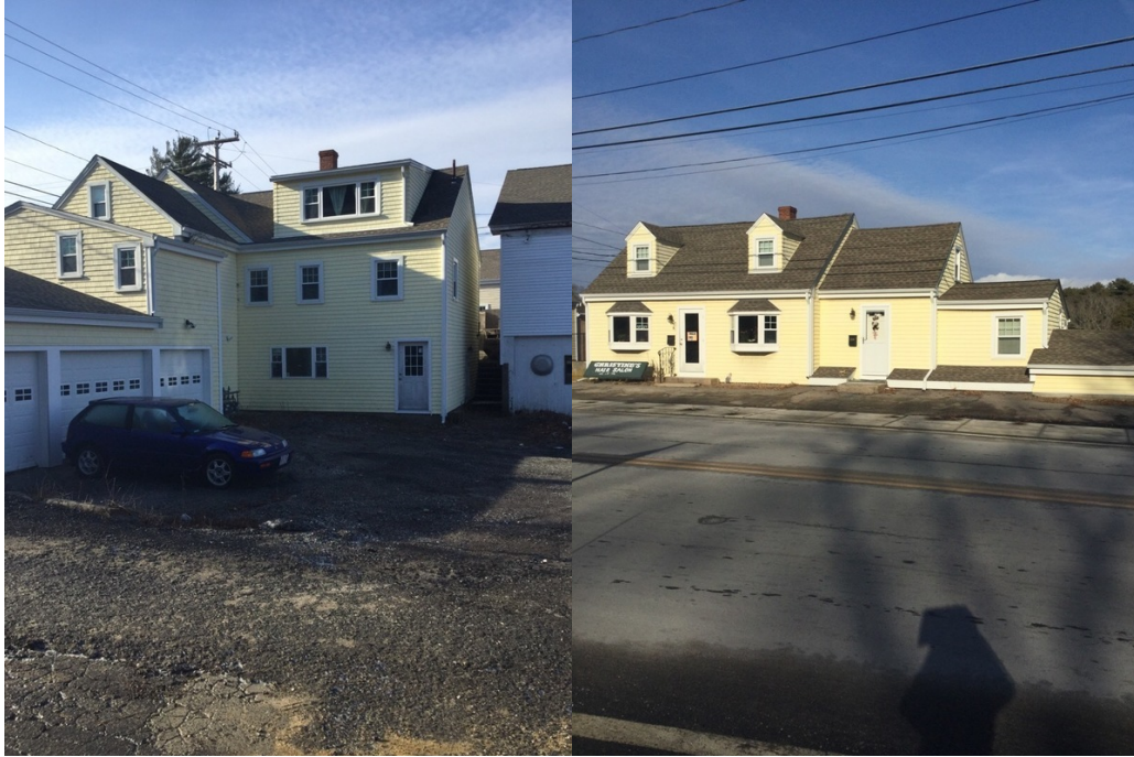
Front building: Christine's Hair Salon. Front façade facing Main Street and garage and parking area.
