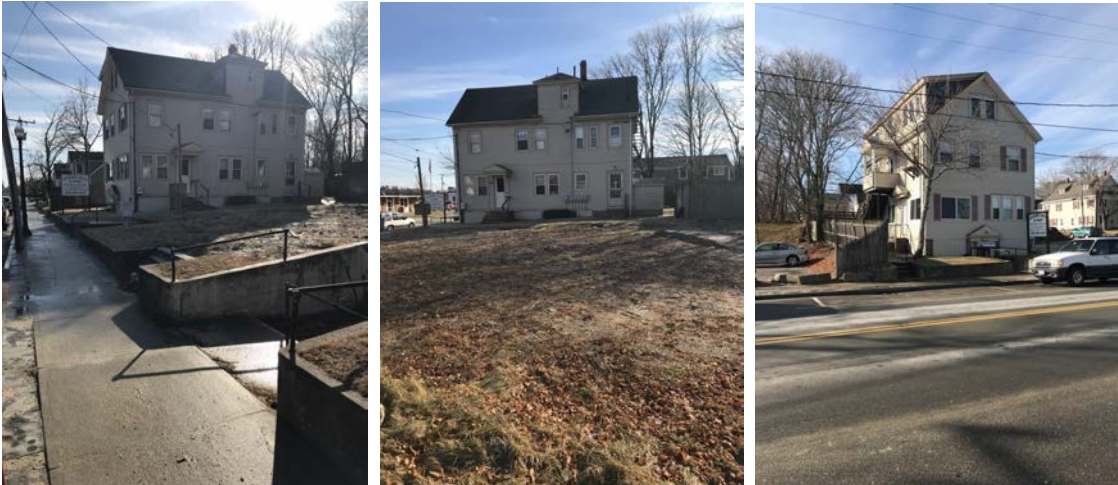
Exterior of building; windows and doors mixed in condition
