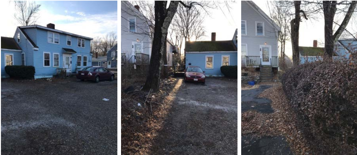
Sides of structure and driveway; moss growing in on roofs
