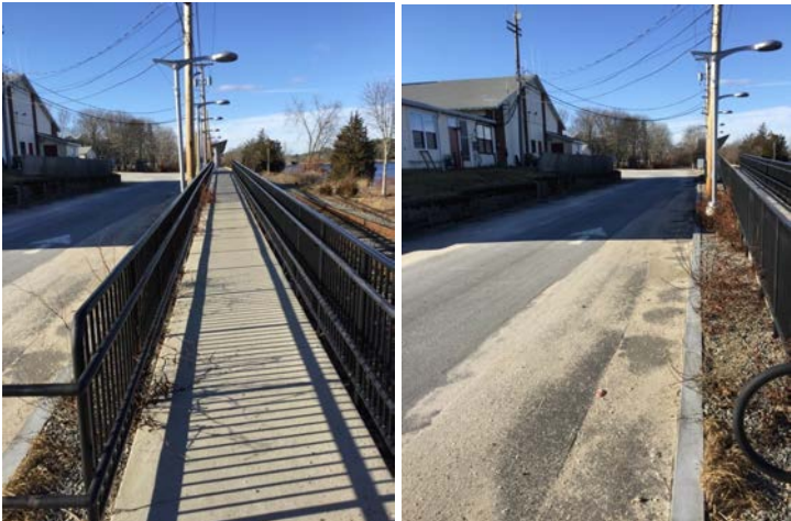
Looking northerly along “Merchant’s Way.” This area is dark, lacks sidewalks on westerly side and needs attention.
