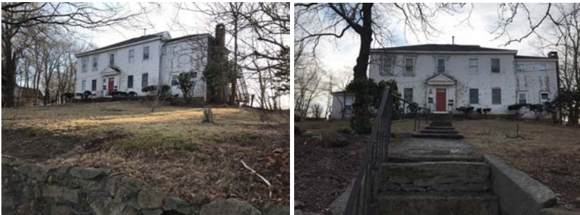
Front façade, yard, and entry stairs
