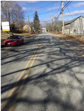
Looking northerly toward limit of area of Main Street where only one sidewalk exists.
