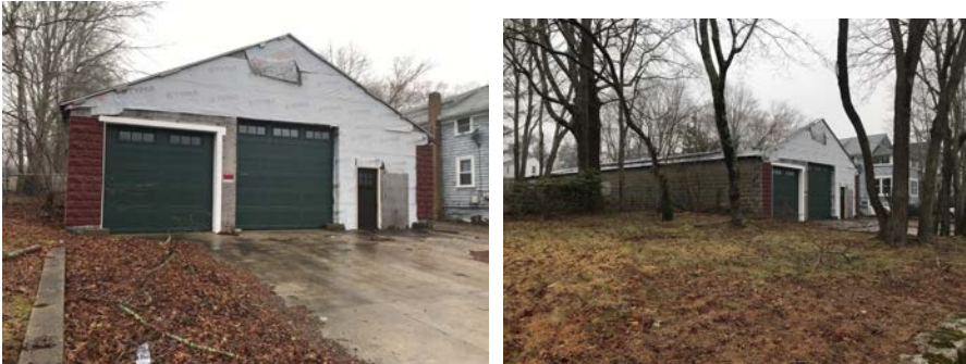
Unclear if building unfinished or abandoned due to present appearance
