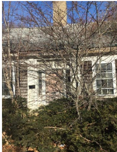
Front exterior of structure; blocked by fallen tree and overgrown brush
