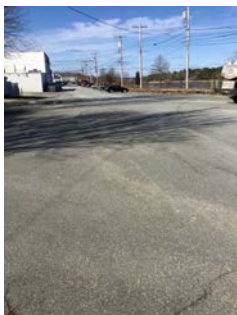
Looking northerly along rear Main Street. This area has potential but currently lacks pedestrian controls, landscaping, lighting and other much needed improvements.
