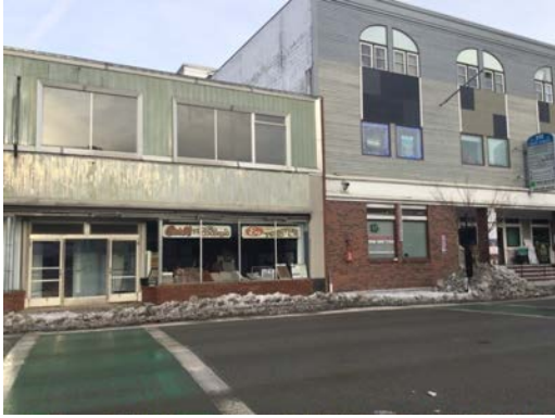
Front façade of building
