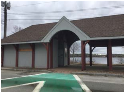
Street facing façade of train station
