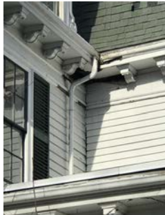
Side and rear façade details – damaged and rotting trim and gutters, vines growing on and inside building
