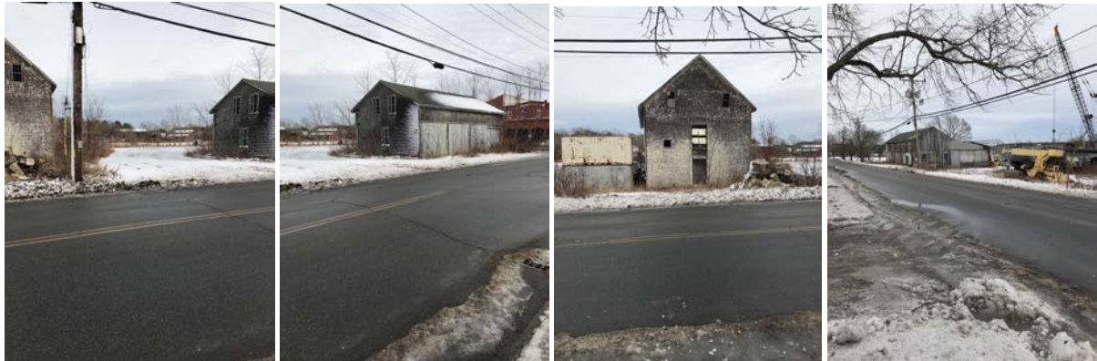
Buildings dilapidated with broken windows
