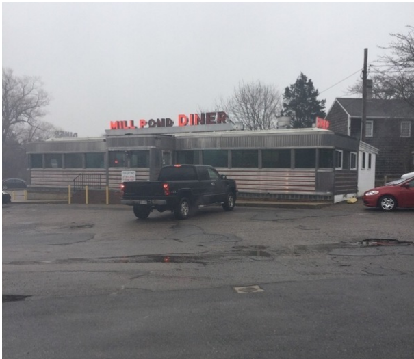
Front of building and parking lot, in poor condition
