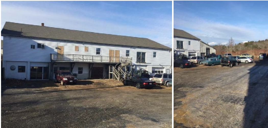
Rear building; residential use with some signage for an auto body shop. Some boarded up doors, partially vacant.
