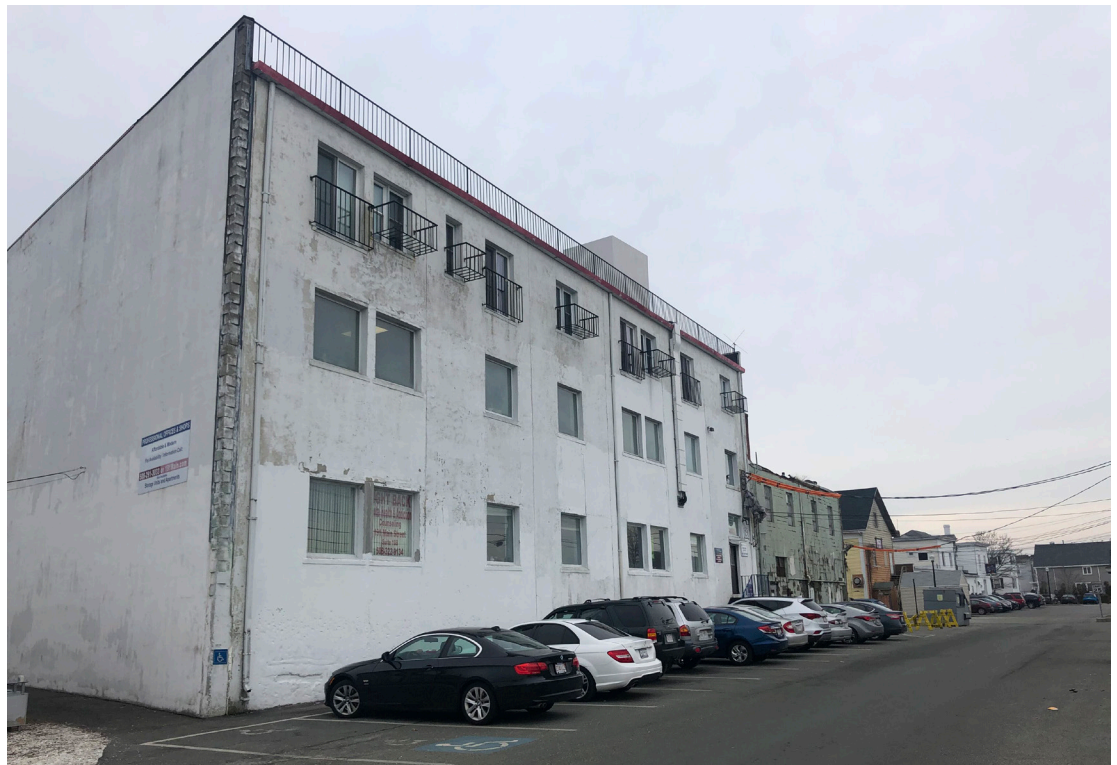
Rear of 191 Main St.
