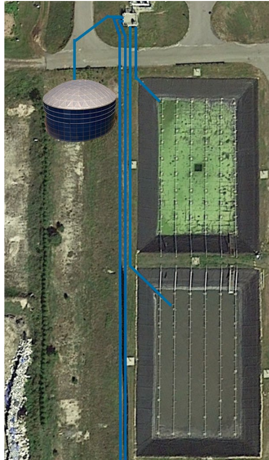
Aquastore Tank (150,000 gal)
