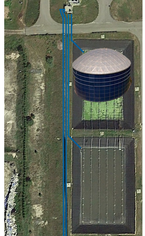
Aquastore Tank (1,200,000 gal)
