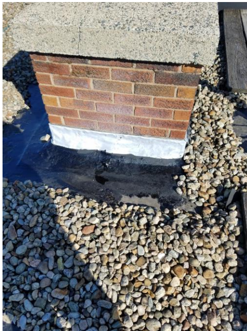
Figure 6 Sludge Dewatering Building
