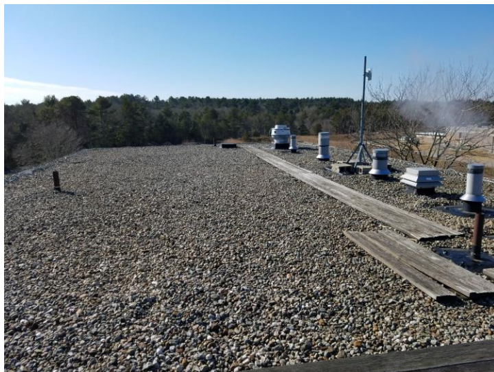
Figure 2 Sludge Dewatering Building
