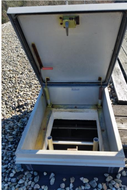
Figure 5 Sludge Dewatering Building
