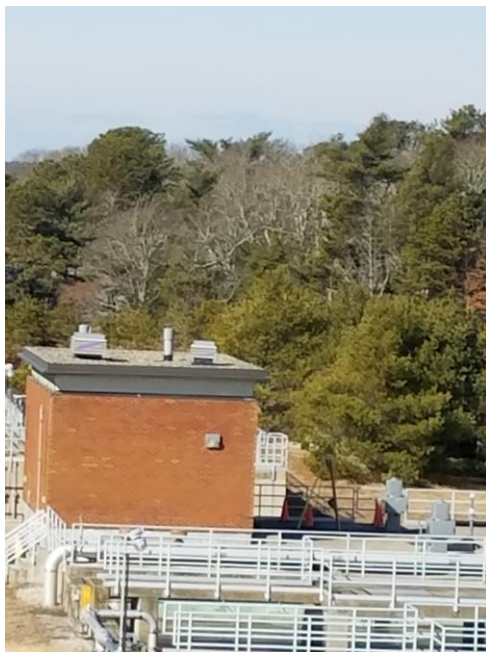
Figure 10 Septage Blower Building - West
