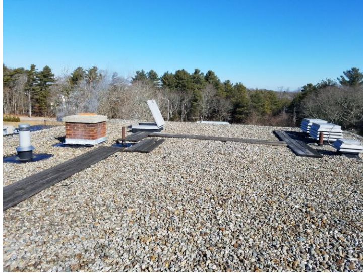
Figure 1 Sludge Dewatering Building
