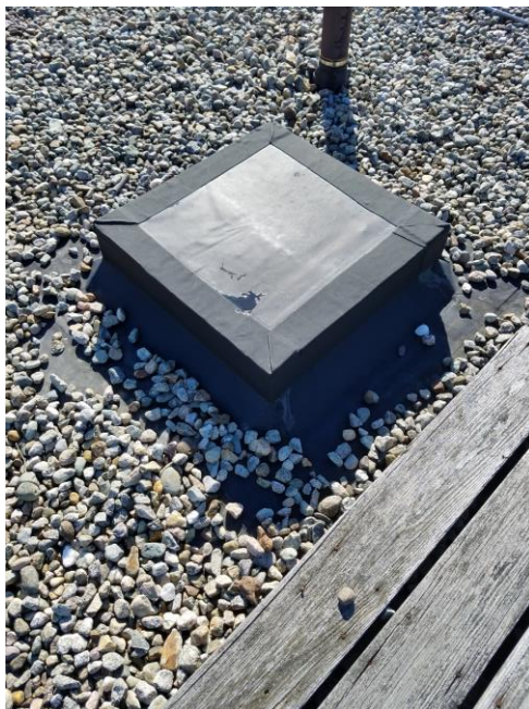
Figure 4 Sludge Dewatering Building
