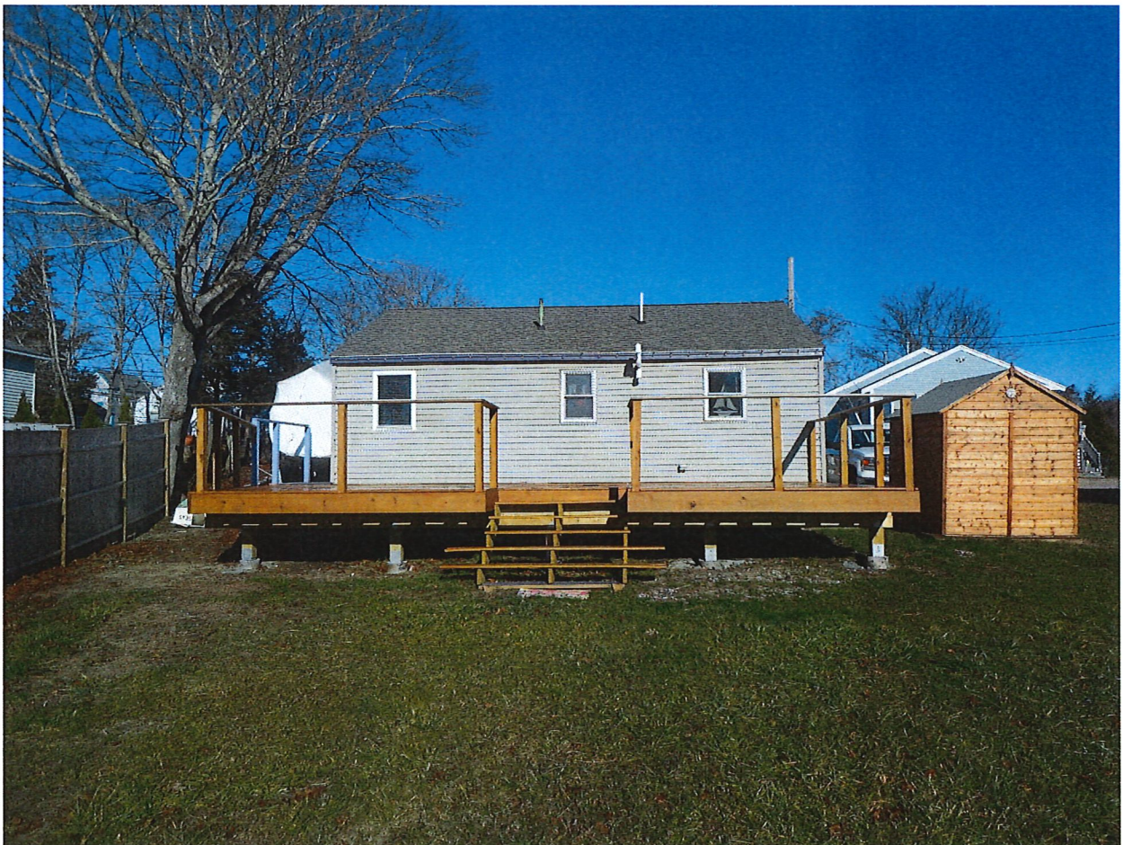
REAR VIEW OF NEWLY CONSTRUCTED WOOD DECK
